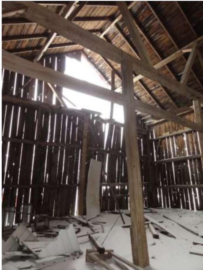
*Image 9: View of barn interior illustrating damaged exterior bent and cladding, east face (2019-02-14).*
