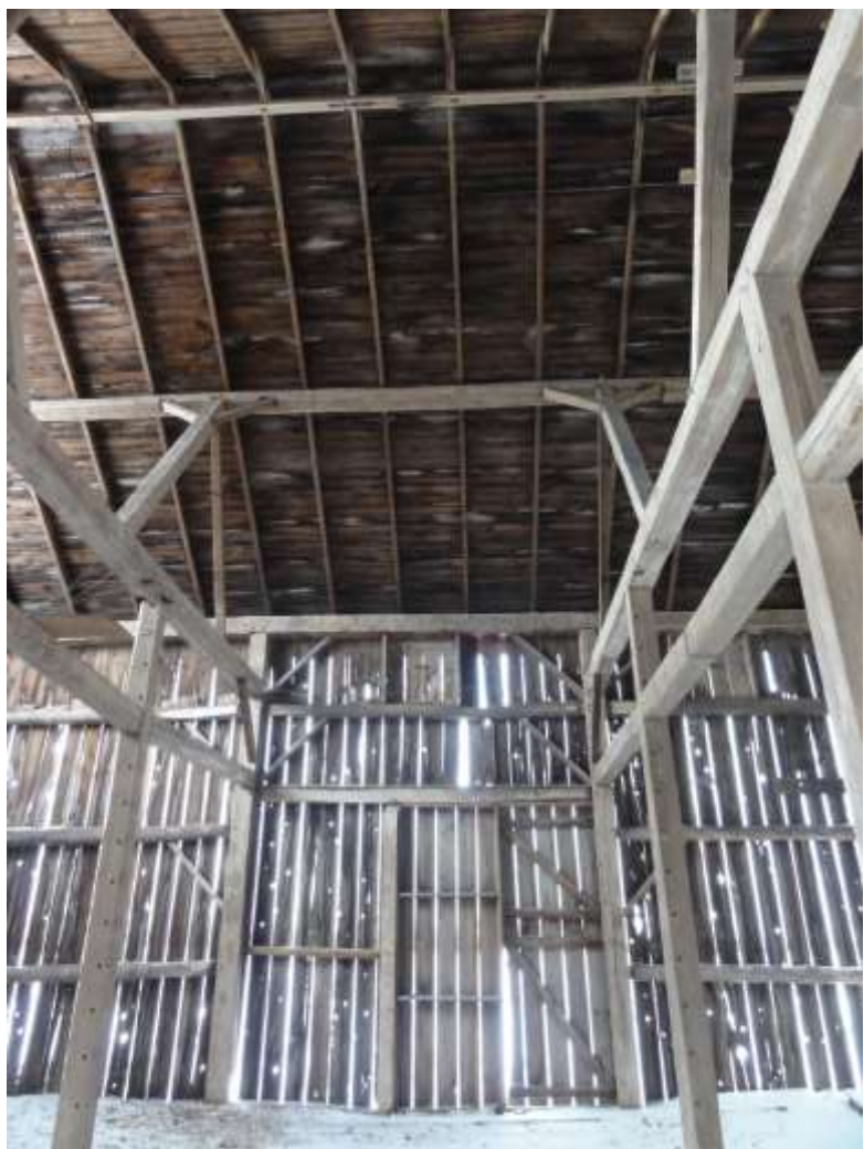
Image 5: View of barn interior illustrating structure, middle bay and timber framed bents (2019-02-14).
