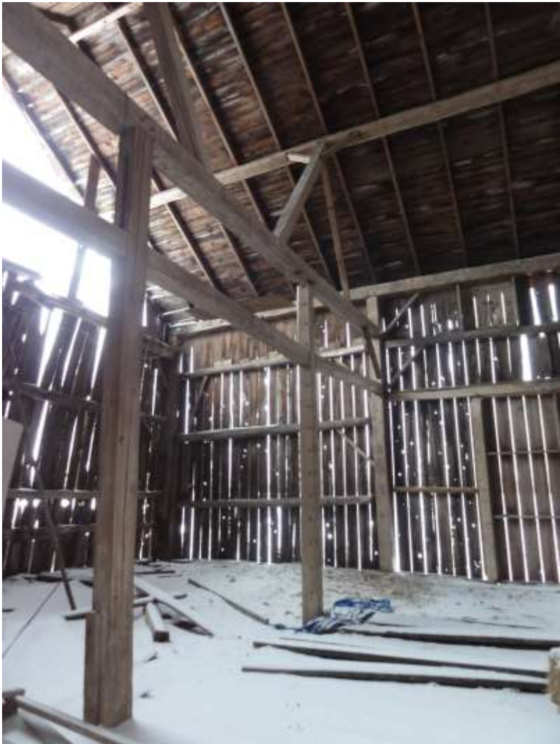
Image 7: View of barn interior illustrating damaged exterior bent and cladding, east face (2019-02-14).
