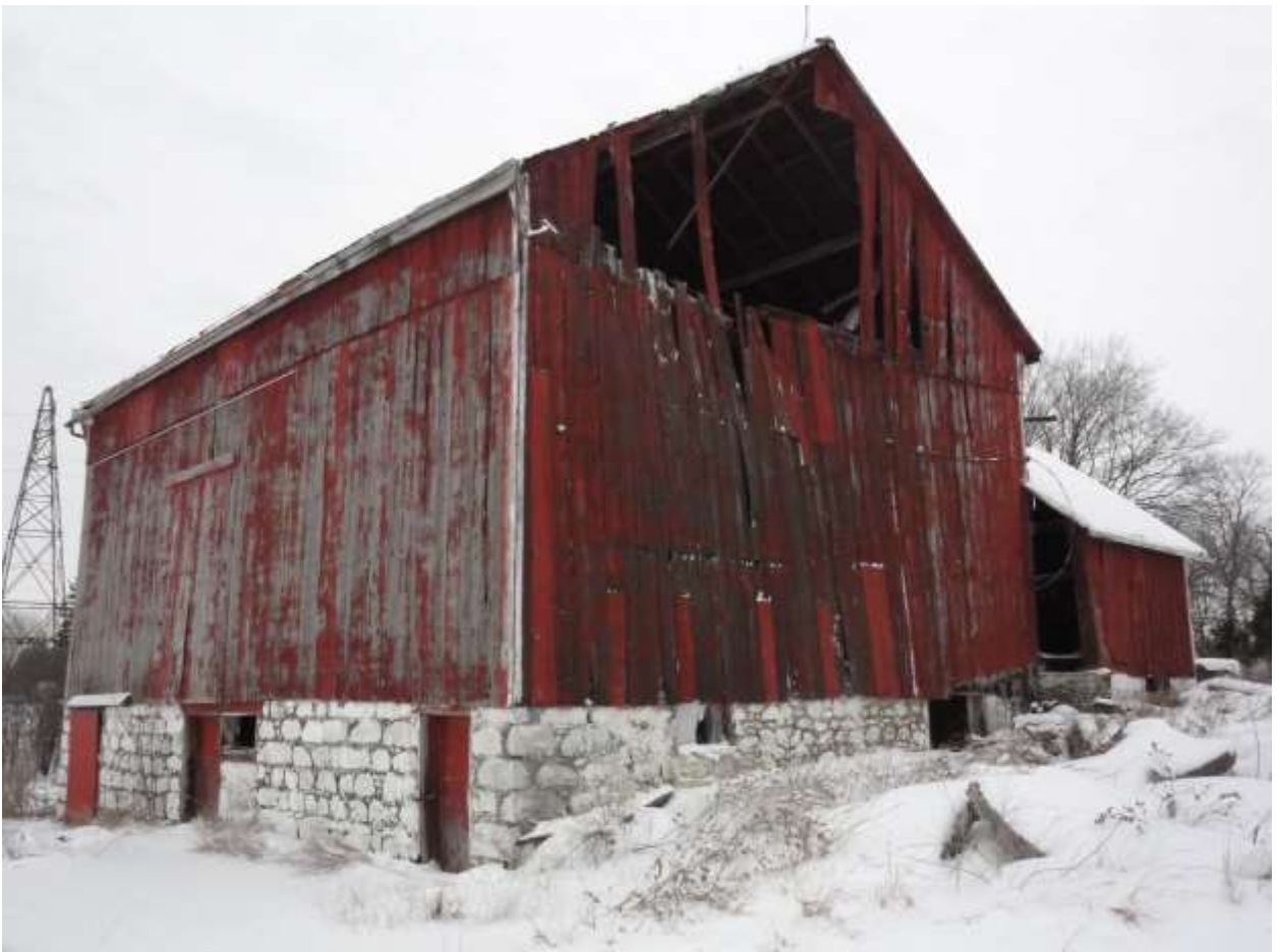
Image 4: View of barn, east-south corner illustrating gangway, rubble foundation and lower stable level (2019-02-14).
