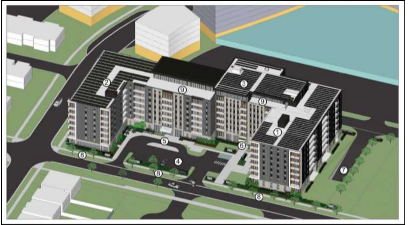
Aerial perspective looking south-east towards the Shore Road frontage.
