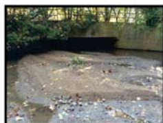
Photo 23: Sediment deposition downstream of Proudfoot Lane. The culvert is also full of sediment.
