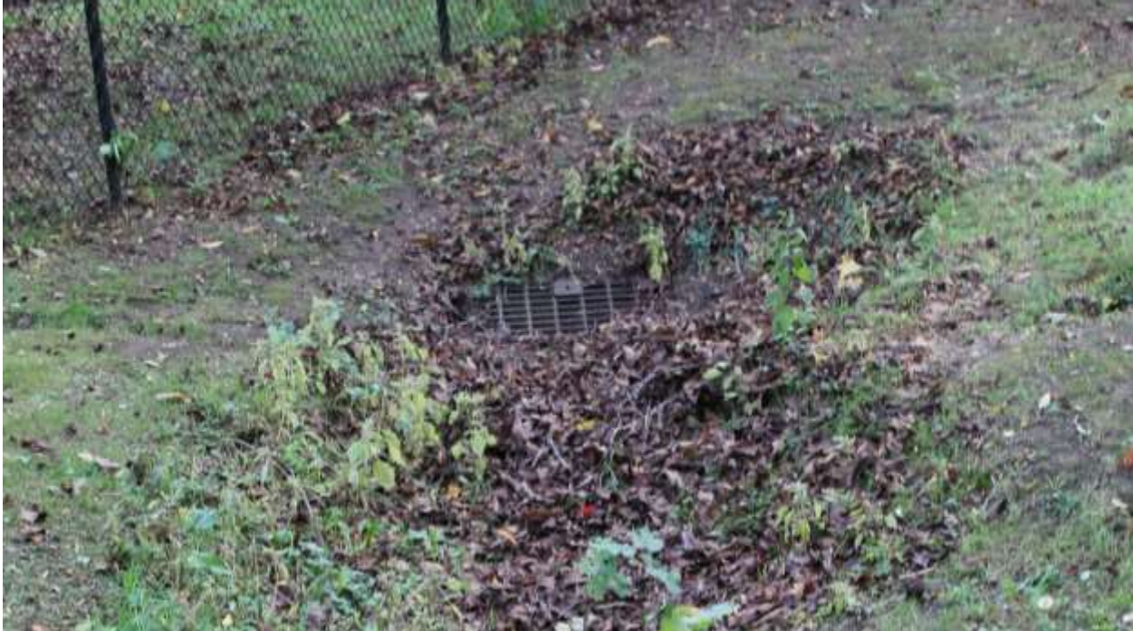
Figure 3: Stormwater inlet/catchbasin on 542 Windermere Road
