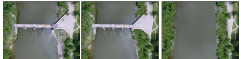
Partial Dam Removal
