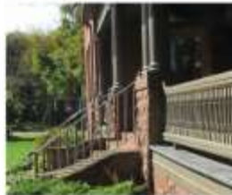
12. Porch: sandstone plinths, balustrade, columns, frieze, decking
