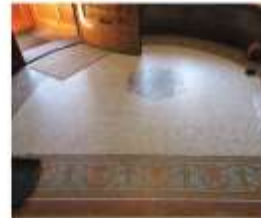
14. Mosaic tile in the front foyer (interior)
