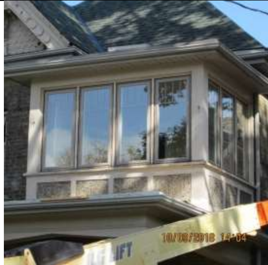
Image 9: Solarium windows – after alterations
