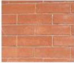
5. Red brick exterior cladding
