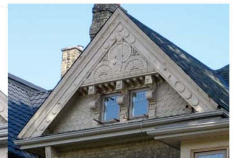
508 Waterloo Street after removal of the attic windows
