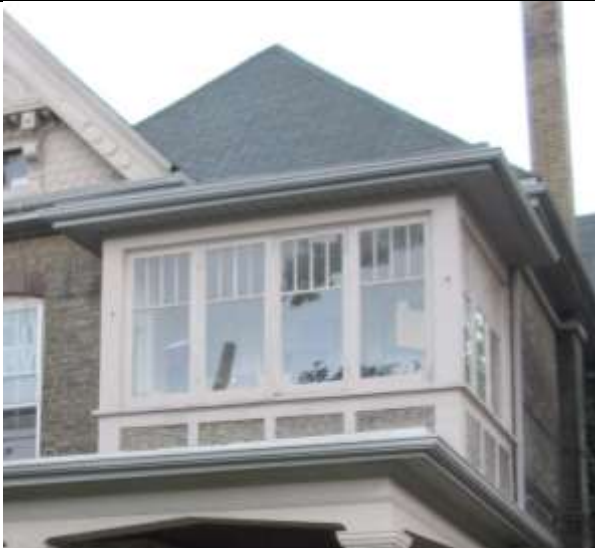
Image 8: Solarium Windows c.2016
