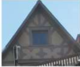
9. Half-timbering of the end-gables (north gable shown)
