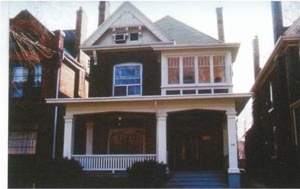
Image 1: 508 Waterloo Street (c.1990)
