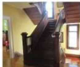
16. Wood, bifurcated main staircase (interior, second storey)
