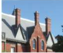
10. Four chimneys with decorative brick detailing (three shown)
