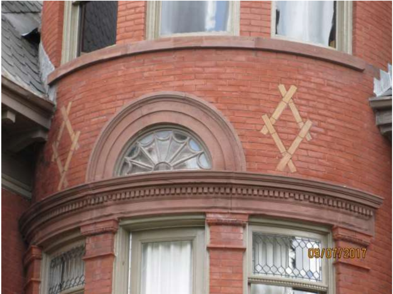
Image 5: Detail of the brickwork detailing, sandstone lintels, and leaded windows forming one of the Palladian windows found at Kenross.
