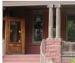
13. Oak enclosure/vestibule at the front door
