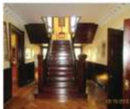
16. Wood, bifurcated main staircase (interior, first storey)
