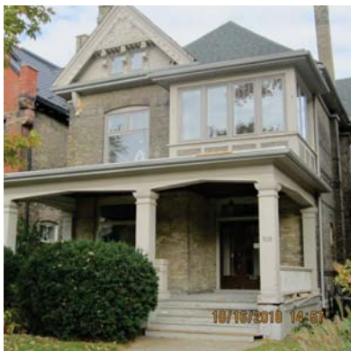
508 Waterloo Street after alterations
