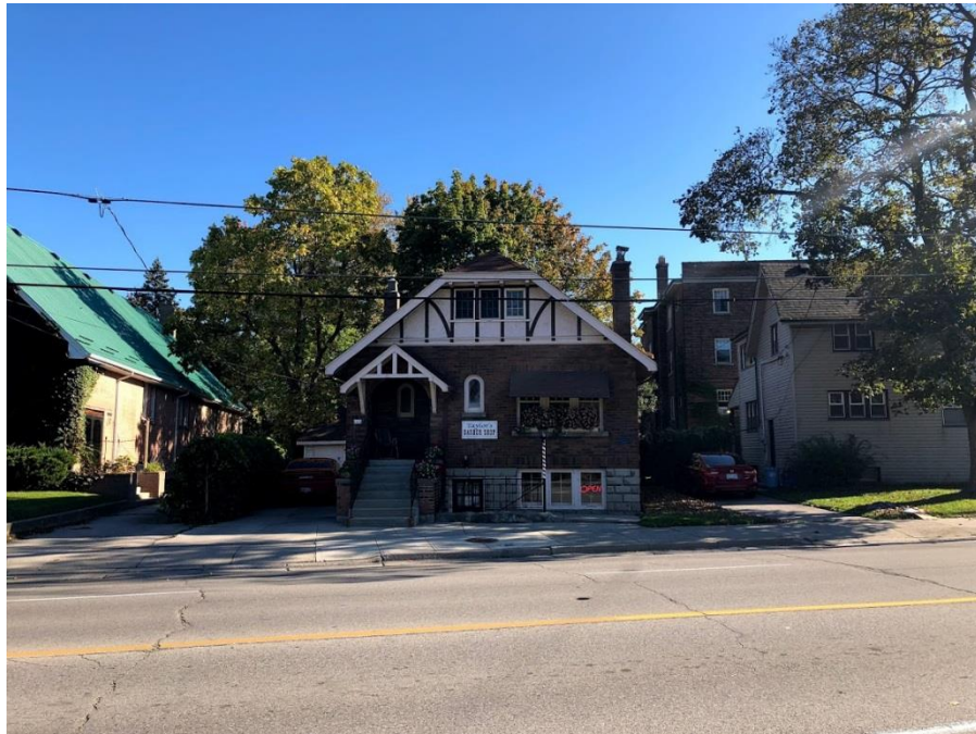
Image 4: View of front elevation of the building located at 1110 Richmond Street, looking east
