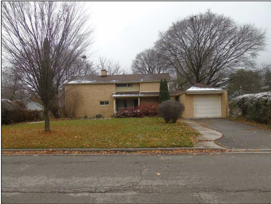
Image 13: View of the rectory at 49 Foxbar Road, located adjacent to the 1957 church building (AECOM, 2018)
