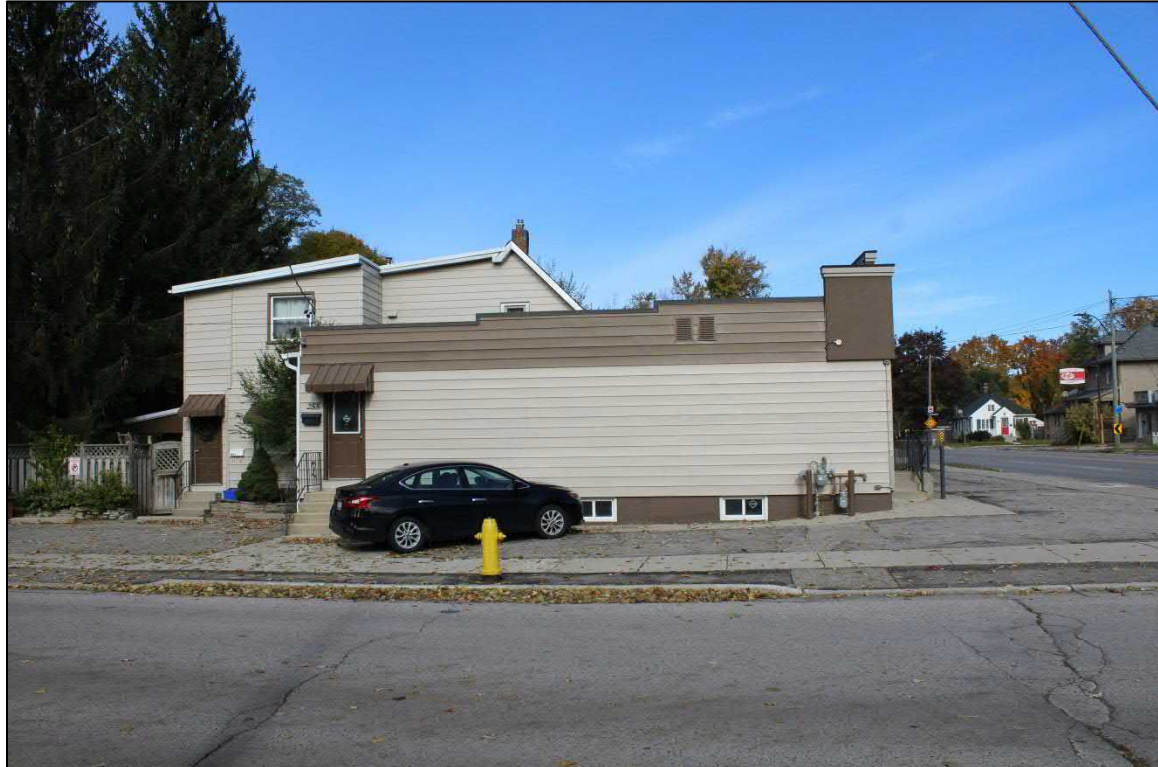
Image 4: South elevation, 255 Wellington Road; the two-storey residential unit at left appears to be a later addition. (AECOM, 2018)
