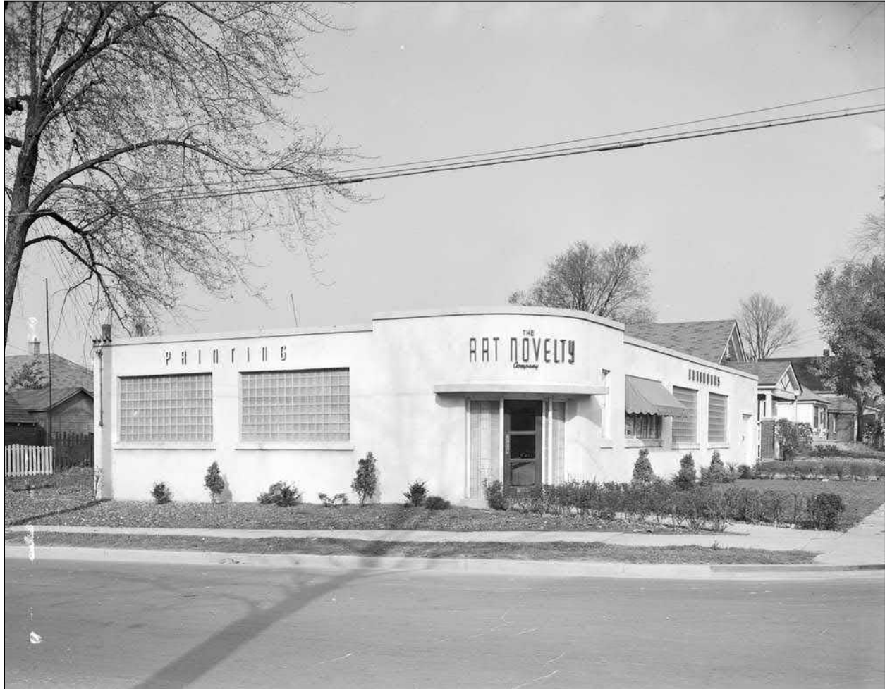
Image 7: 16 Wellington Road circa 1948, showing the building occupied by the Art Novelty Company, shortly after its completion. The existing extension on the north (left) side of the building was added at a later date. (Western Archives, Western University via Historypin.net)
