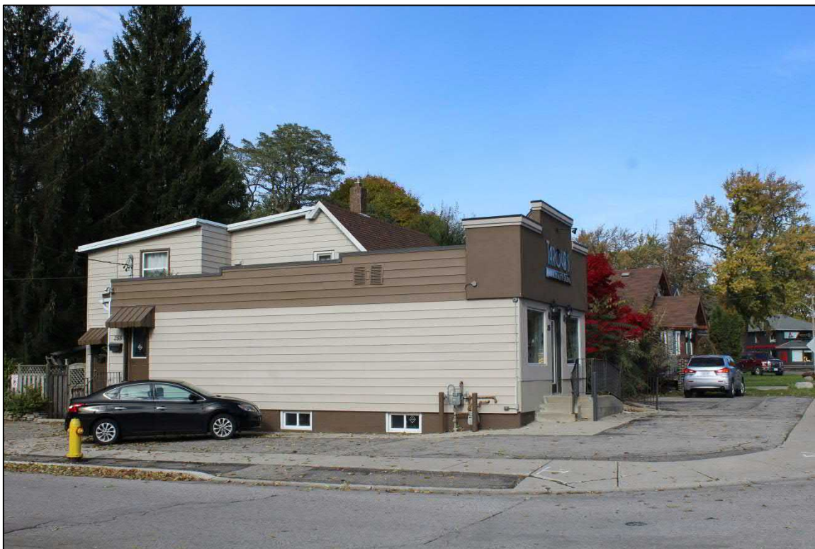
Image 6: South elevation, showing stepped cornice and boomtown style front. (AECOM, 2018)
