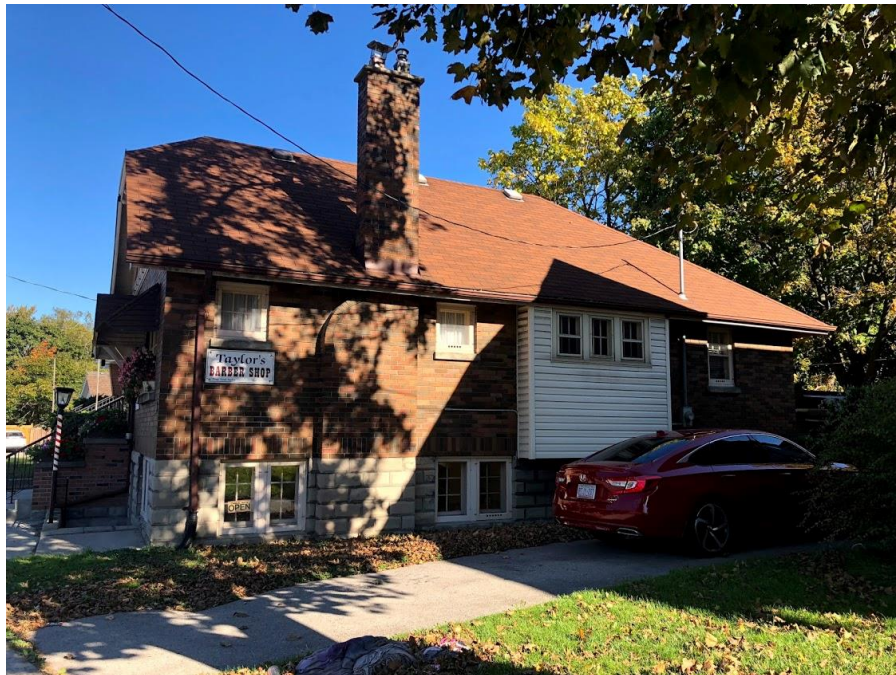
Image 12: View of south elevation including the curved detail of the chimney of the building located at 1110 Richmond Street
