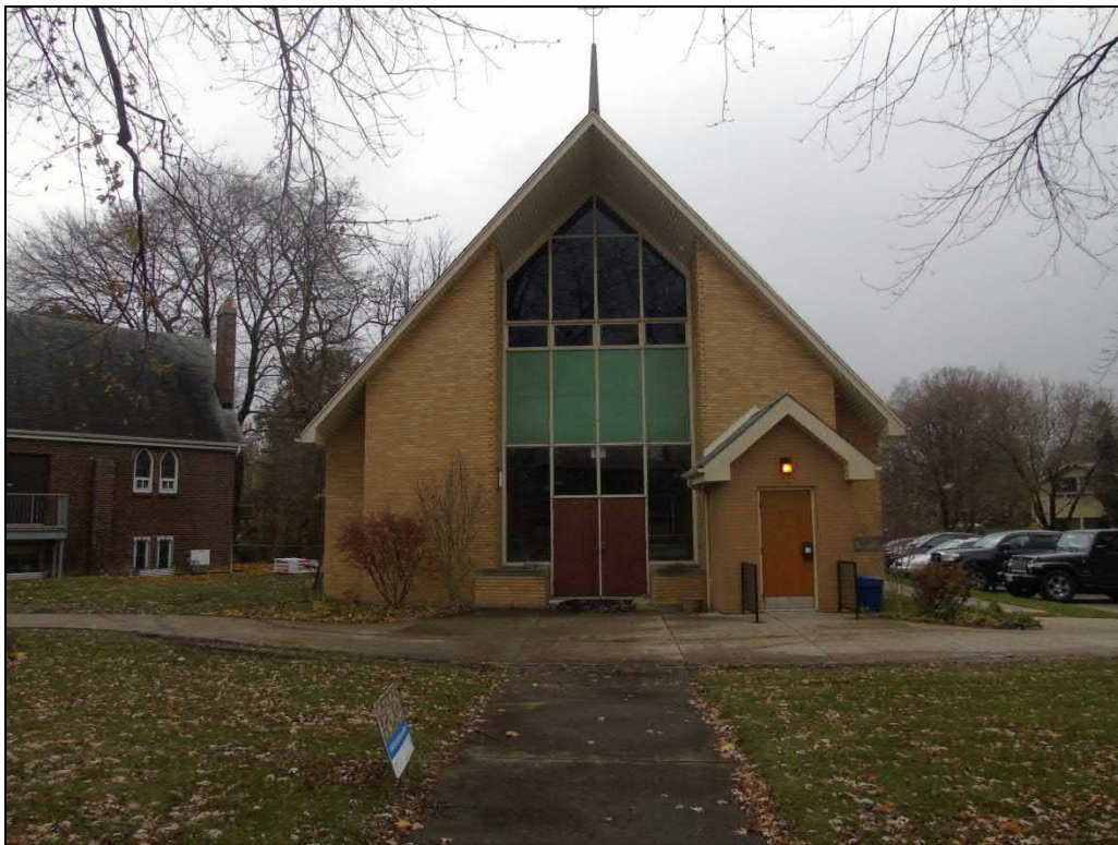
Image 7: East elevation of 1957 church showing design with steep gable roof. (AECOM, 2018)
