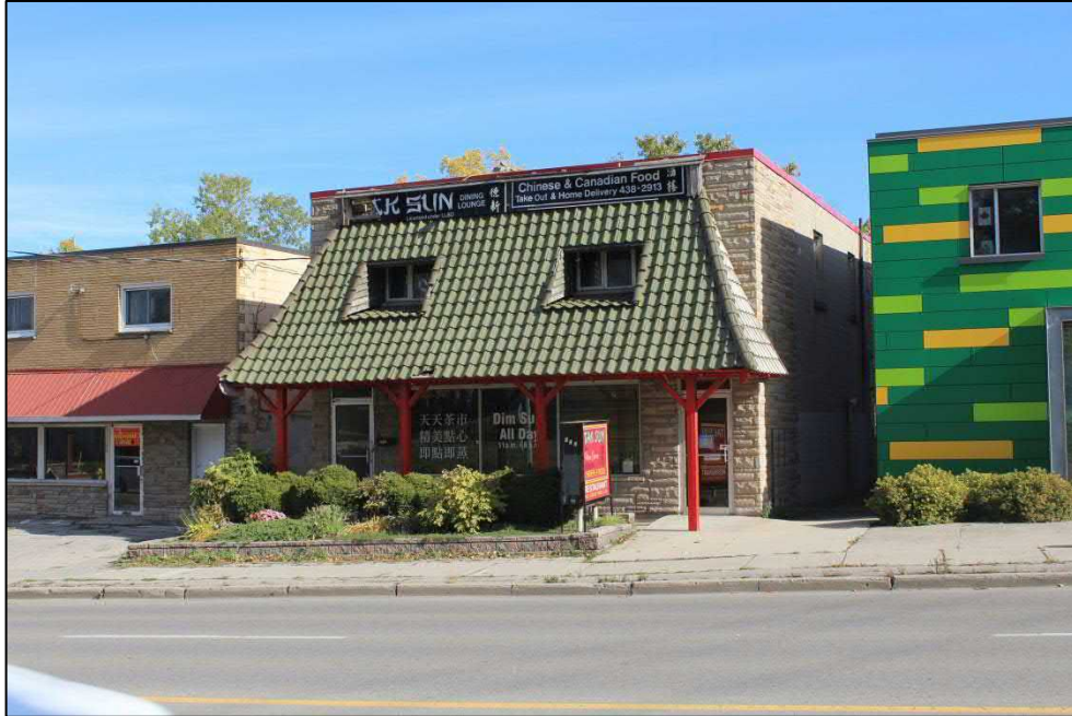
Image 1: Front (west) elevation of 122 Wellington Road. (AECOM, 2018)
