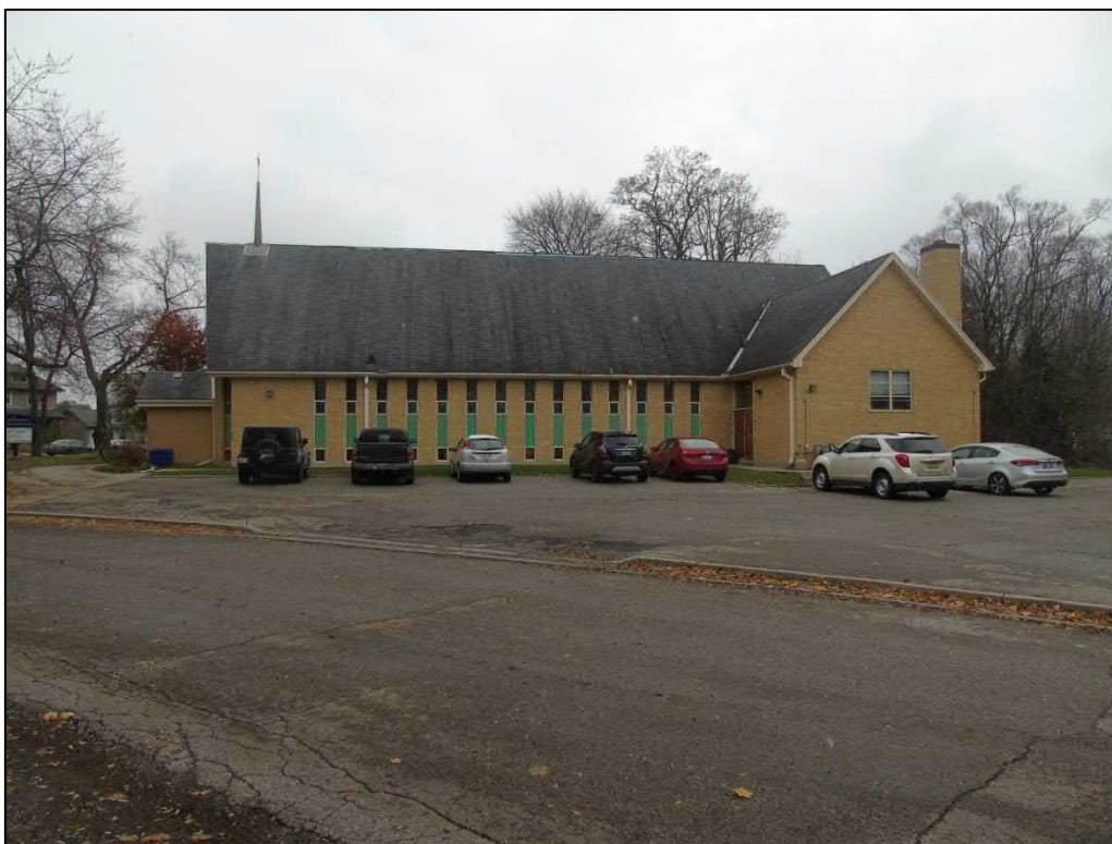
Image 10: North elevation of 1957 church, showing narrow vertical windows and intersecting side gable roof. (AECOM, 2018)
