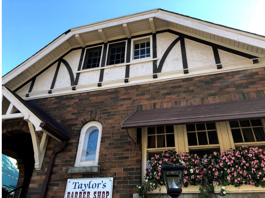
Image 9: View of half timbering in the gable end and the grouping of three windows on front elevation of the building located at 1110 Richmond Street
