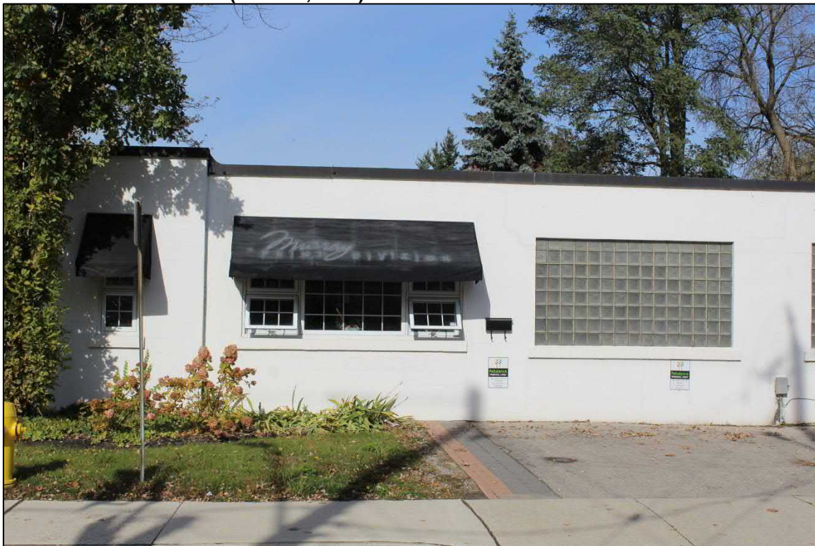
Image 4: Section of south façade showing window treatments and stepped cornice. (AECOM, 2018)
