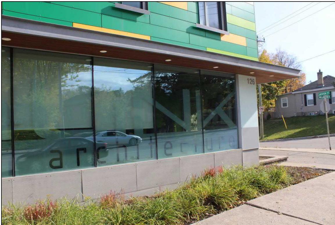
Image 3: Detail of ground floor glazing. (AECOM, 2018)
