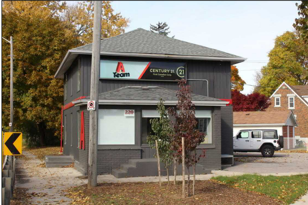
Image 1: Southeast façade, 220 Wellington Road, showing former storefront. (AECOM, 2018)
