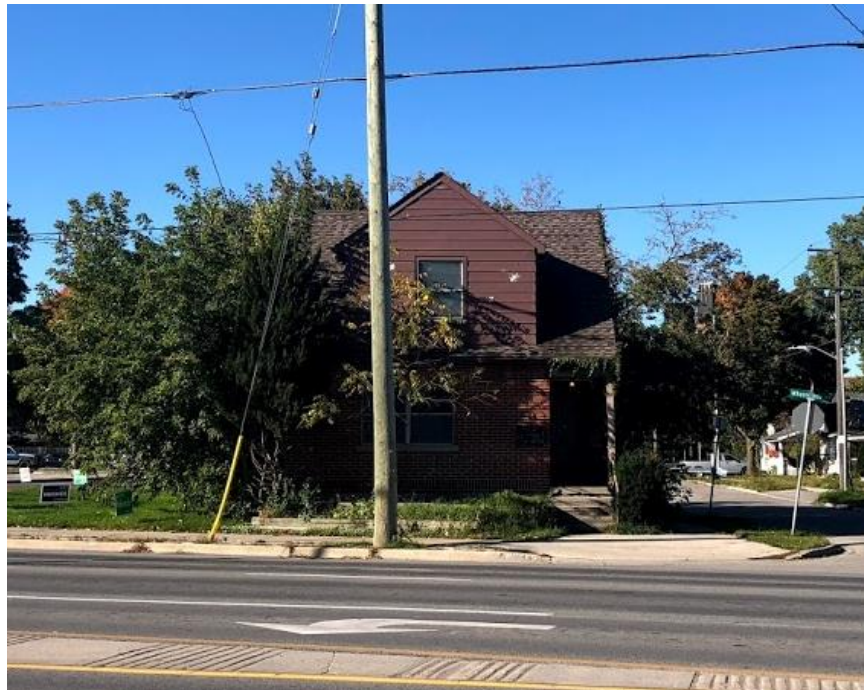
Image 2: View of the front (east) elevation of 44 Wharncliffe Road North, looking west.
