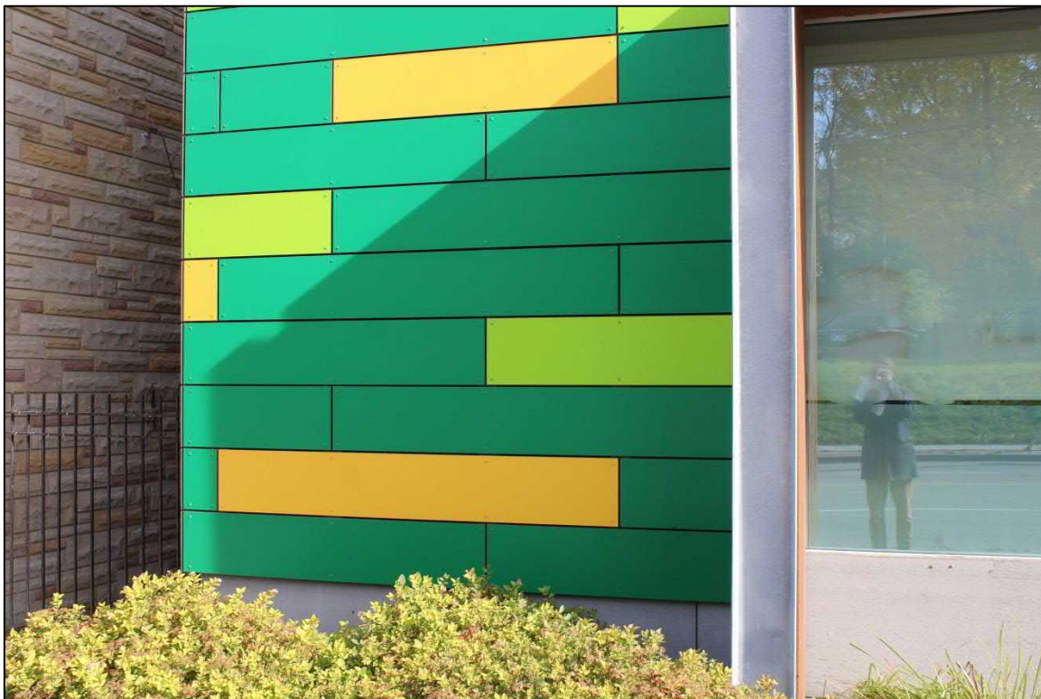
Image 4: Detail of green and yellow cladding added in 2015. (AECOM, 2018)
