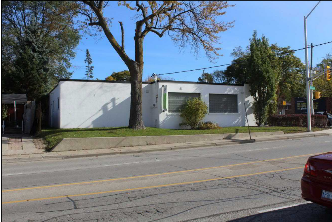
Image 3: West façade of building, facing Wellington Road. The blank wall to the left denotes the extension that was added to the north side of the building sometime after the 1950s (AECOM, 2018)
