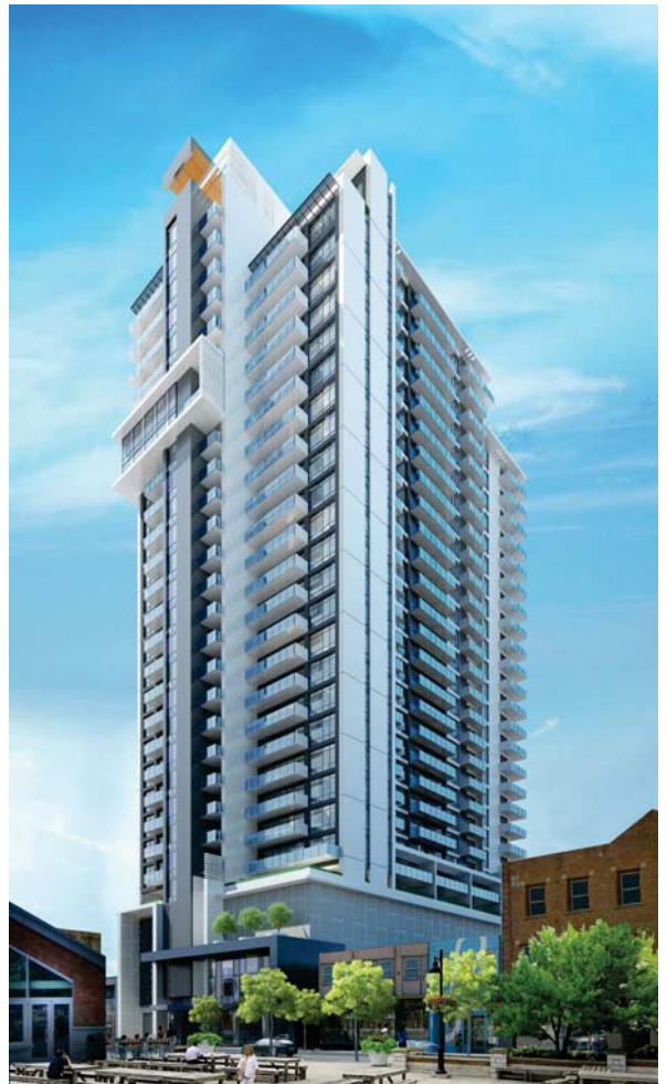
KING STREET LOOKING NORTH
