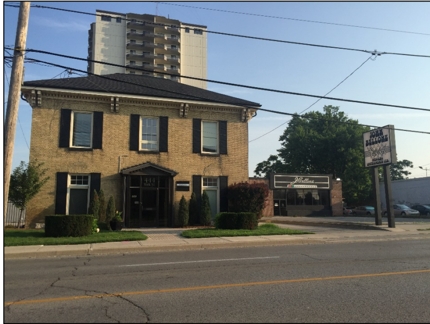
Figure 3 Looking north on York Street toward 444 York Street and 446 York Street
