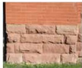
4. Red sandstone (foundation cladding, coping, lintels)
