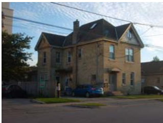
183 Ann Street ( recently purchased by York Development for redevelopment- next to old Carling Brewery site)
