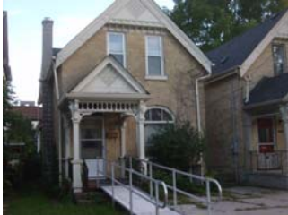
145 Central Ave. Listed on heritage inventory list.
