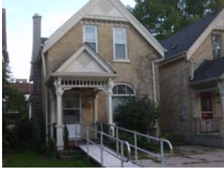
145 Central Ave. Listed on heritage inventory list.
