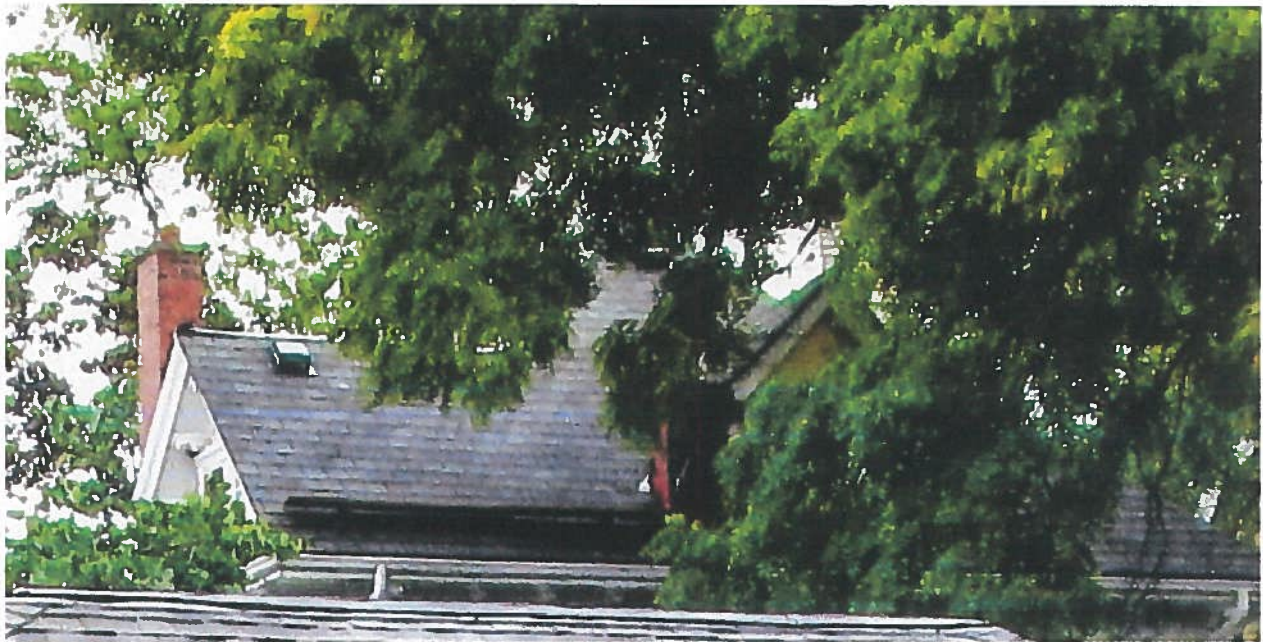
GAF Slateline partially installed on our house
