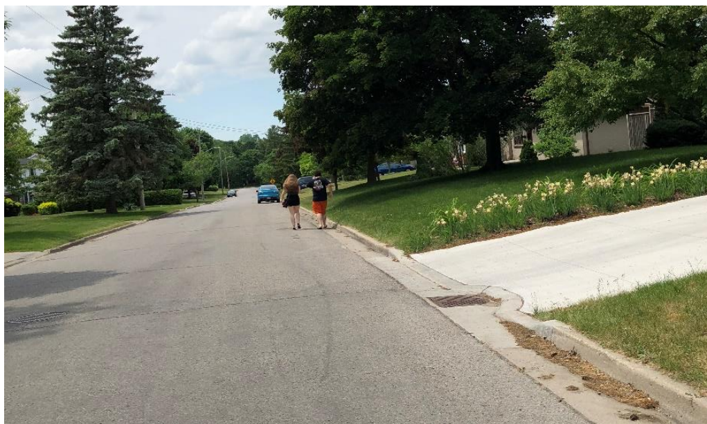
Typical Byron South Street without Sidewalk
