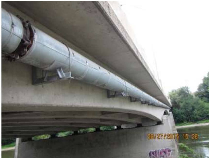
PIPE ALONG WEST SIDE OF BRIDGE - AUG'15
