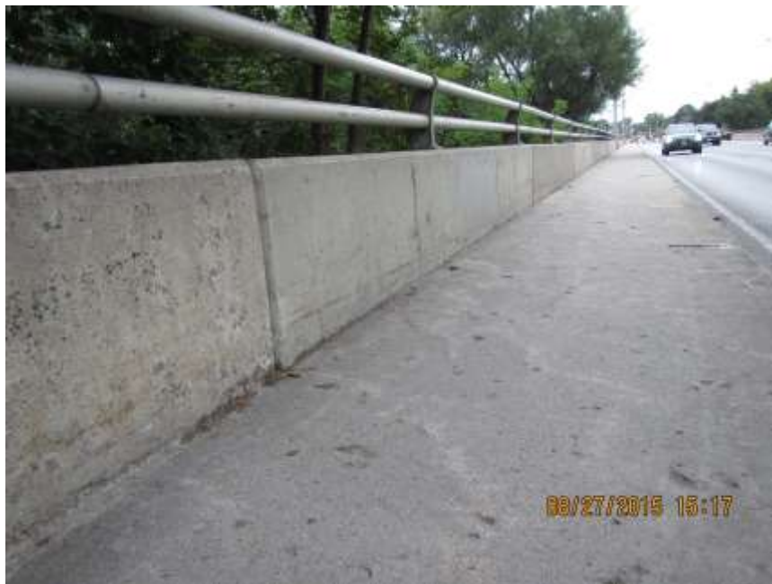
WEST PARAPET WALL - AUG'15
