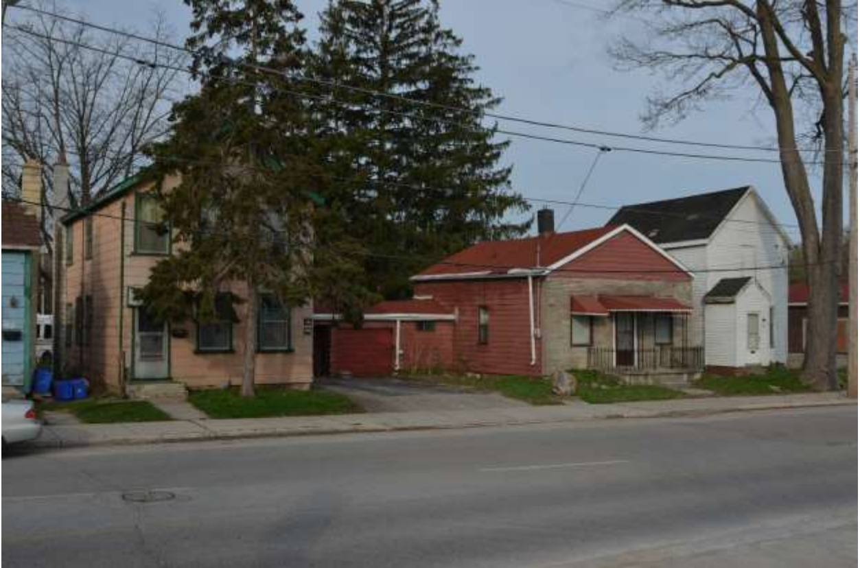
Image 3: Photograph of the property at 275 Thames Street in 2012 showing streetscape
