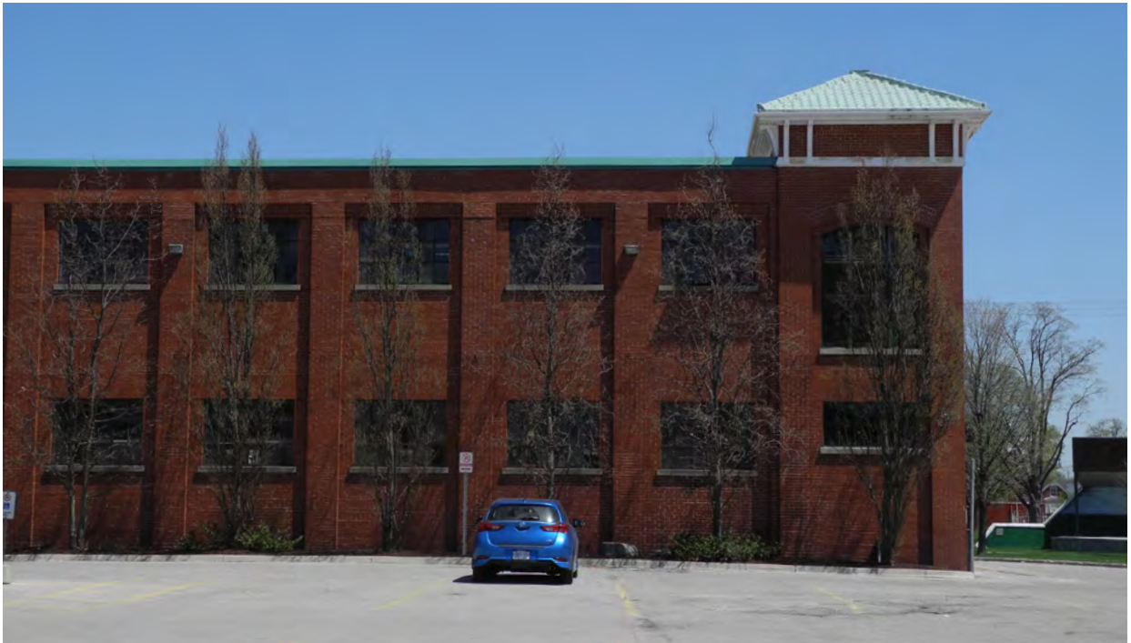
Figure 31 - The south end of the Confederation Building's west elevation, show recessed bays, steel sash windows, and elaborated corner towers (CBCollective 2018).
