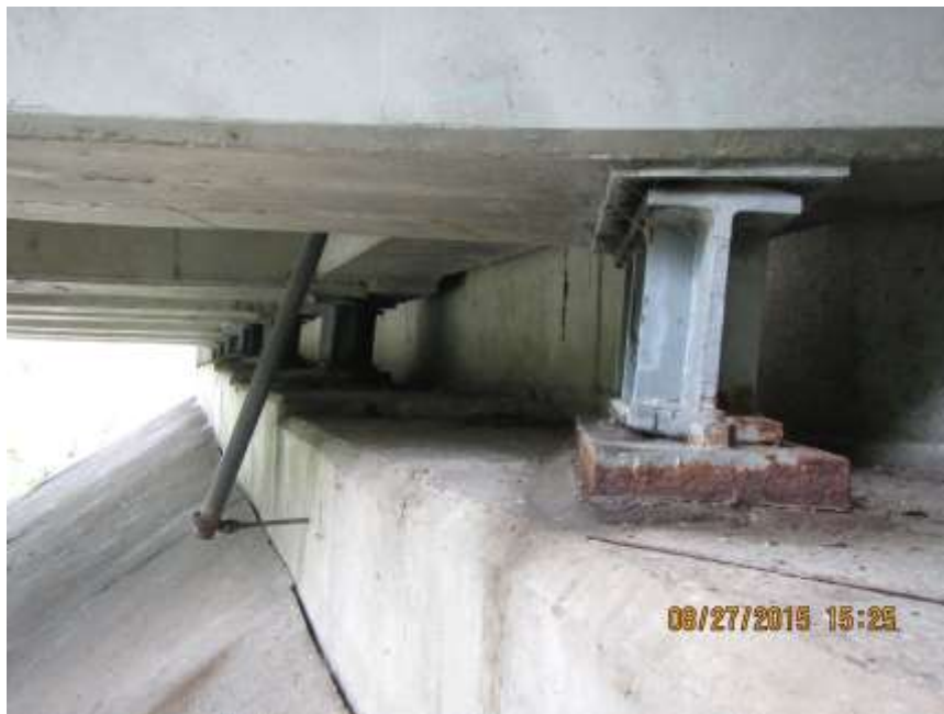
NORTH ABUTMENT - AUG'15
