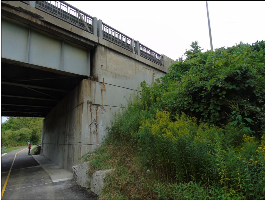
Photograph 14: View showing north abutment
