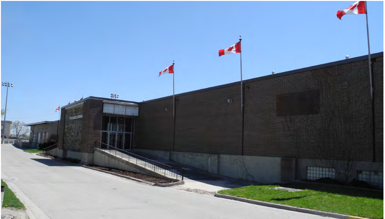
Figure 39 - The north elevation of the Progress Building. The portico at the top of the ramp was a subsequent addition (CBCollective 2018).
