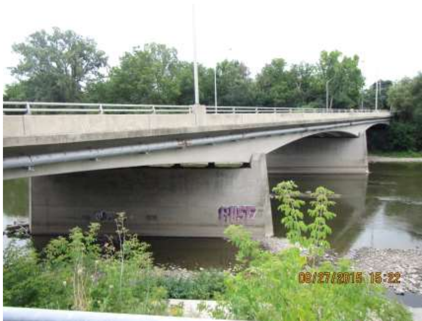
WEST ELEVATION LOOKING SOUTH - AUG'15
