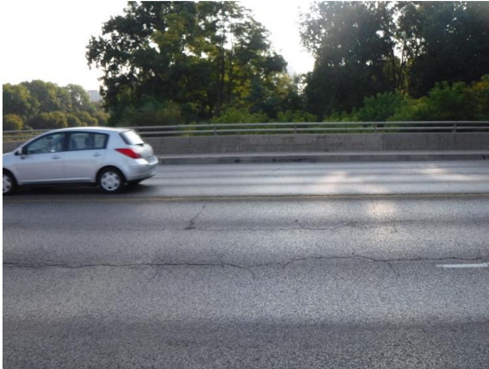
Plate 9: View of the bridge deck and east sidewalk and curb.
