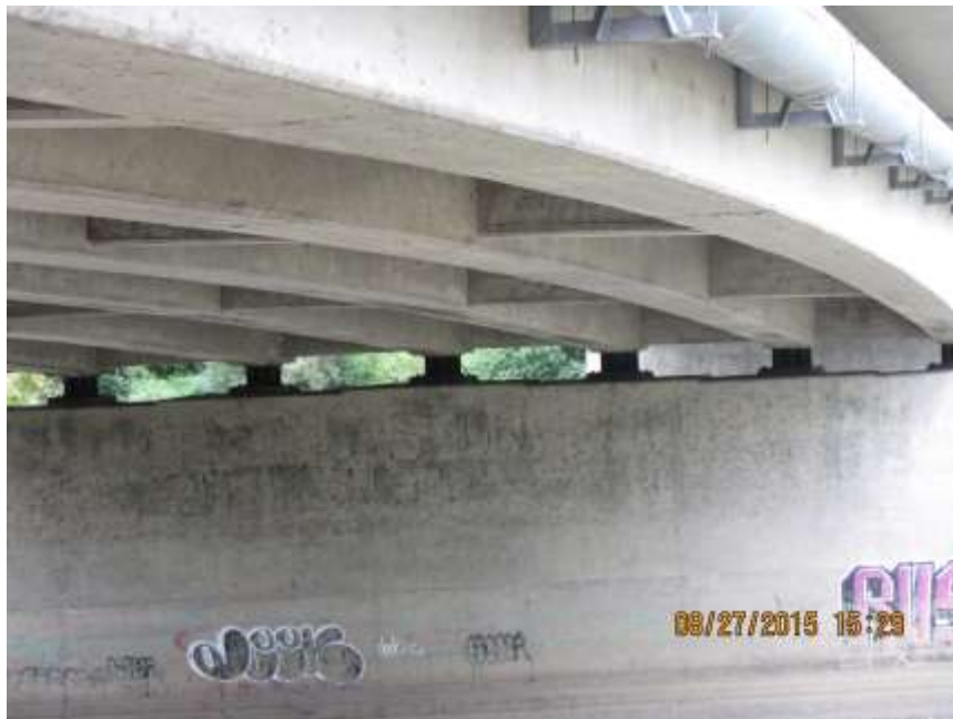
BEARINGS AT NORTH PIER - AUG'15
