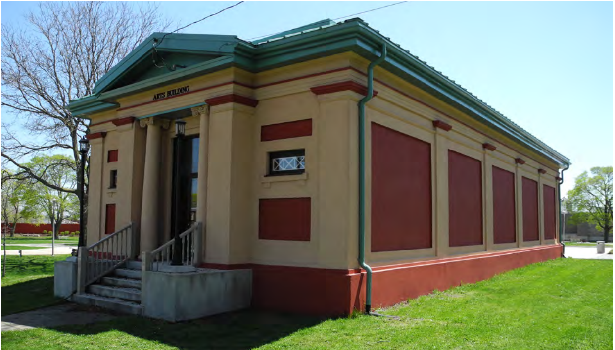
Figure 29 - View southeast onto the principal north elevation of the Arts Building at the north end of Queen's Park. (CBCollective 2018).
