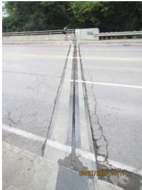
SOUTH EXPANSION JOINT - AUG'15
