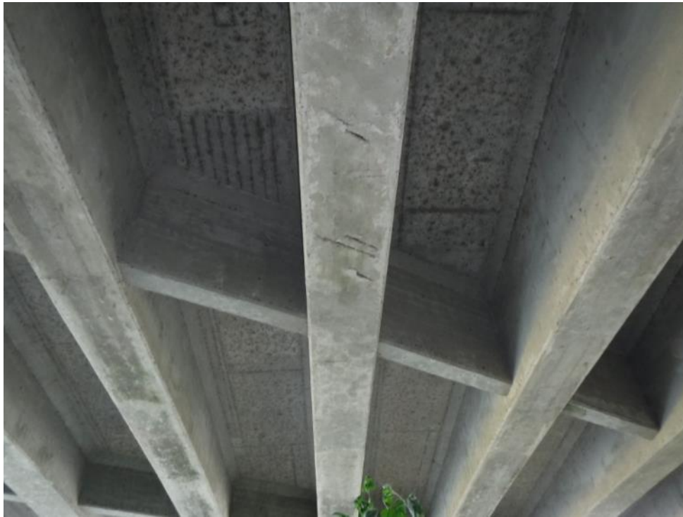
Plate 21: View of the bridge soffit and beams.
