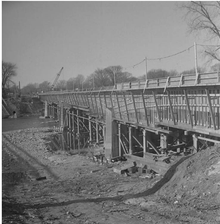
Figure 16: “Wharncliffe Road Bridge is ready for cement”, view northeast Source: LFP Collection of Photographic Negatives, Western Archives, April 13, 1958
