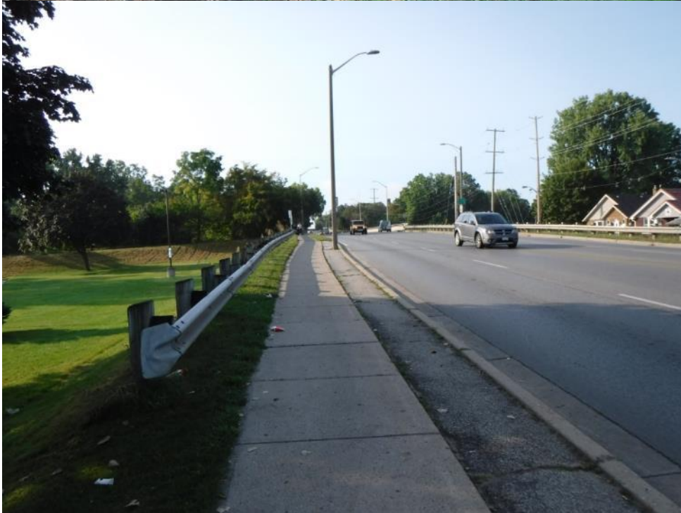
Plate 30: View of the north approach and the Blackfriars/Petersville HCD property to the left of the bridge.
