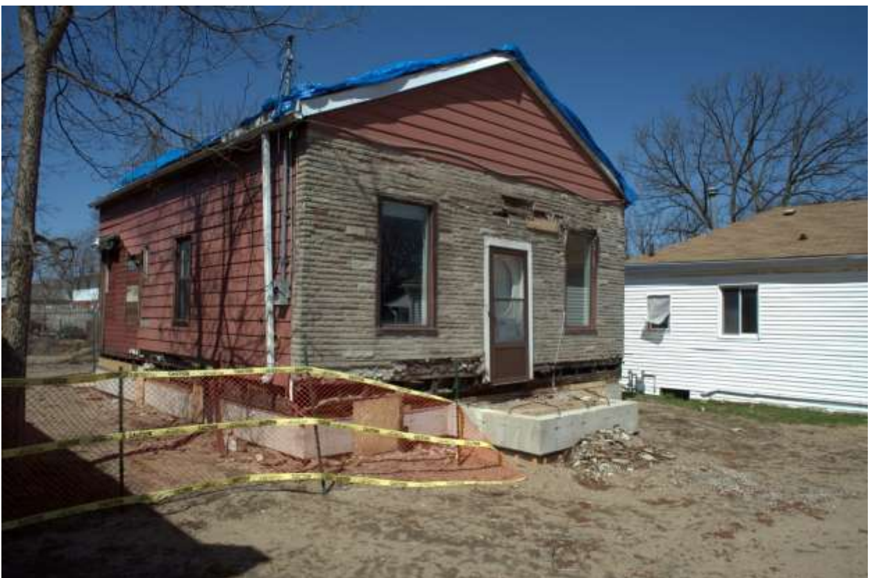
Image 6: Photograph of the Fugitive Slave Chapel building being position onto new concrete foundation at 432 Grey Street, April 24, 2015
