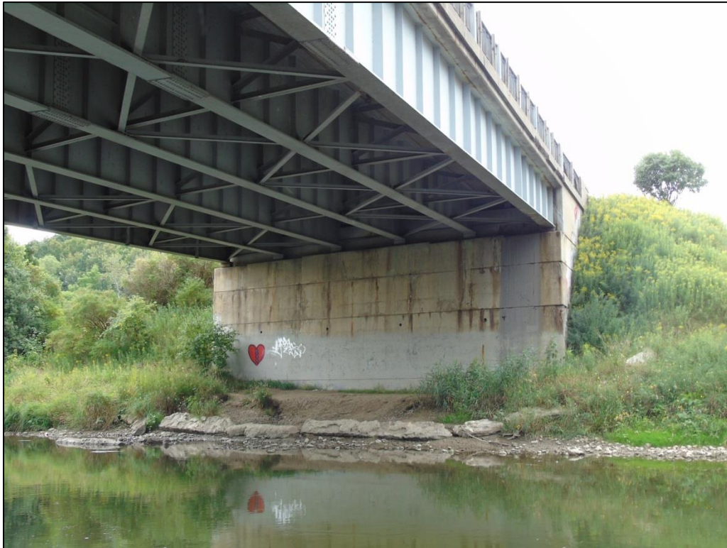
Photograph 16: View from the pier showing south abutment
