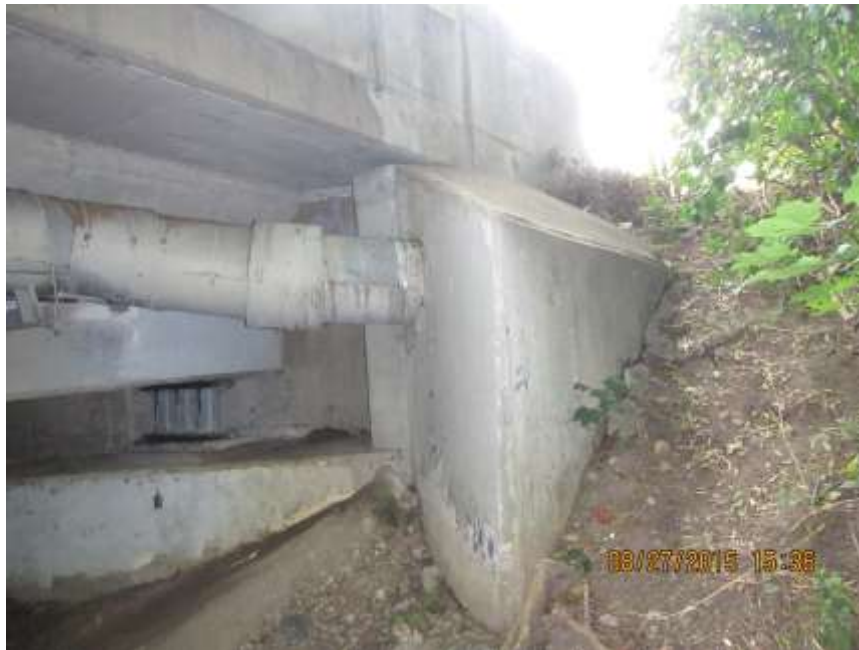
SOUTHWEST WINGWALL - AUG'15
