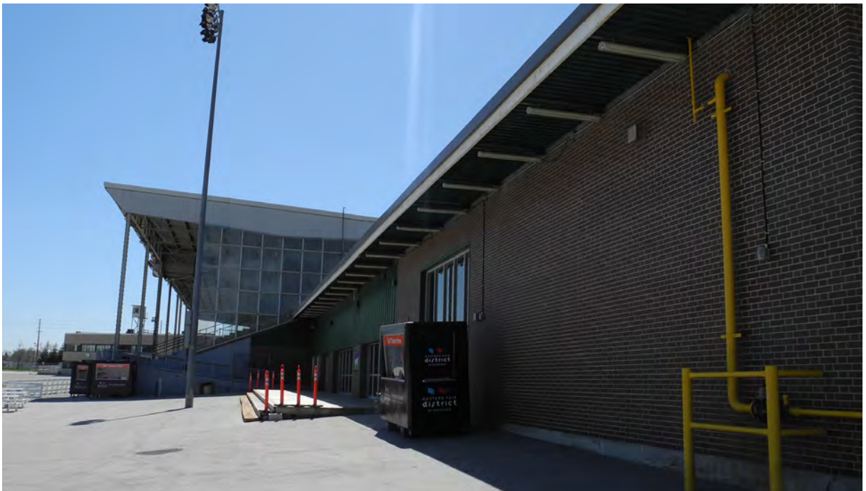
Figure 42 - East elevation of the East Annex, with glazed areas facing onto the racetrack (CBCollective 2018).
