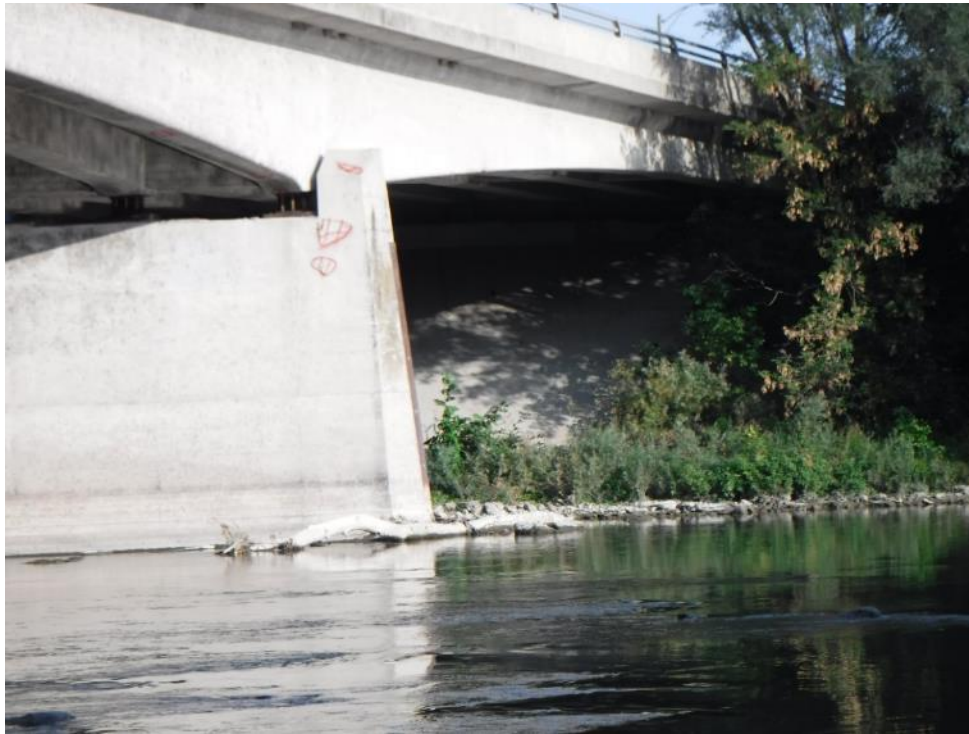
Plate 23: View of the steep backwall and north pier.
