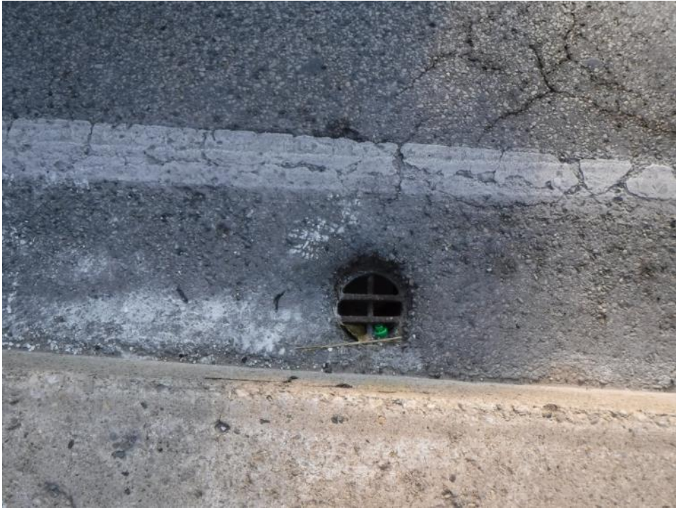
Plate 11: Example of the deck drains.
