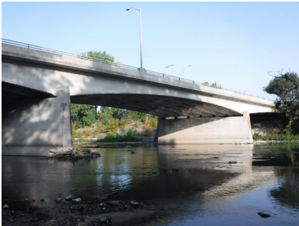
Plate 22: Oblique view of the east elevation.
