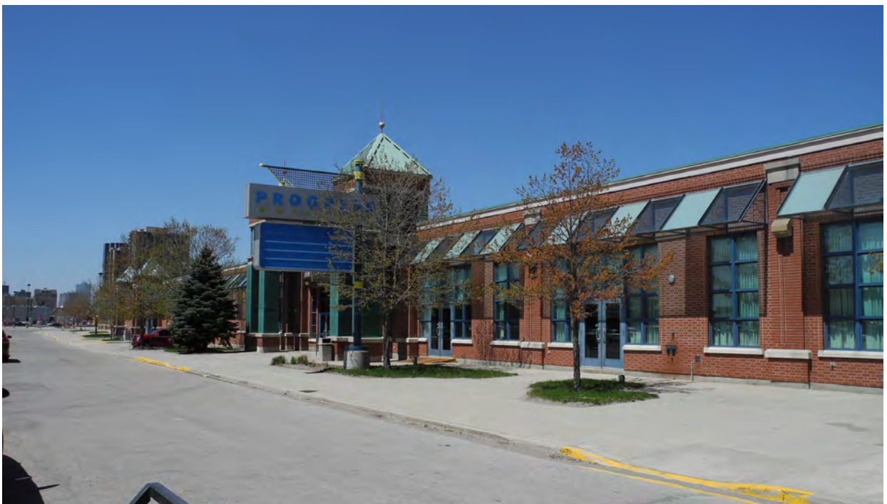
Figure 38 - The Progress Building (right), West Annex (centre), and Canada Building (left) all present as a single elevation, unified with post-modern detailing (CBCollective 2018).
