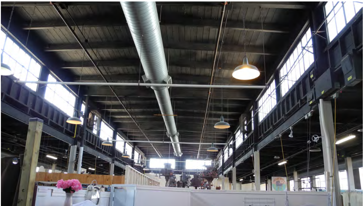
Figure 32 - The substantial, open space on the second storey of the Confederation Building, showing the monitor structure above (CBCollective 2018).
