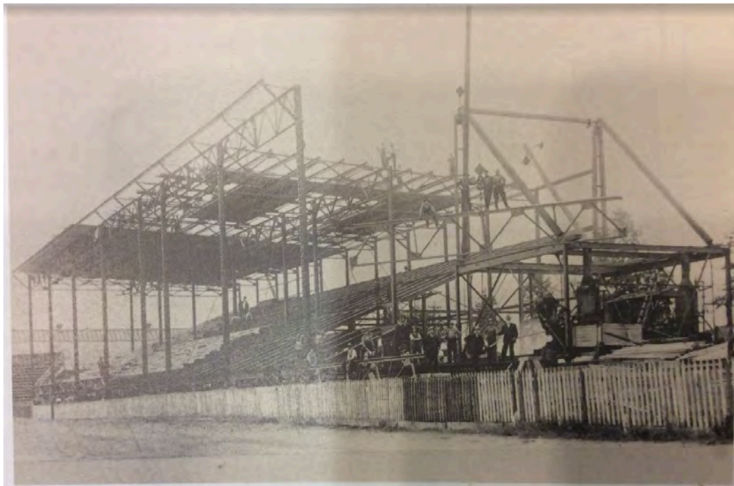
Figure 12 - Construction of the steel and wood Grandstand in c1915 which replaced the wooden Grandstand demolished by fire (Western Fair Archives as reproduced in Celebration of Excellence: the history of the Western Fair Association, 1867-2000, 57).
