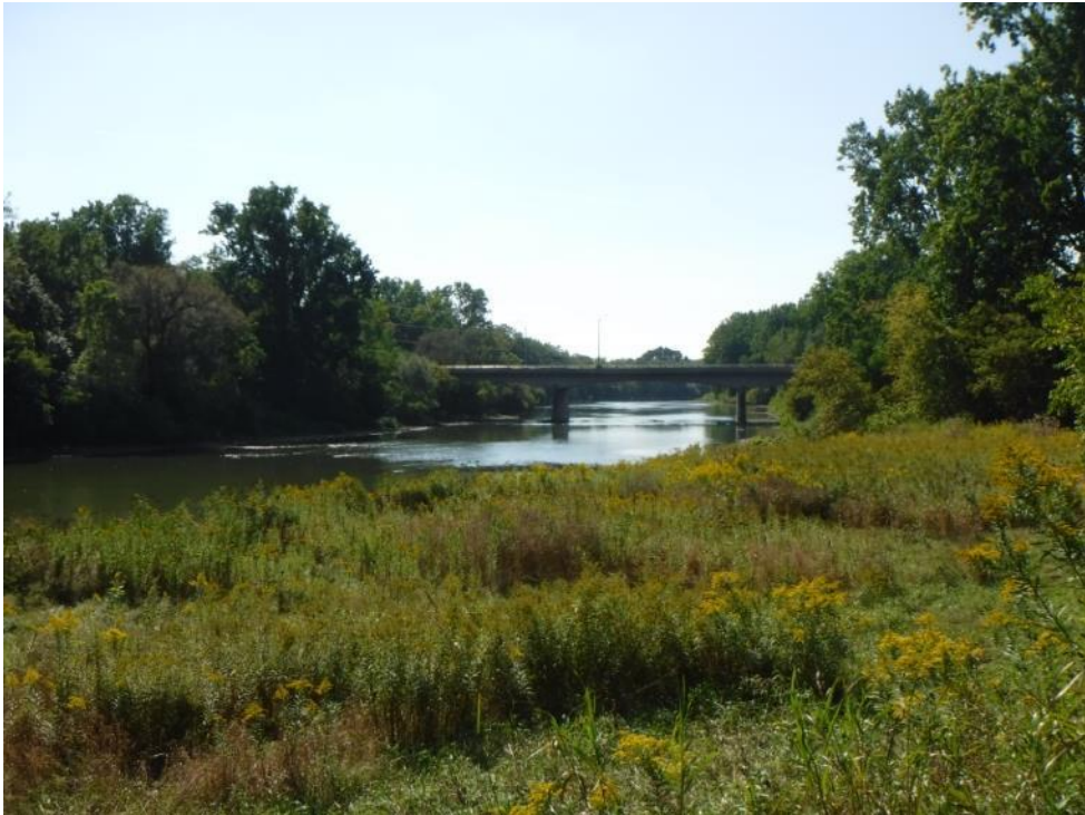
Plate 31: View of the east elevation from within the Thames River Corridor.
