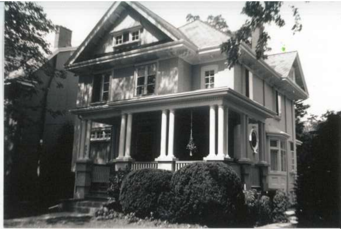
Image 1: View of the property located at 836 Wellington Street (c.1995) – note the slate roof
