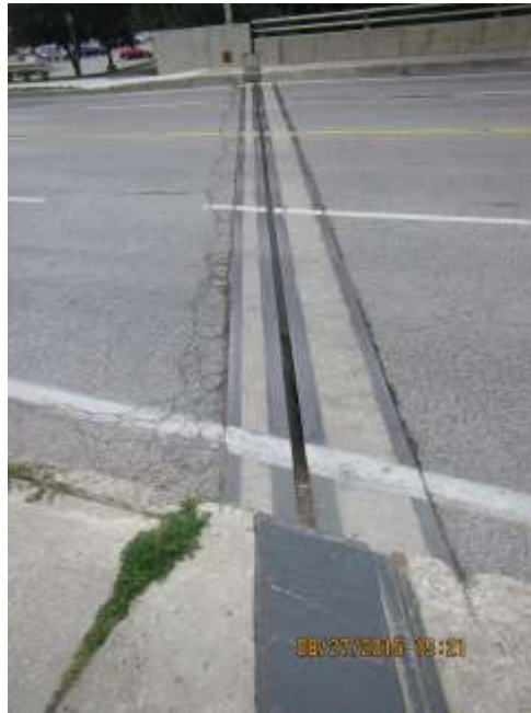
NORTH EXPANSION JOINT - AUG'15
