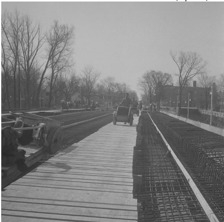
Figure 17: Pouring cement at Wharncliffe Road Bridge, view south Source: LFP Collection of Photographic Negatives, Western Archives, April 14, 1958
