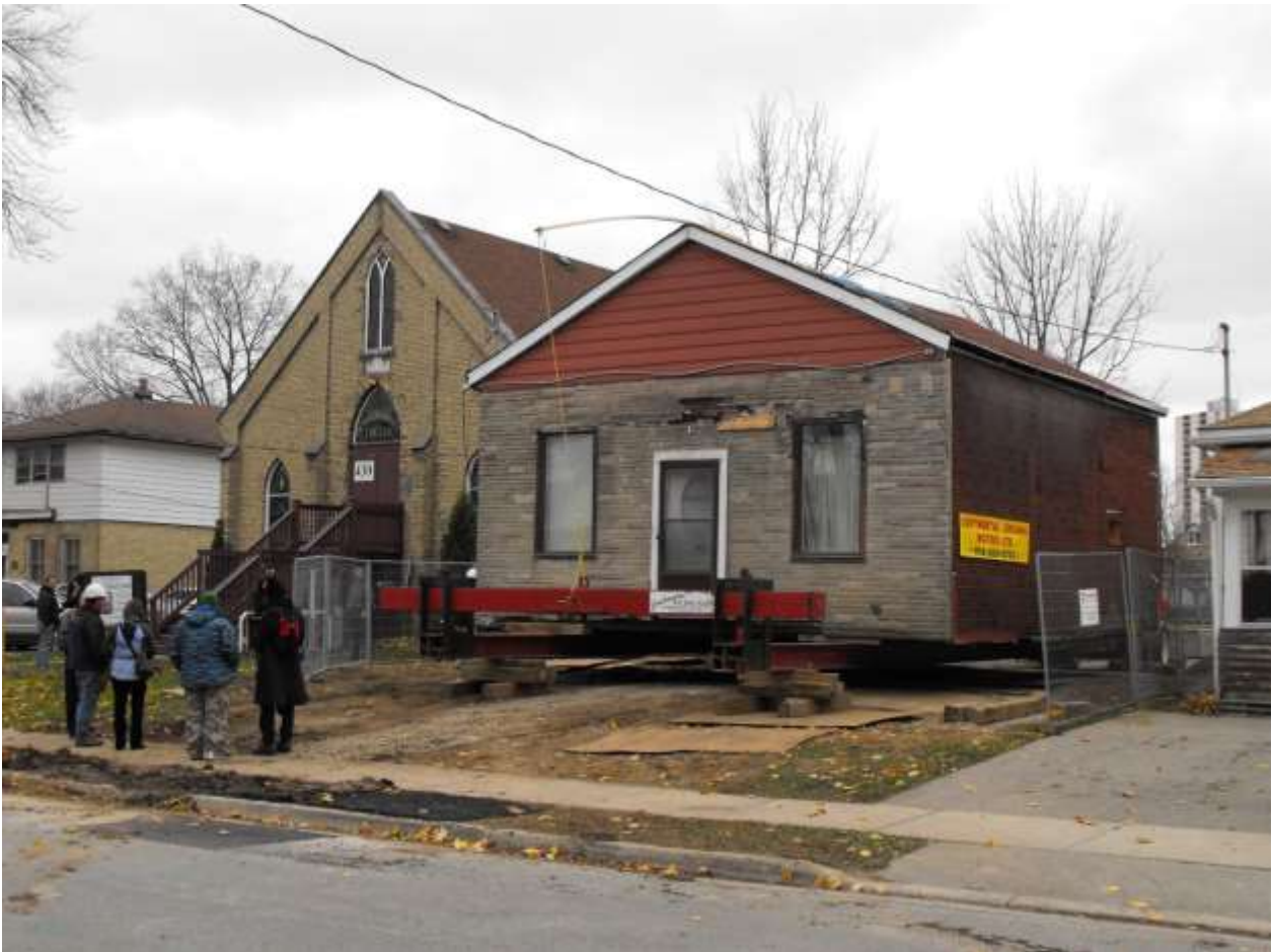
Image 5: Photograph of the Fugitive Slave Chapel building being relocated to 432 Grey Street, November 11, 2014
