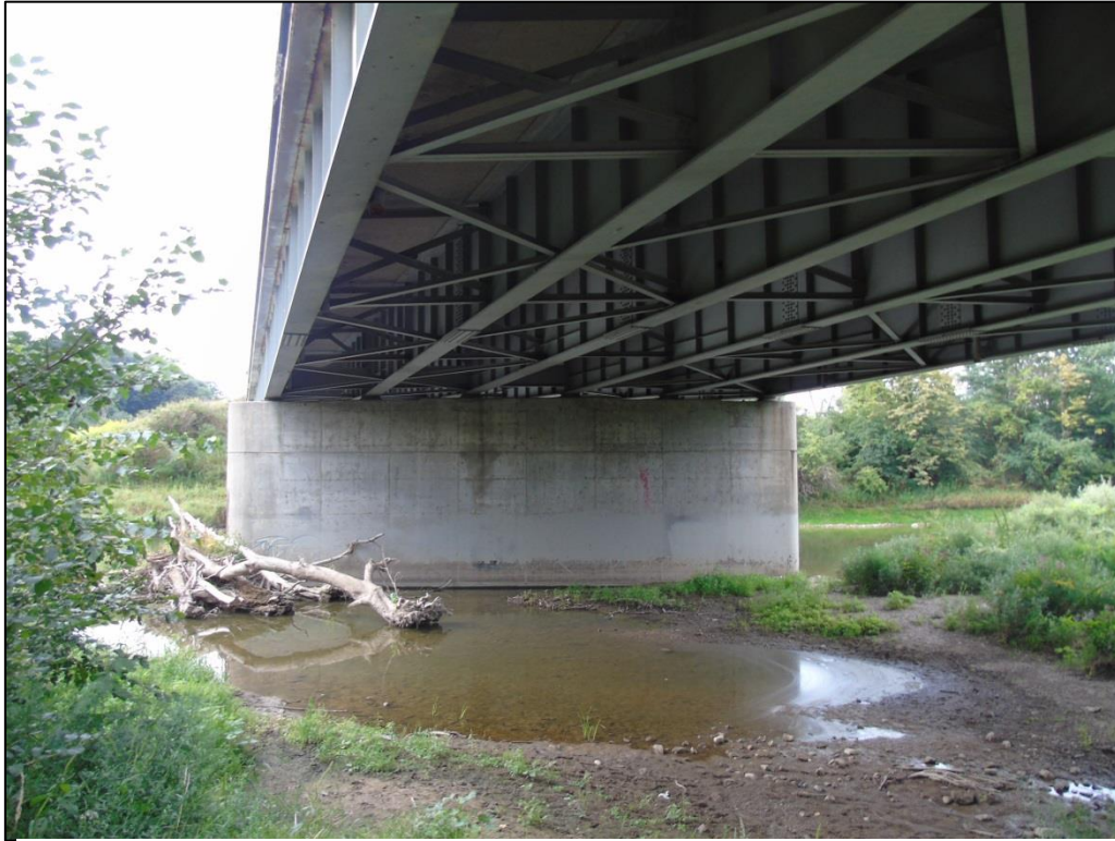
Photograph 18: View showing east side of the centre pier
