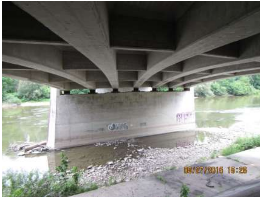
NORTH PIER - AUG'15
