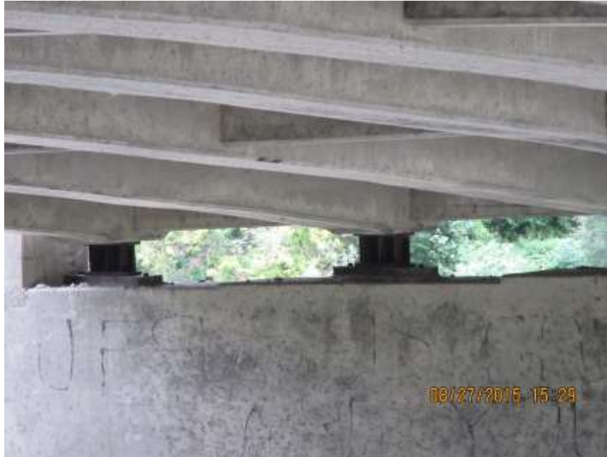
BEARINGS AT NORTH PIER (2) - AUG'15
