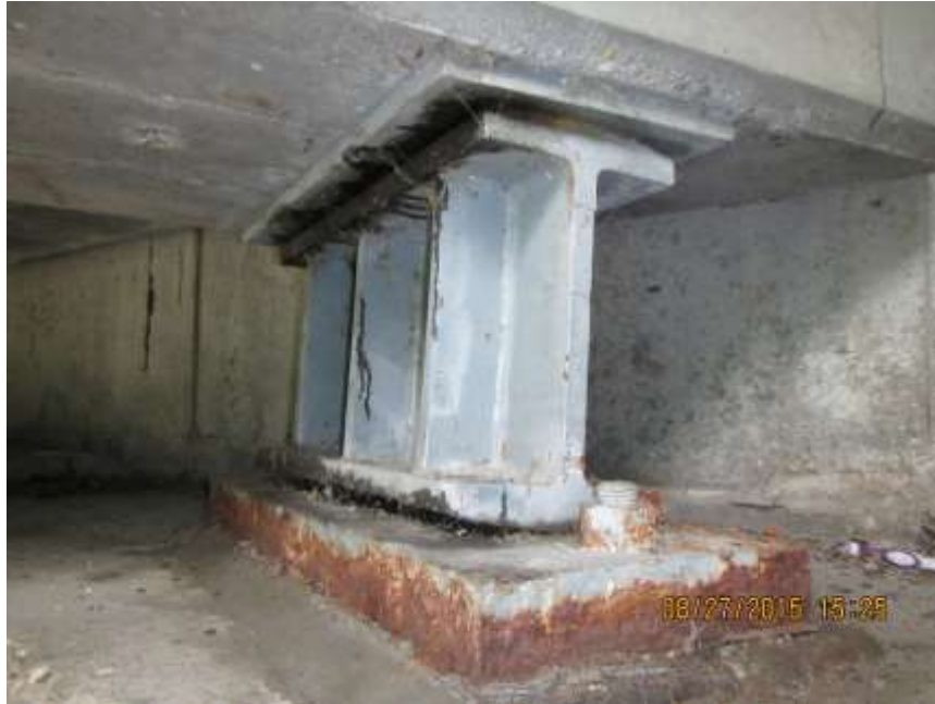
TYPICAL ROCKER BEARING - AUG'15
