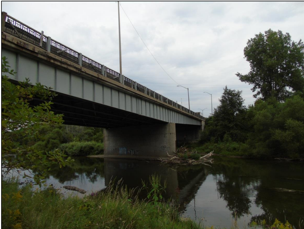
Photograph 5: View showing west side of the Wenige Expressway Bridge
