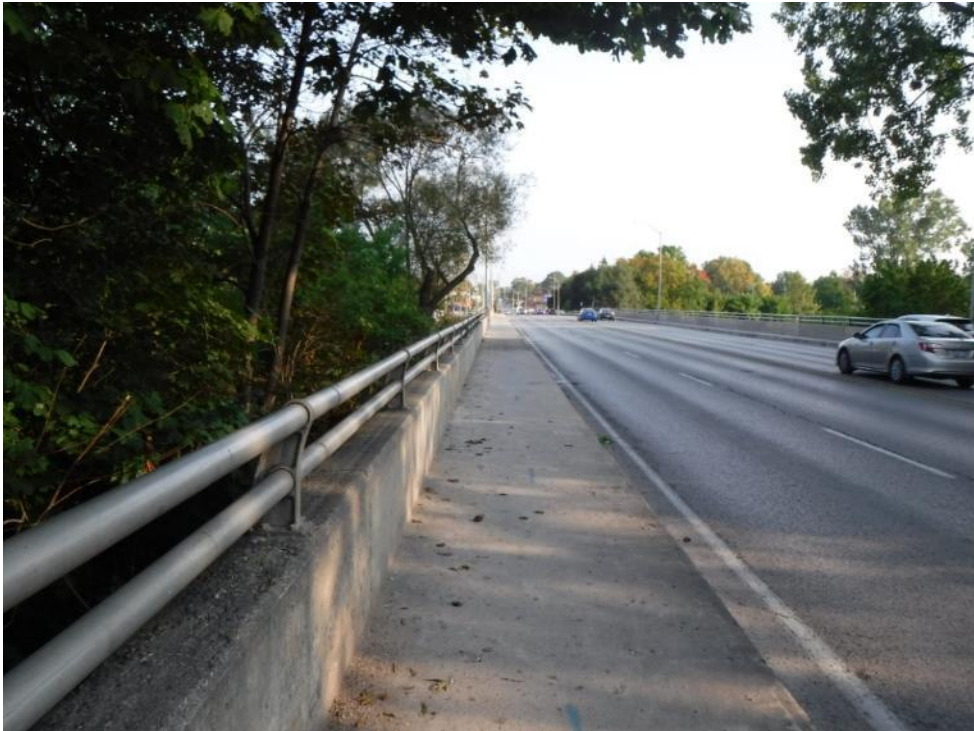
Plate 13: View of sidewalk, looking north.
