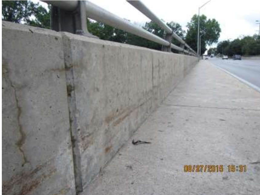
EAST PARAPET WALL - AUG'15
