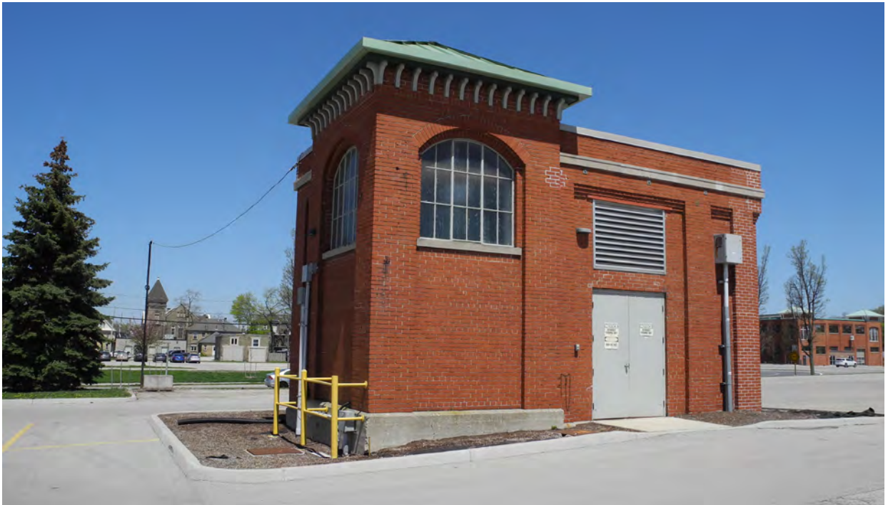
Figure 37 - The Electrical Substation utilizes the former southwest corner of the historic Poultry Building (CBCollective 2018).
