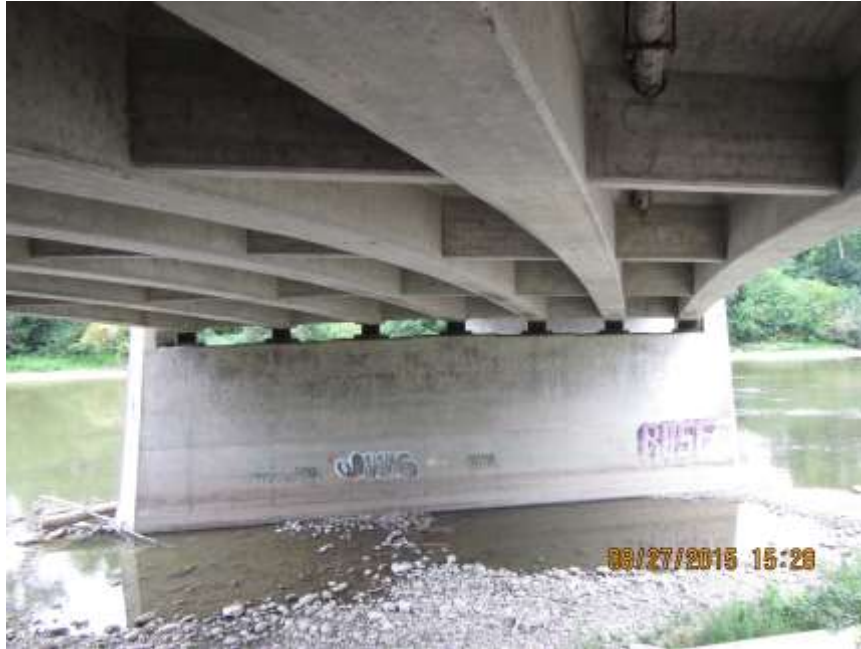
NORTH SPAN - AUG'15
