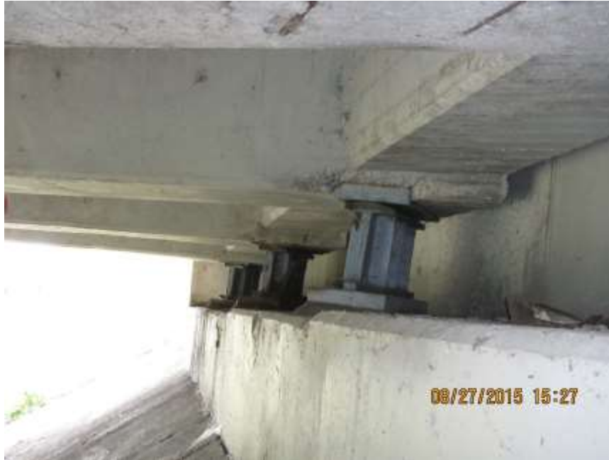
NORTH ABUTMENT BEARINGS - AUG'15
