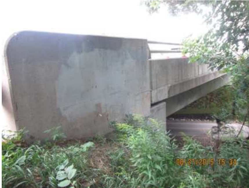
SOUTHEAST WINGWALL - AUG'15
