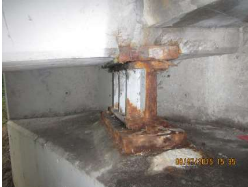
SOUTH ABUTMENT BEARING - AUG'15
