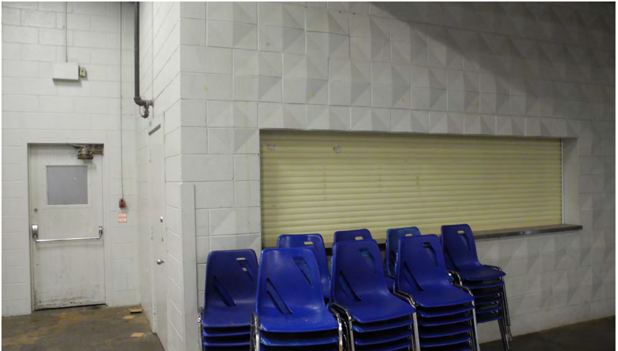
Figure 41 - Interior finishes on the Progress Building, including sculptural CMU blocks, and strong wooden door (CBCollective 2018).
