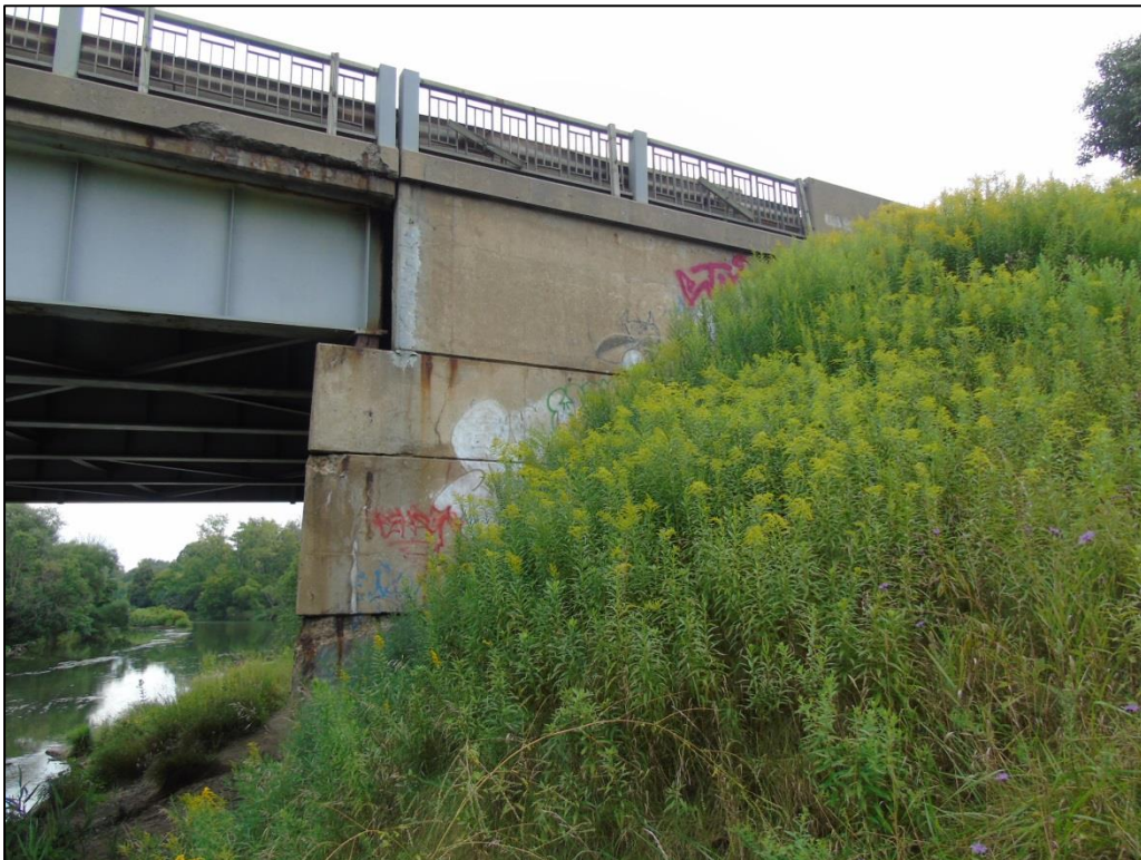
Photograph 17: View showing south abutment and earthen embankment
