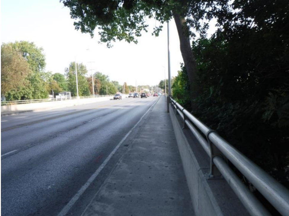
Plate 26: Sidewalk looking north along the east side of the bridge.
