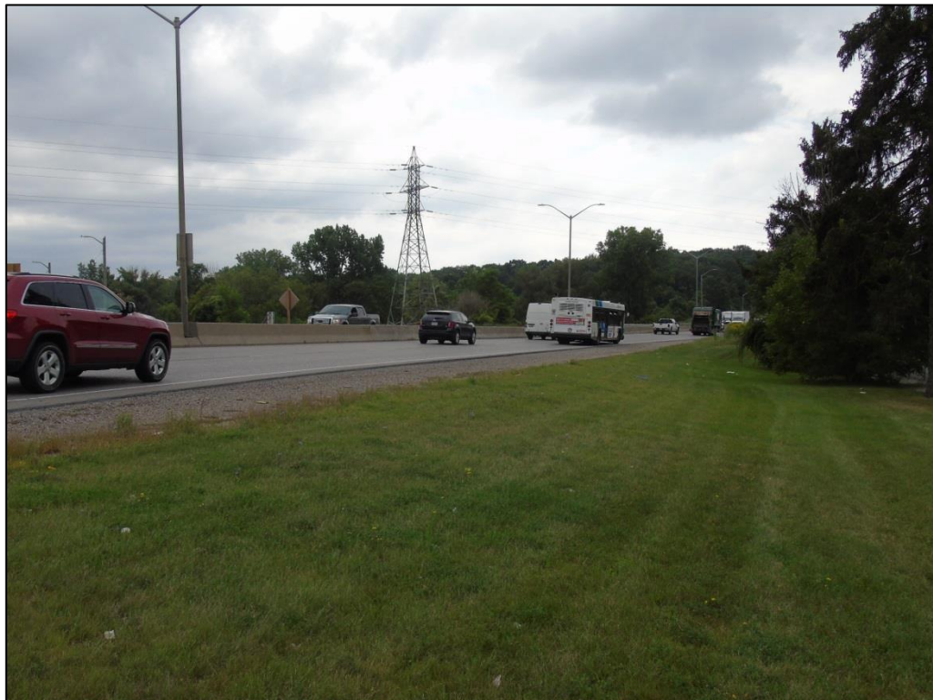
Photograph 13: View south of the bridge showing curve of Highbury Avenue as it approaches the bridge
