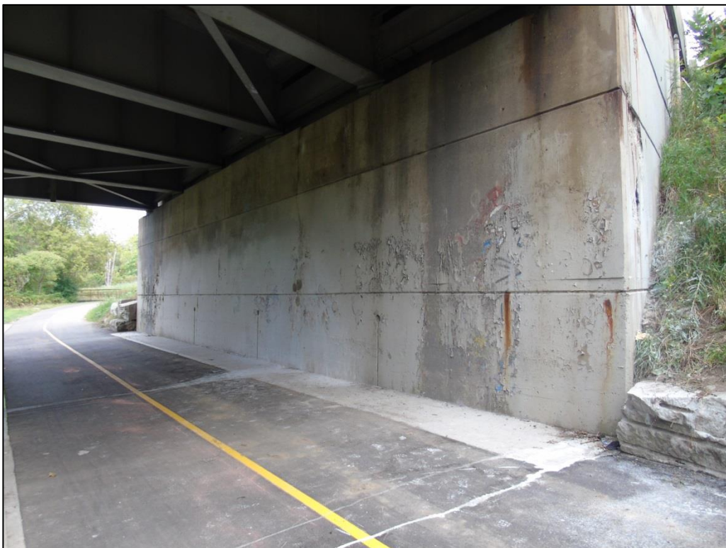
Photograph 15: View showing north abutment and proximity of Thames Valley Parkway
