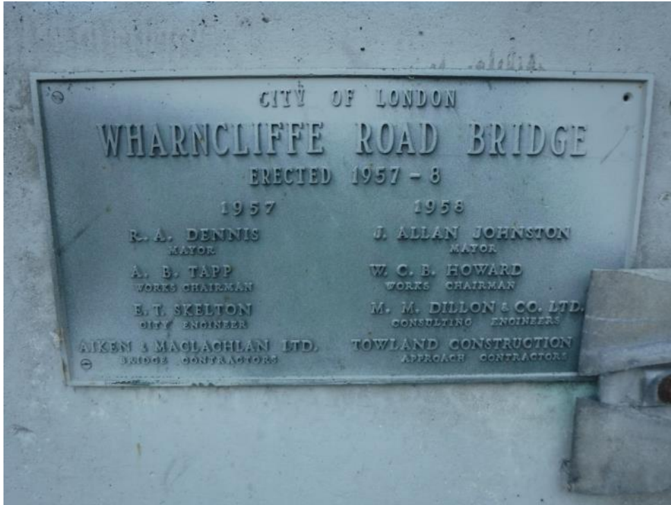
Plate 27: City of London bridge plaque, located on the southeast wingwall.
