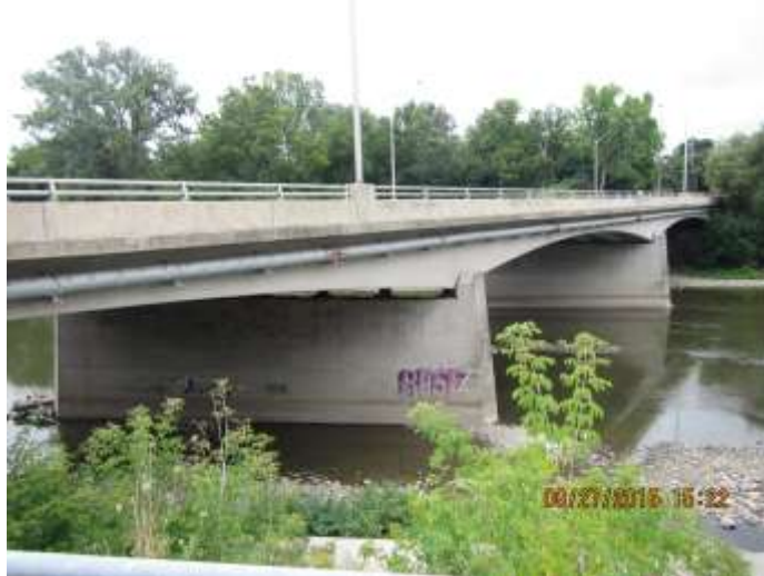
WEST ELEVATION LOOKING SOUTH - AUG'15
