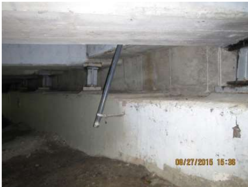
SOUTH ABUTMENT BEARINGS - AUG'15
