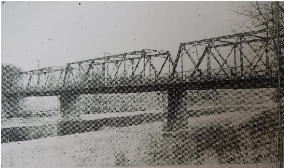
Figure 13: View of the first two lane Wharncliffe Road crossing over the Thames River
