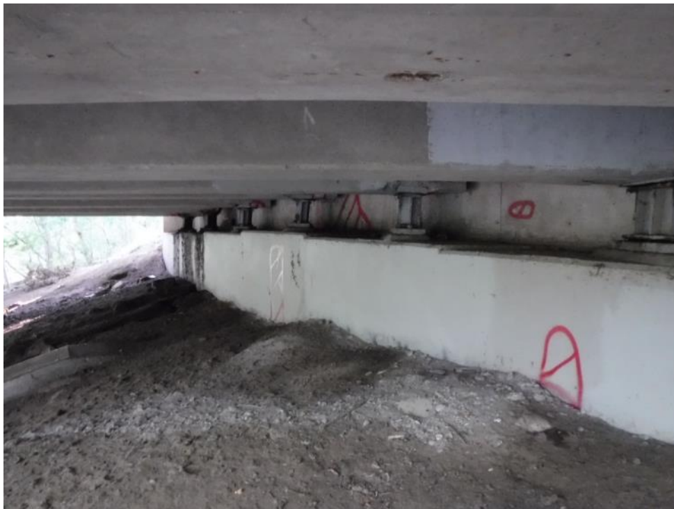
Plate 18: View of the south abutment and bearings.
