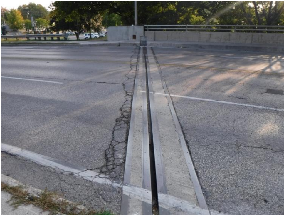
Plate 7: North expansion joint with view of the wingwall and the railing system.
