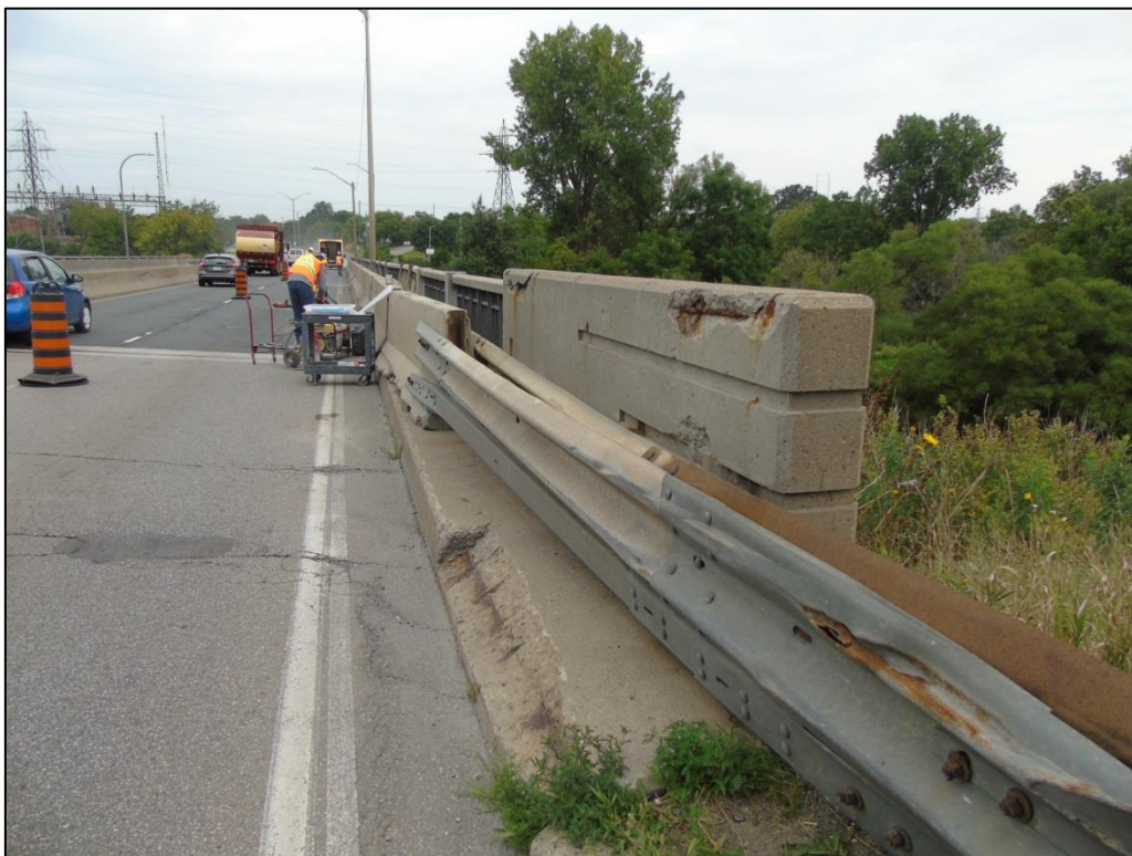
Photograph 21: View showing deck with asphalt wearing surface, concrete curbs, as well as temporary concrete barriers
