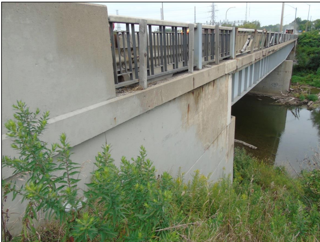
Photograph 23: Steel railing systems, not visible from roadway
