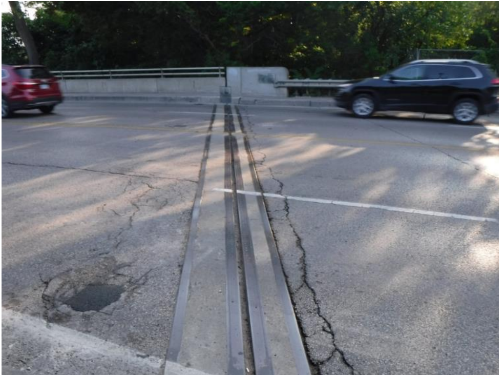
Plate 14: View of south expansion joint.
