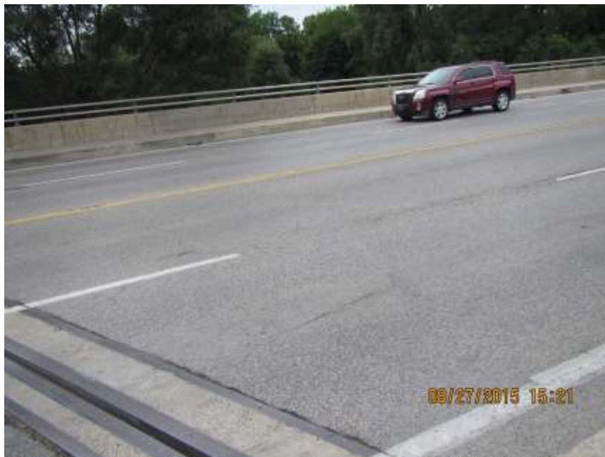
WEARING SURFACE LOOKING NORTH (2) - AUG'15
