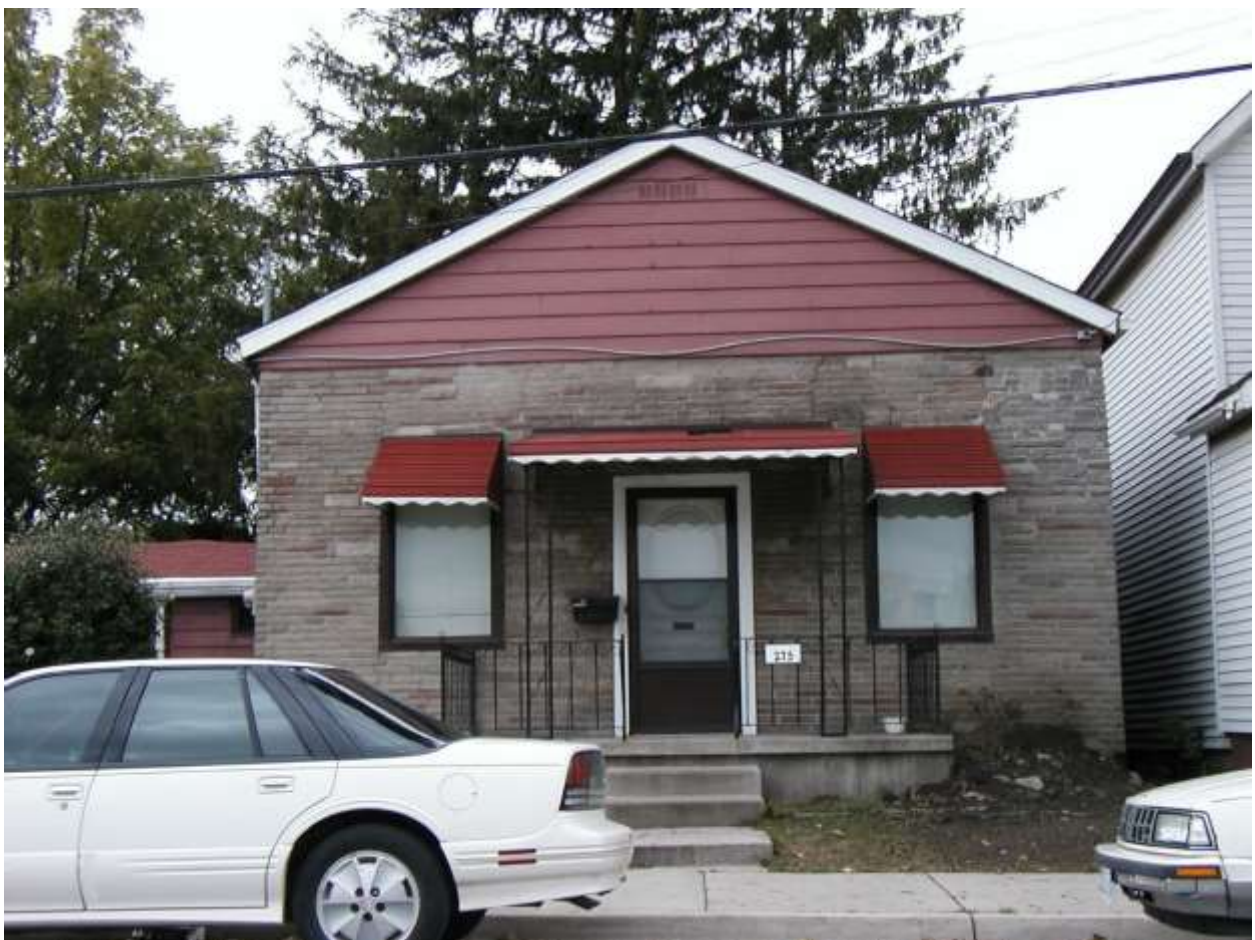
Image 2: Photograph of the building at 275 Thames Street in 2001, front facade
