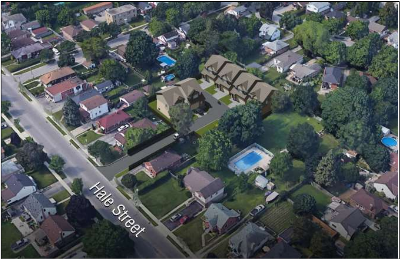
3D Google map view of the neighbourhood with massing model of the proposed development inserted into the image.
