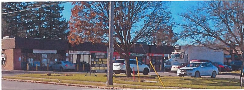
Single-storey plaza on the southwest corner
