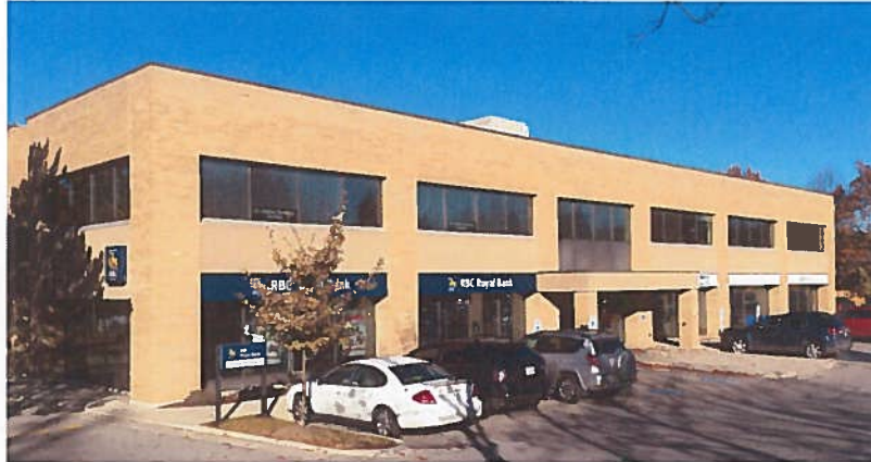
Two-storey office building on the southeast corner
