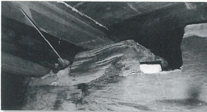
Image 20: Cut joist at rear of house.
