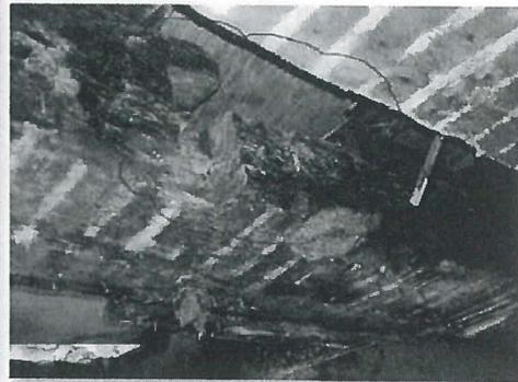
Image 21: Charred and cut joist at rear of house.
