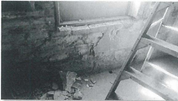
Image 26: Cracked Brick wall at Window
