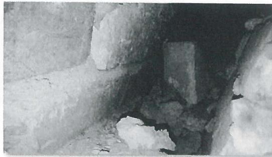
Image 4: Penetration in Exterior Brick Wall at base.
