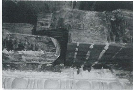
Image 15: Connection of Double Cantilever Joists
