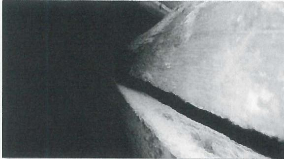
Image 18: Longitudinal Crack in wood joist
