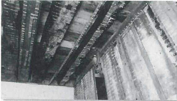
Image 24: Joist framing on brick Wall.
