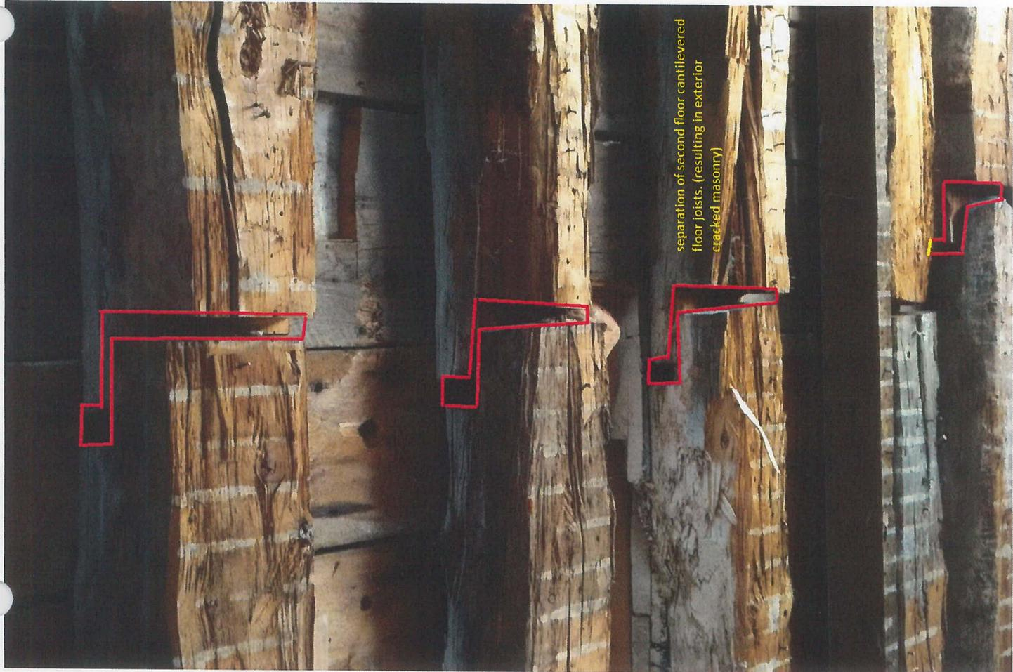
separation of second floor cantilevered floor joists. (resulting in exterior cracked masonry)
