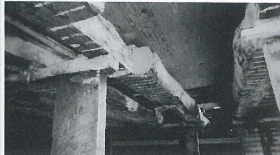
Image 17: Cut joist and stud top plate.
