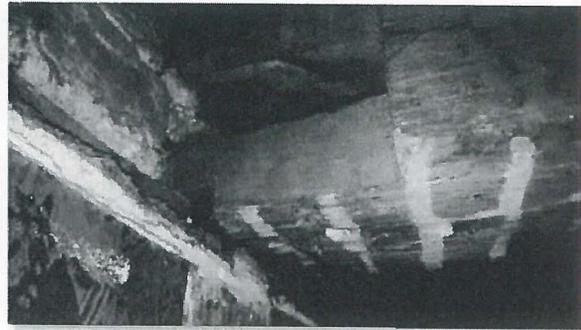
Image 27: Cut floor joists and minimal bearing at brick wall
