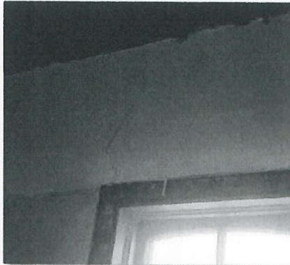
Image 29: Cracking at Window
