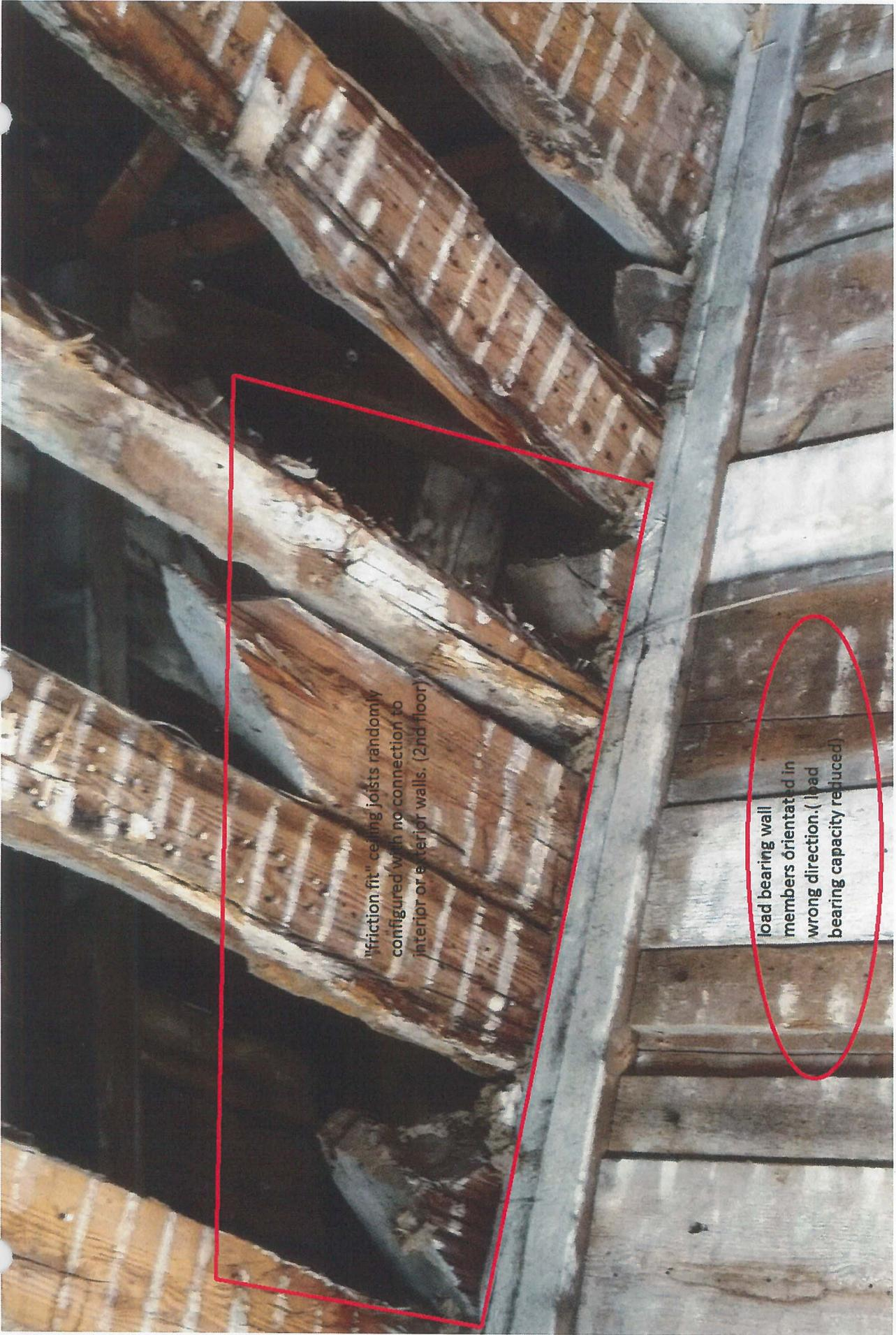
"friction fit" ceiling joists randomly configured with no connection to interior or exterior walls. (2nd floor)
