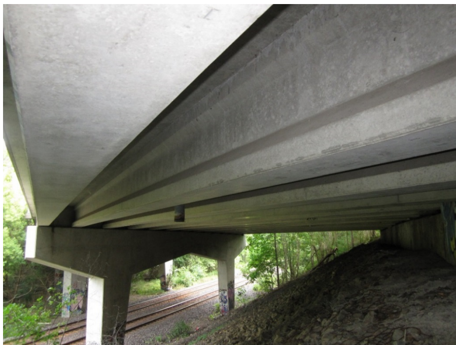
Plate 10: View looking northeast beneath the bridge showing the concrete I-beam girders
