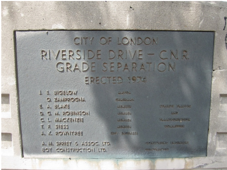
Plate 16: Detail view of the plaque at the northeast end post of the bridge
