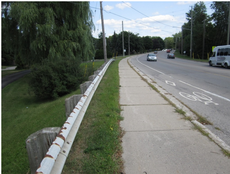
Plate 6: Looking east along Riverside Drive, showing curb, sidewalk, and bike lane.
