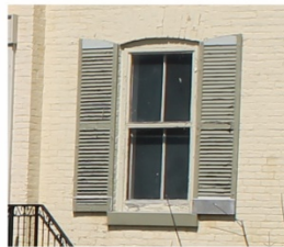
11. Wood shutters on the front facade
