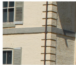
4. Brick exterior cladding (now painted) and brick detailing
