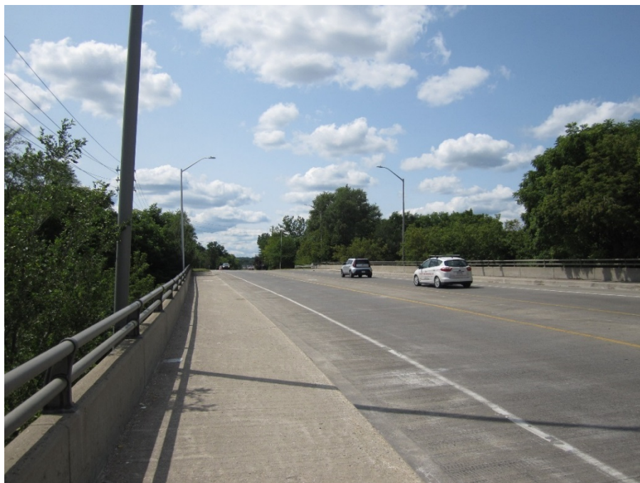
Plate 13: View looking southwest across the Riverside Bridge
