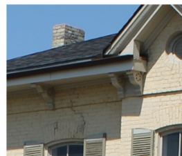
8. Paired and single wood brackets at the eaves
