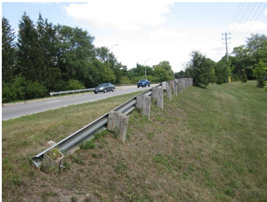
Plate 17: View looking northeast along the guide rail at the bridge approach
