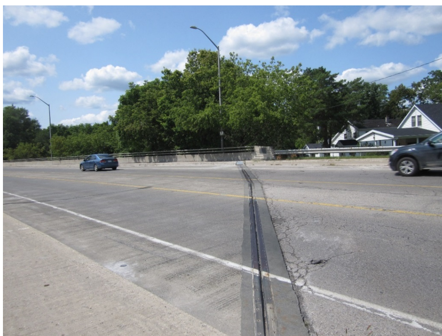
Plate 14: View looking northwest at the expansion joint of the Riverside Bridge
