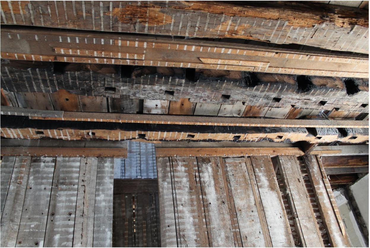
*Image 7: Photograph of the interior of the building at 172 Central Avenue; lath and plaster has been removed to reveal the structure of the building. Note the inconsistent charring of the timber members, which suggests that the wood was charred before its assemblage in this building (May 1, 2018).*
