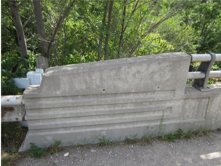
Plate 15: Detail view of the decorative concrete impression at the end railing post
