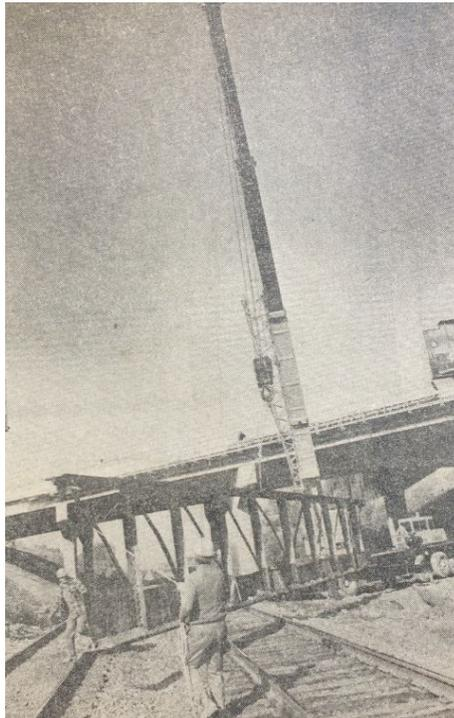
**Plate 3: Construction crews remove the steelwork of the old Riverside Bridge, October 1974
