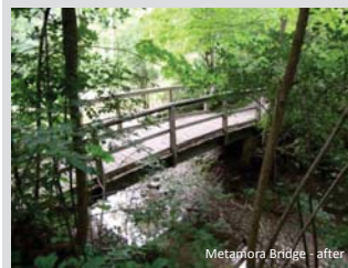
Metapora Bridge - after
