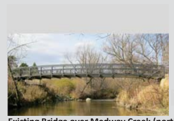
Existing Bridge over Medway Creek (north)
