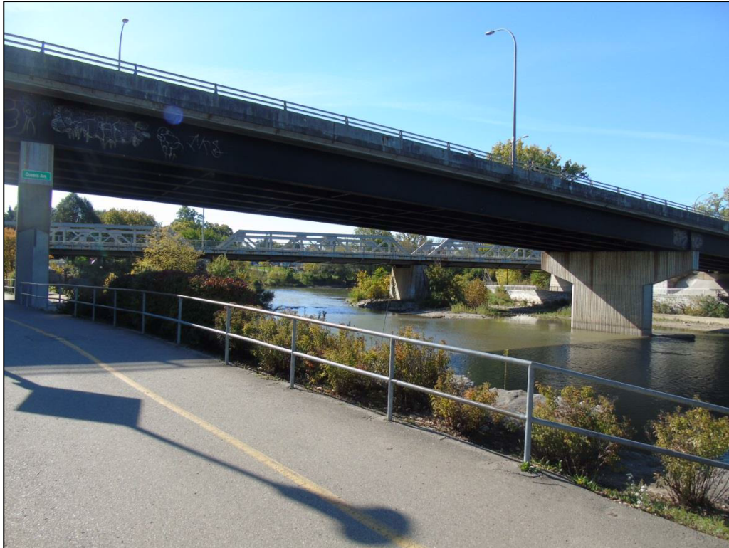
Image 12: View showing north side of The Queen's Bridge, showing Kensington Bridge located further south (downstream) of the river
