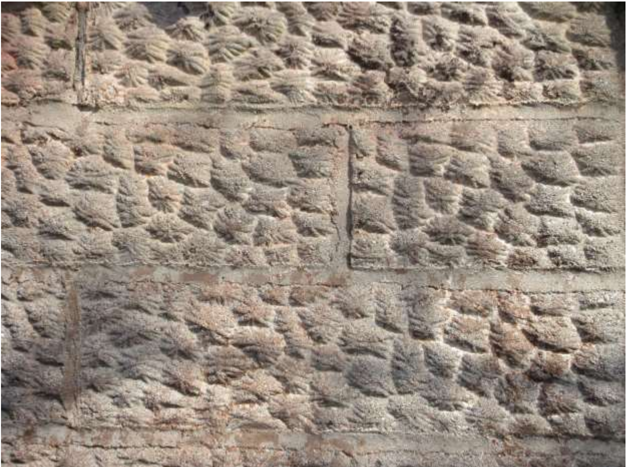
Image 14: Detail of the cast concrete block which comprises the base of the barns located at 2154 Richmond Street.
