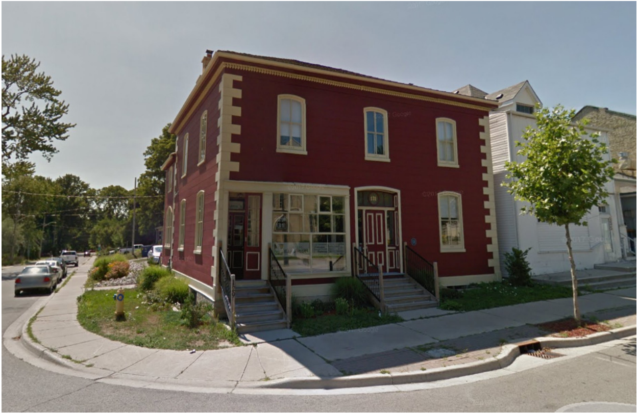
5. 129, 131 Wellington Street looking west
