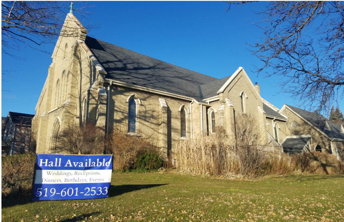
10. 138 Wellington Street looking east
