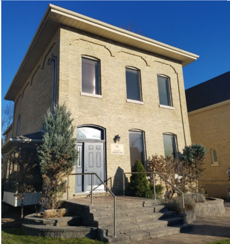
12. 152 Wellington Street looking east
