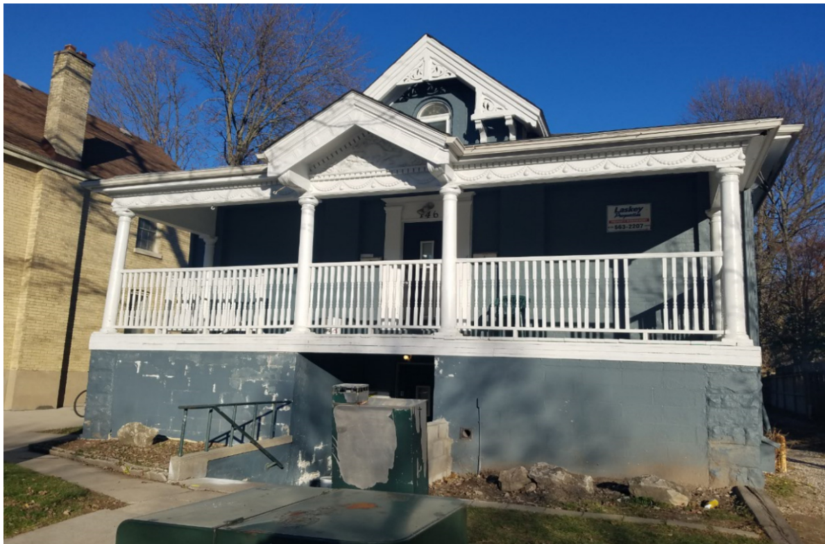
11. 146 Wellington Street looking east
