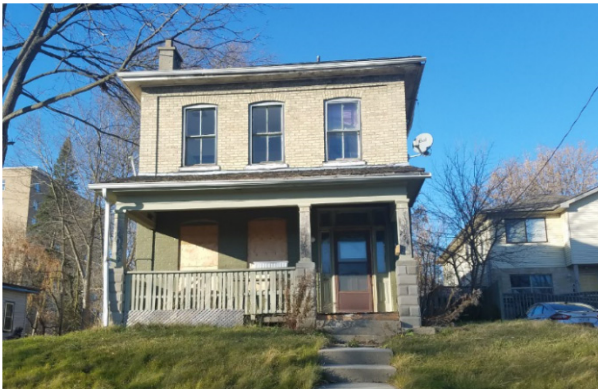
7. 254 Hill Street looking north
