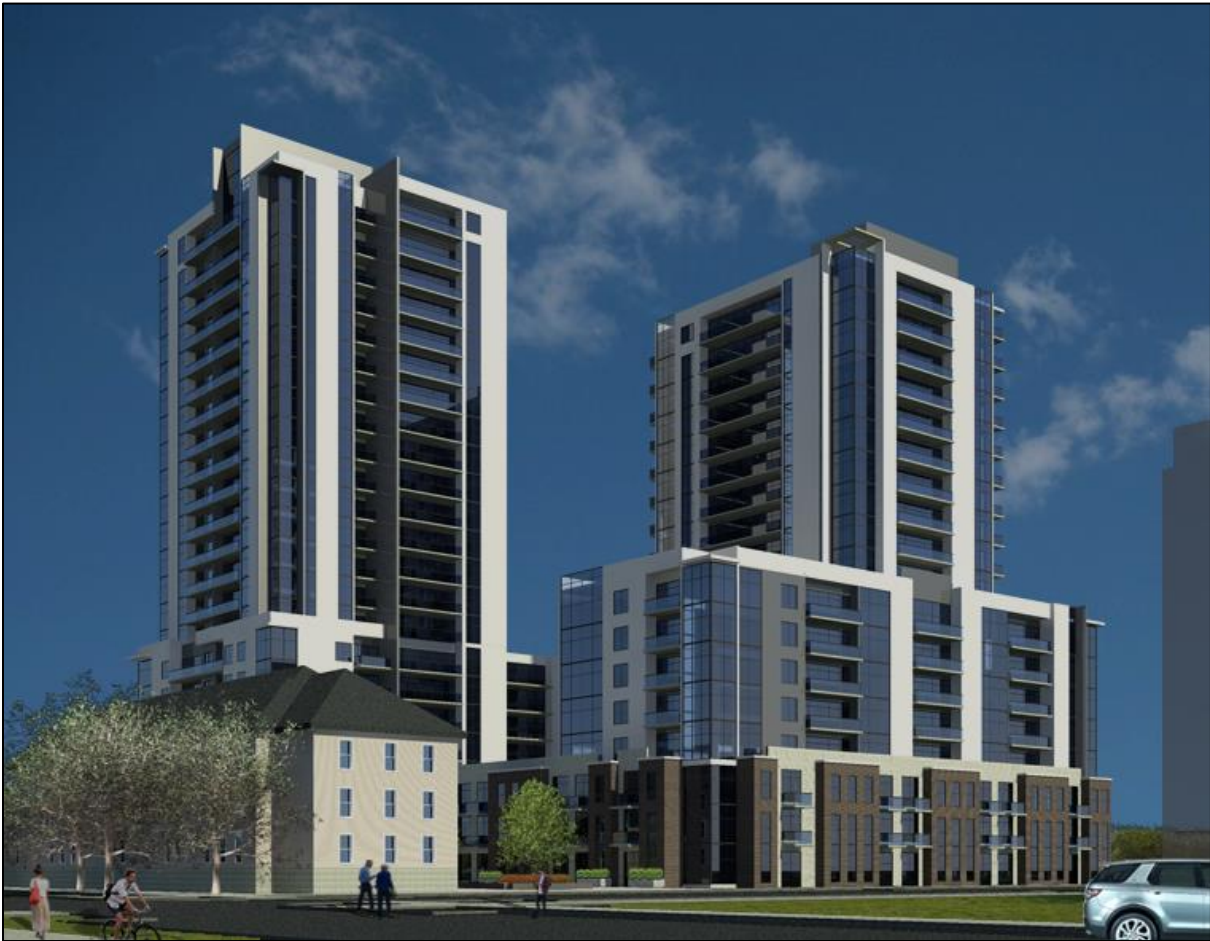
View from Northeast
