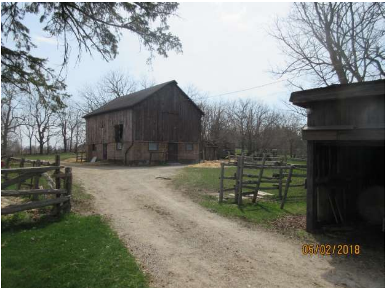
Image 10: View looking southeast from into the barnyard, showing the north barn located at 2154 Richmond Street. Note ruins of south barn in the distance beyond the north barn.
