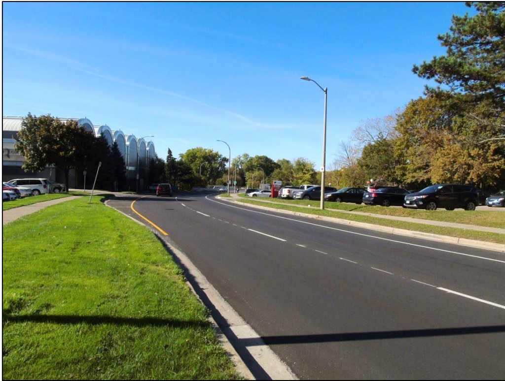
Image 16: Queens Avenue, showing curvature of the road at east approach to the bridge
