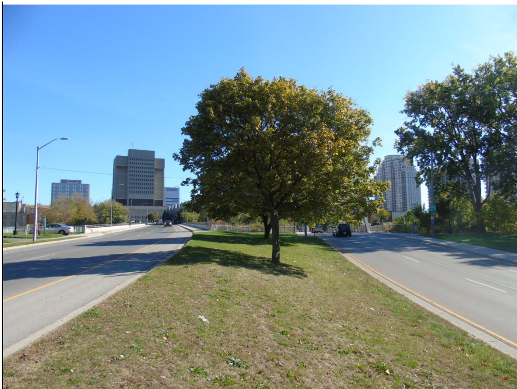
Image 15: View looking east showing west approach of The Queen's Bridge is on the left side. The photograph shows the grassed median where the Riverside Drive diverts at Queens Avenue and Dundas Street
