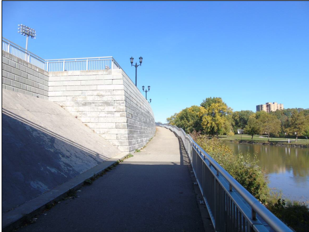
Image 20: View looking north from the west abutment, showing rise in grade to the TVP as part of the West London Dyke system
