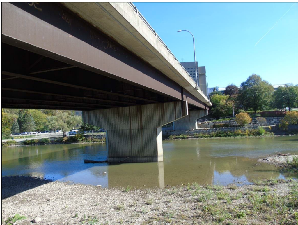
Image 19: View looking east across the river, showing piers supporting the steel girders
