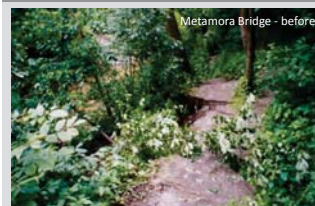
Metapora Bridge - before
