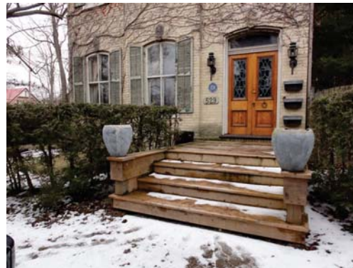
529 Princess Avenue after removal and construction of new porch (April 18, 2018)
