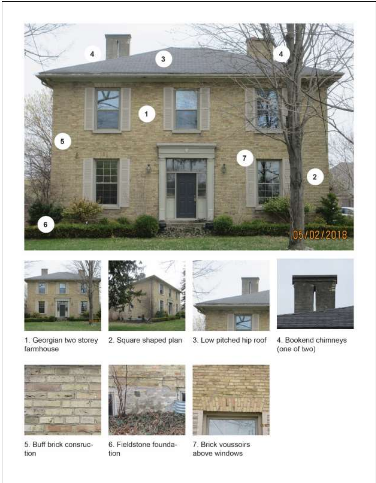
Figure 2: Heritage attributes of the property located at 2096 Wonderland Road North, as identified in the Statement of Cultural Heritage Value or Interest (see Appendix E).
