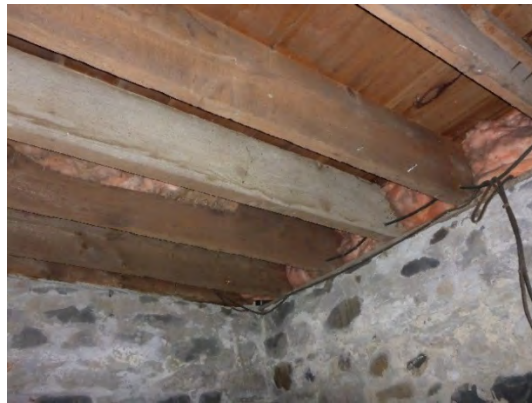
Plate 32: Basement with joists and foundation
