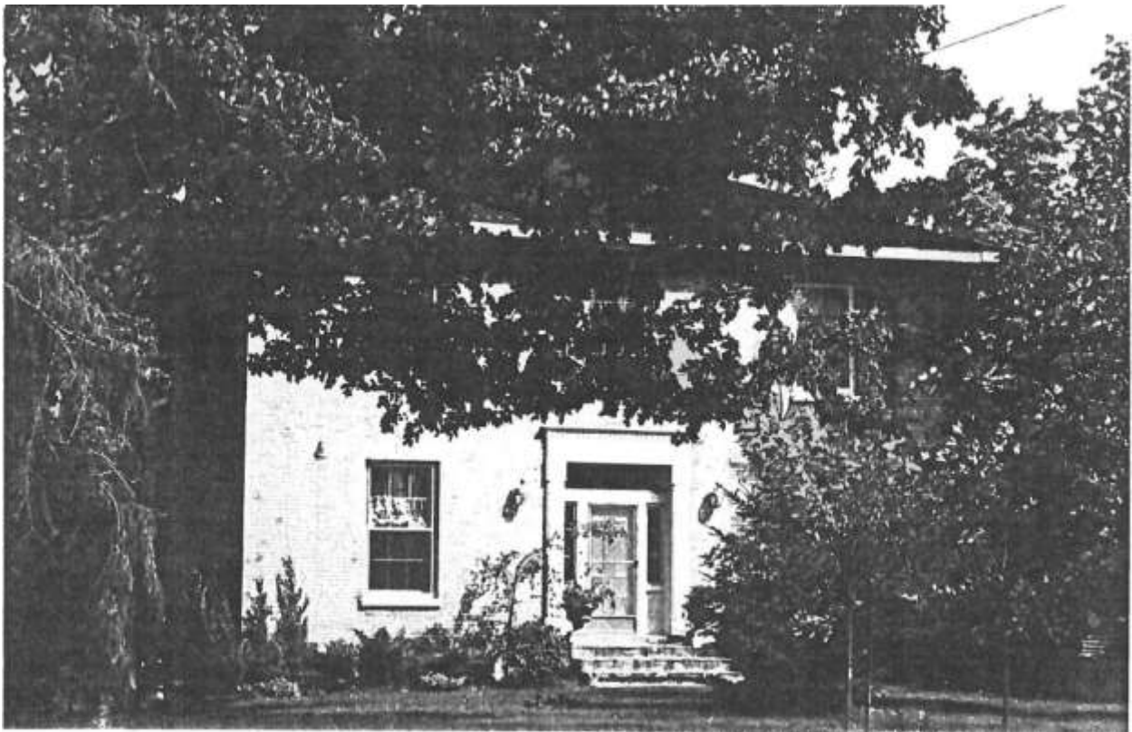
Image 4: View of the main (west) façade of the building located at 2096 Wonderland Road North (1993).
