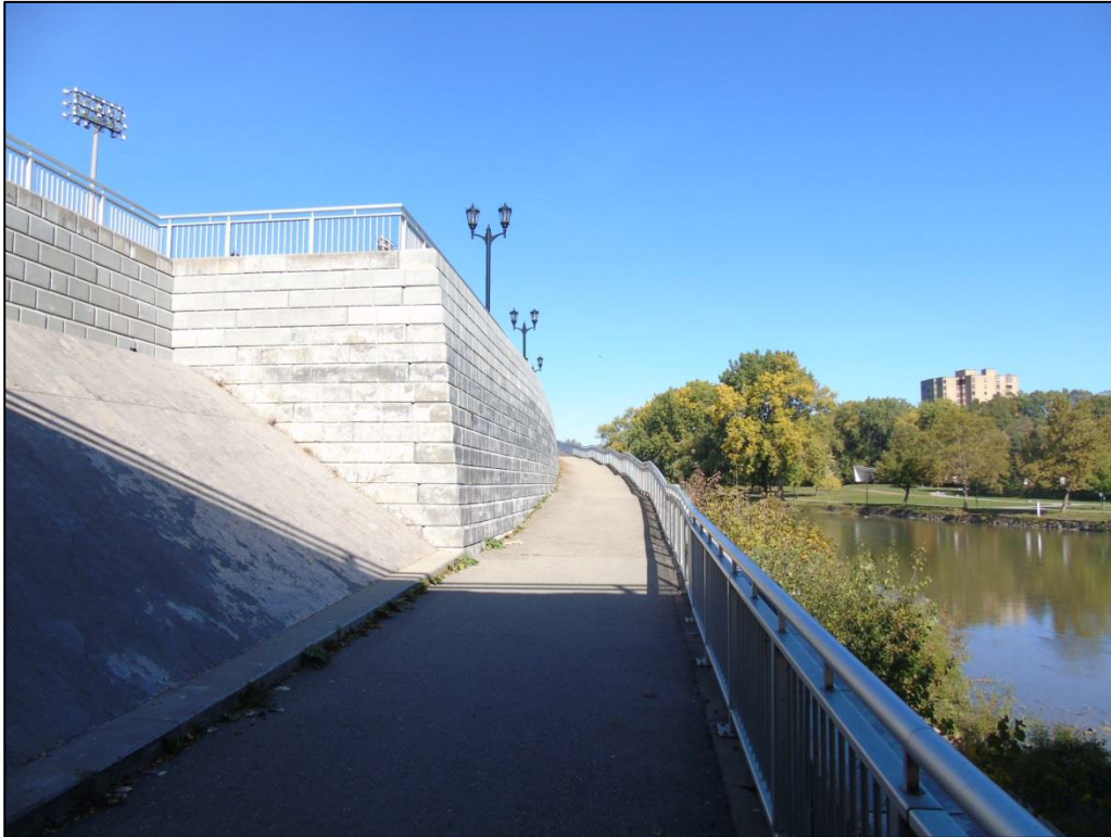
Image 20: View looking north from the west abutment, showing rise in grade to the TVP as part of the West London Dyke system
