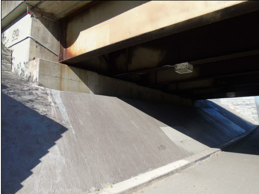
Image 18: West abutment, showing concrete revetment wall and TVP trail in the foreground
