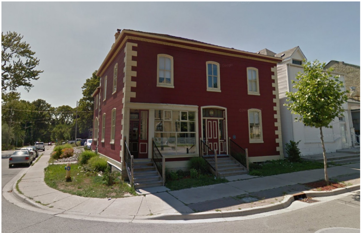
5. 129, 131 Wellington Street looking west
