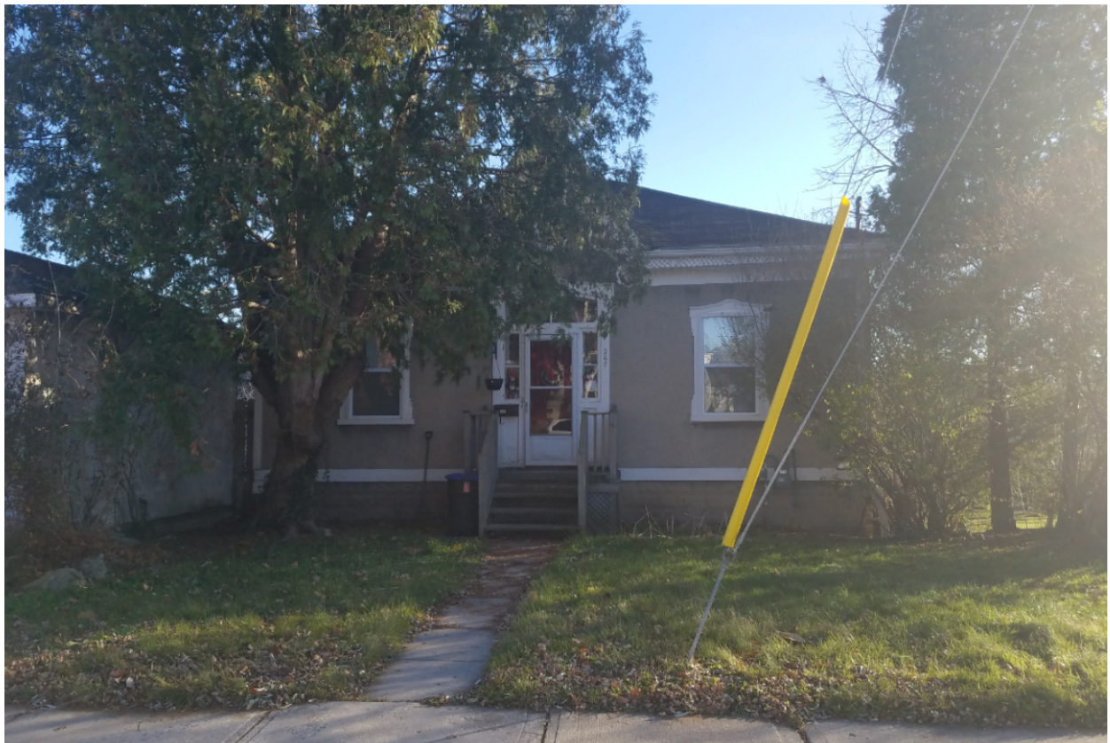
6. 267 Hill Street looking south
