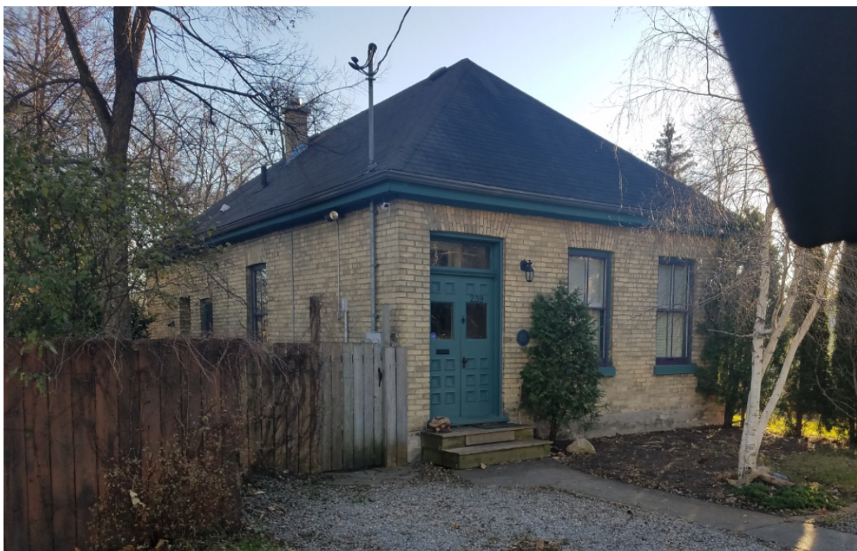
8. 239 Hill Street looking south
