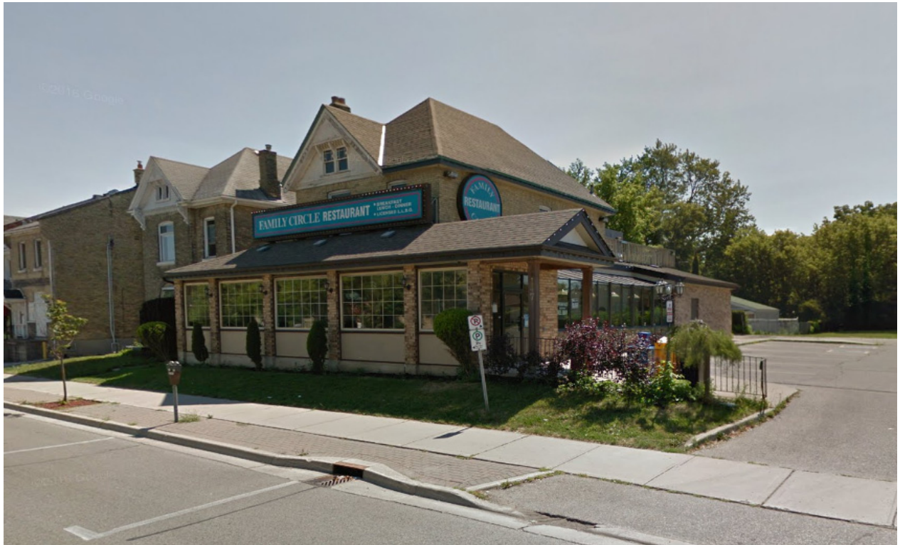
3. Family Circle restaurant in the south portion of the subject lands. To be demolished.
