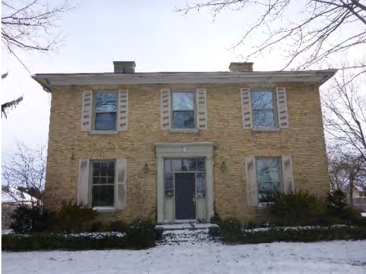
Plate 5: Front façade (western elevation)
