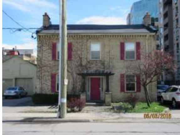
Image 16: Property at 177 Kent Street, built circa 1860. Note the urban context of this property, which translates into projecting firewalls at the gable ends of the building.
