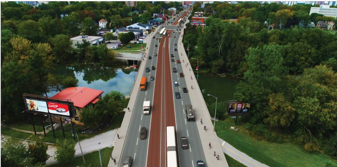
Clark's Bridge, Wellington Road (looking north)
