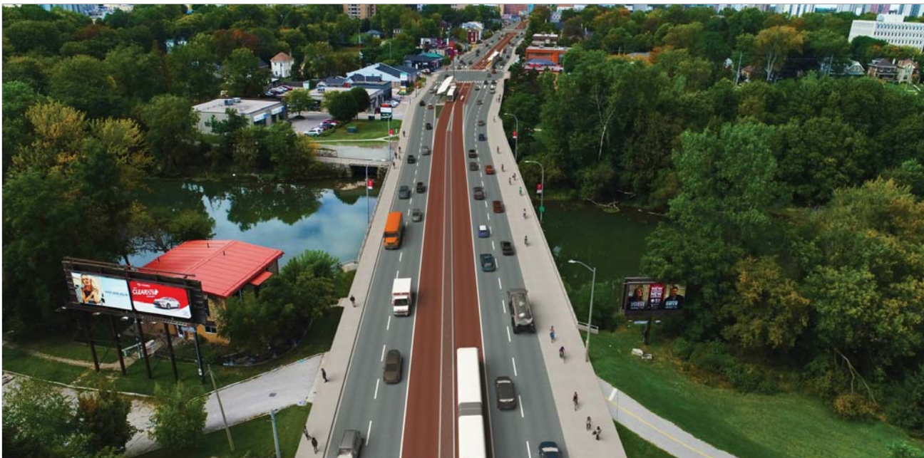
Clark's Bridge, Wellington Road (looking north)
