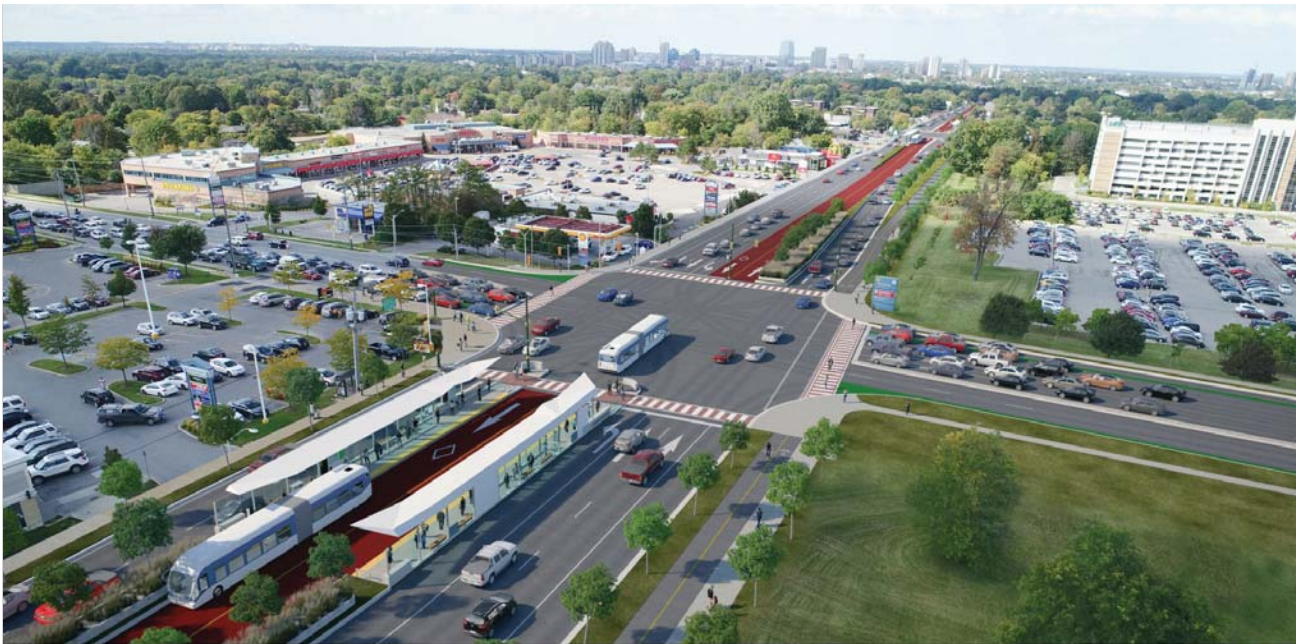
Wellington Road at Commissioners Road (looking north)
