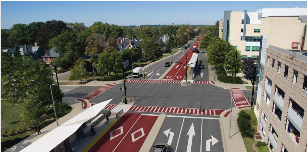
Richmond Street at Grosvenor Street (looking north)
