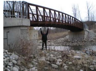
Note damage to bank caused by construction
