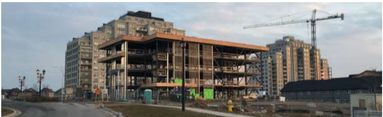
Figure 1: Photo of office building under construction on the site.
