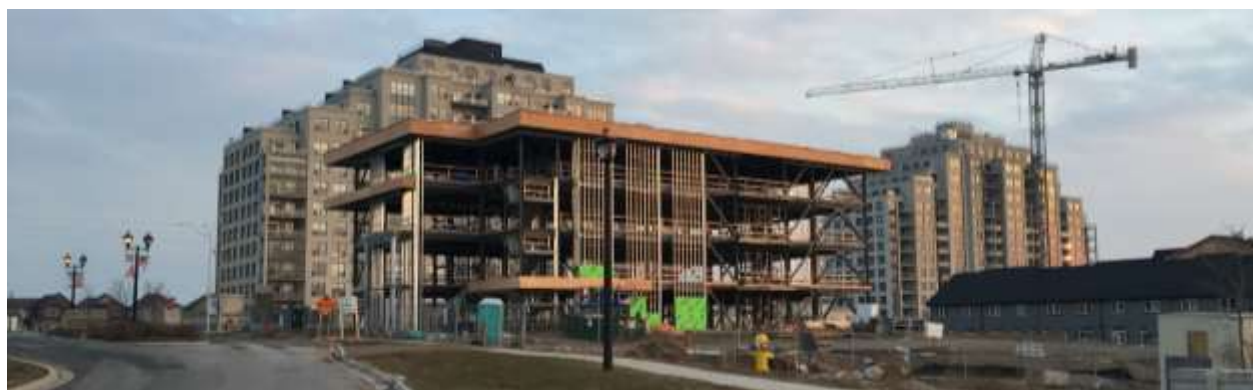
Figure 1: Photo of office building under construction on the site.
