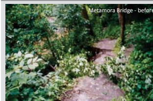
Metamora Bridge - before
