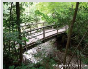
Metapora Bridge - after
