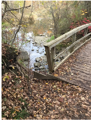
Approach to Metamora Bridge
