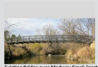
Existing Bridge over Medway Creek (north)
