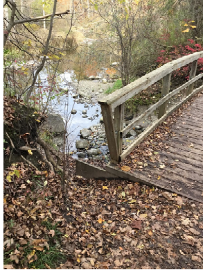
Approach to Metamora Bridge
