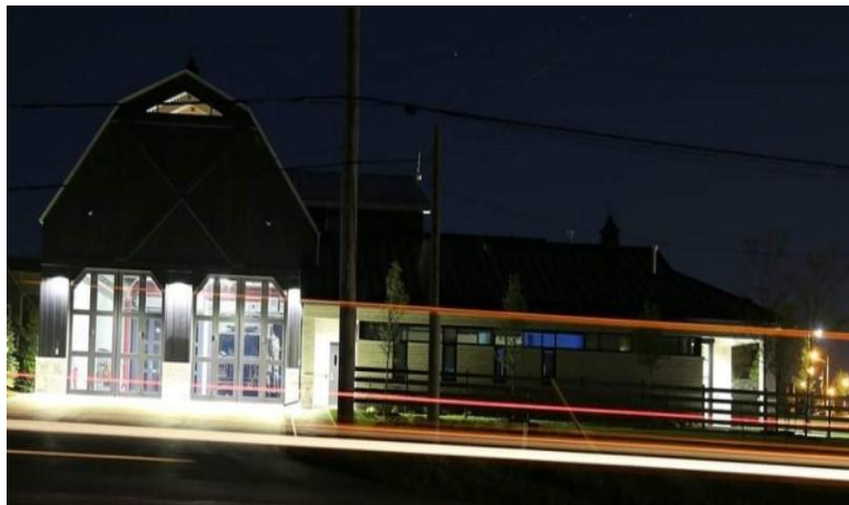
City of Oshawa Fire Station 6
