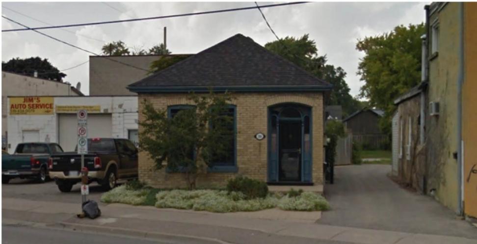
Figure B-8: 380 Hamilton Road, Priority 1 Listed Property – Built 1886 – Ontario Cottage
