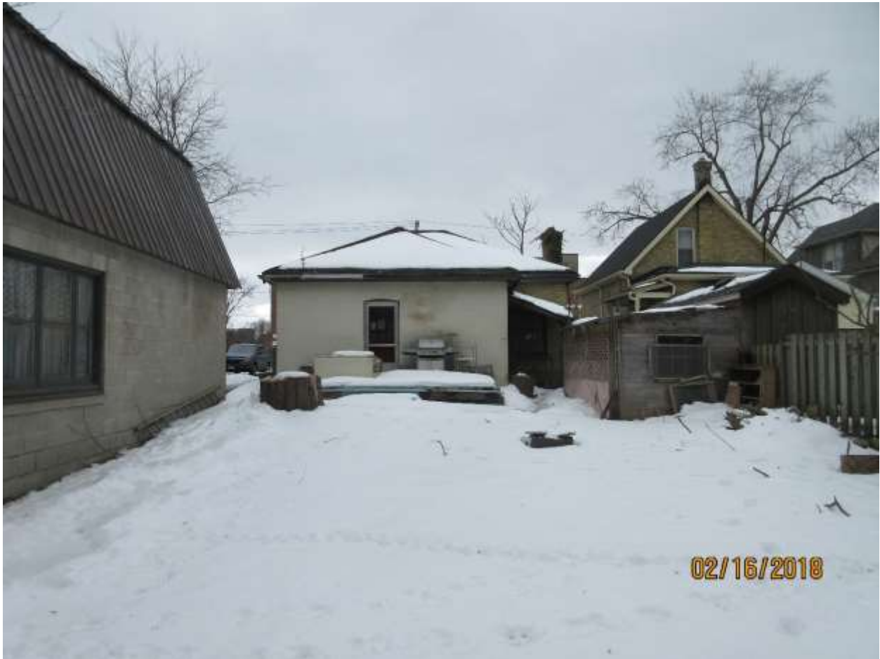
Image 5: View of rear (east) façade of the building located at 504 English Street.
