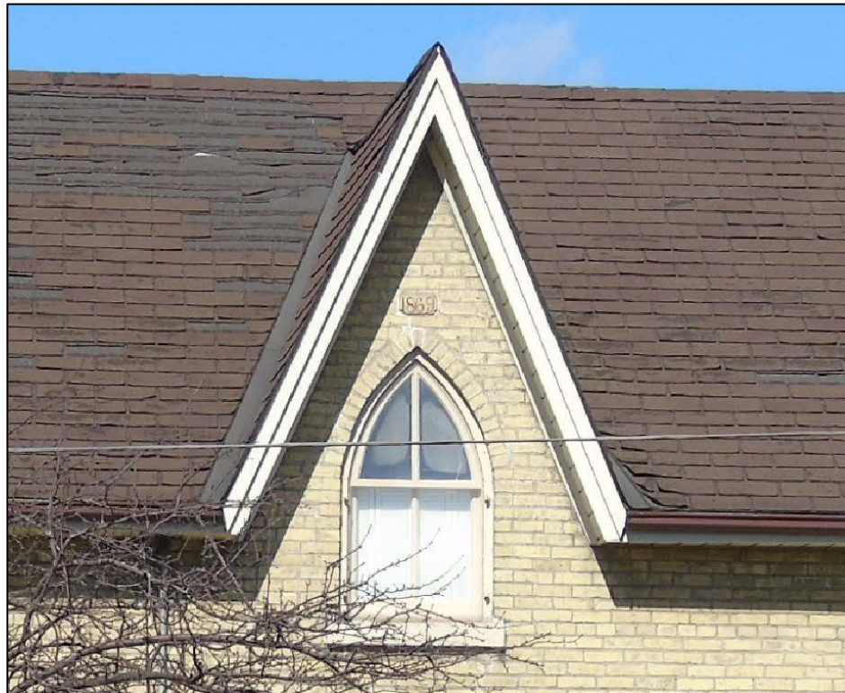
Image 4: Detail showing centre gable peak on front facade including cross gable, pointed arch window, and terra cotta date marking above the window (2018)
