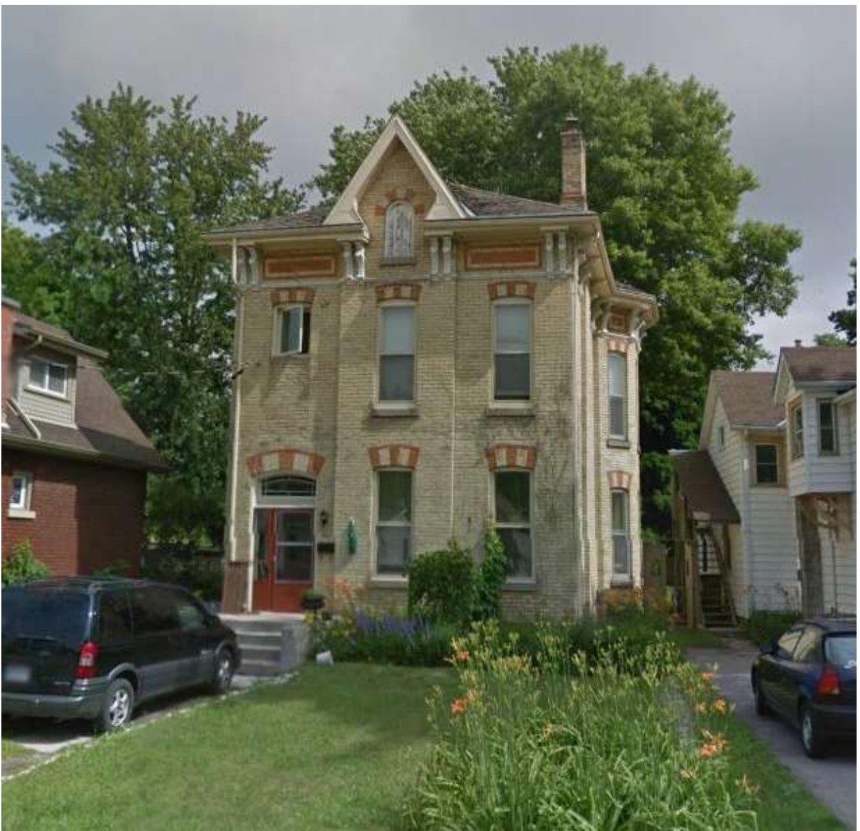
Image 6: View of (north) façade of the building located at 60 Euclid Avenue
