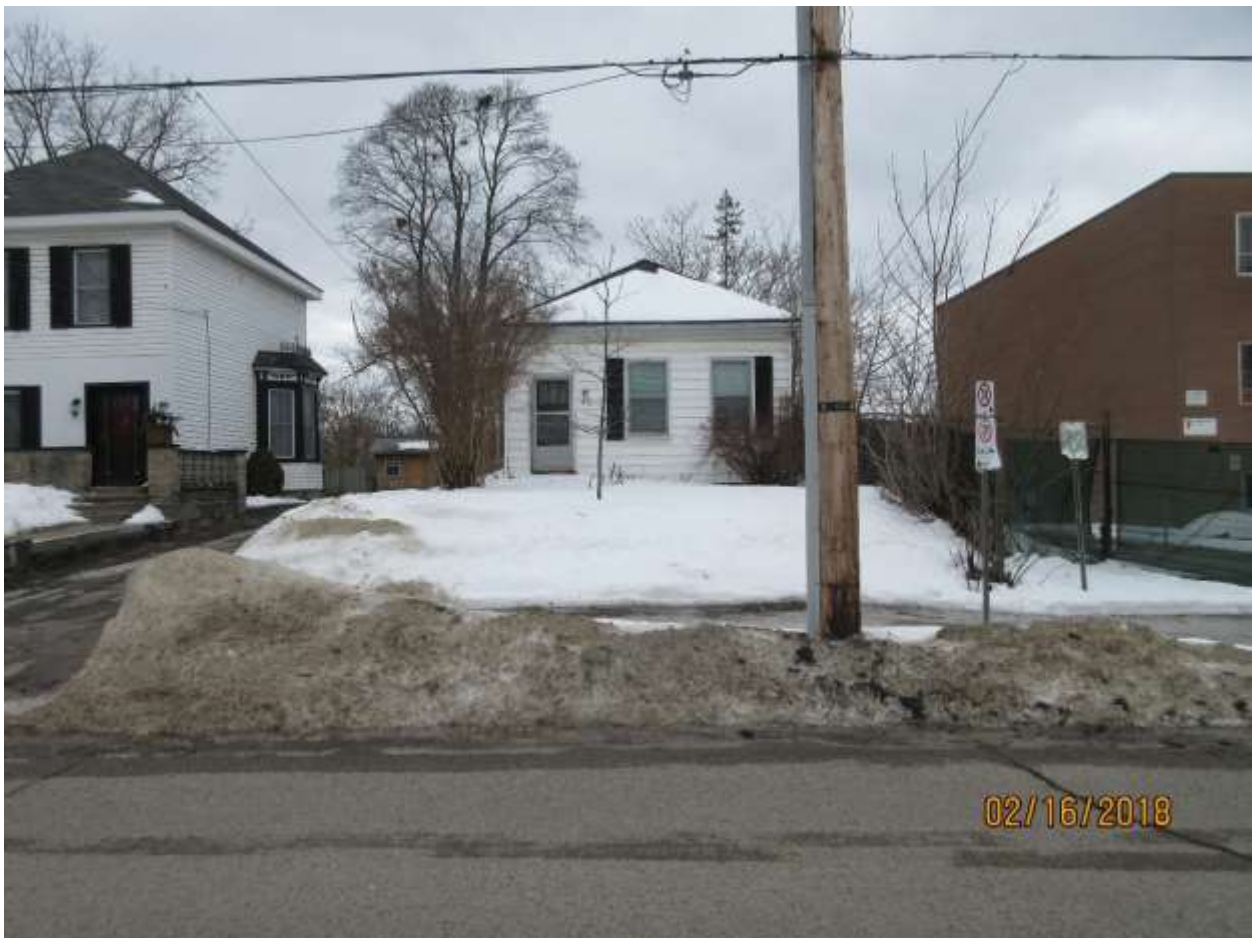
Image 1: View of front (east) façade of the building located at 491 English Street.
