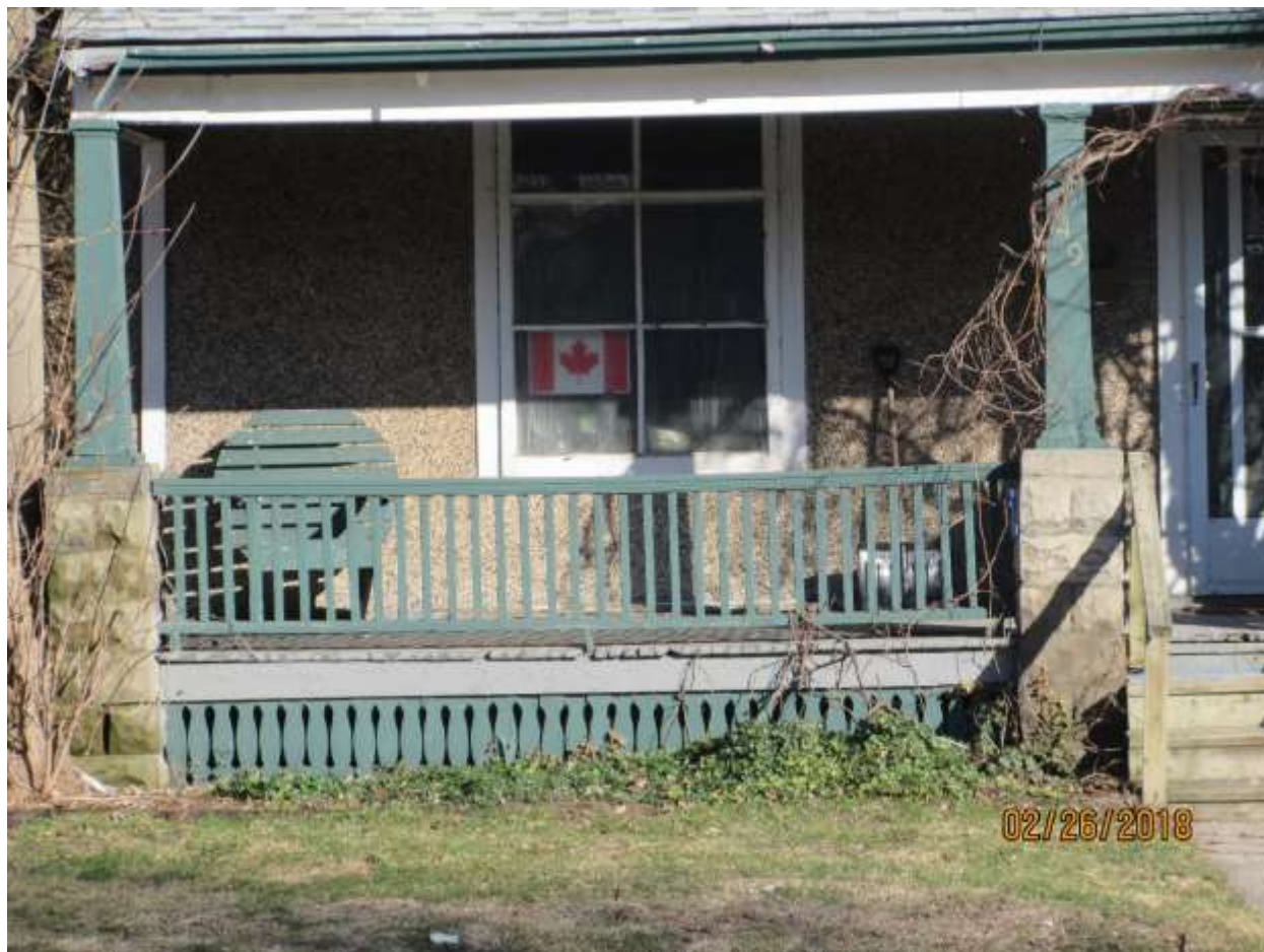
Image 9: Detail of porch balustrade at appropriate height with appropriate details and finish located at the building at 149 Wharncliffe Road North. Note the height of the balustrade is at the appropriate height to match the capstone of the cast concrete plinths.
