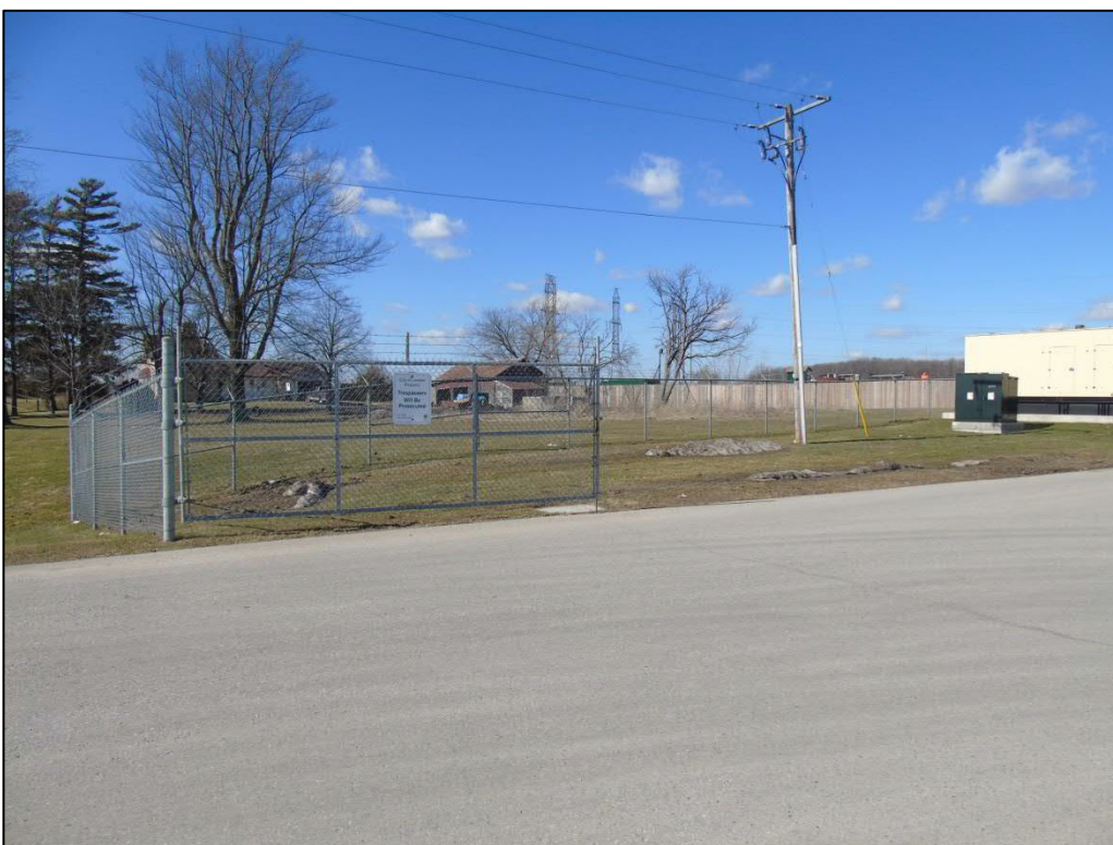
Image 10: View looking west from the Dingman Creek Pumping Station showing the view to the subject property and the location of the pumping station in relation to the historic farm property (2018)
