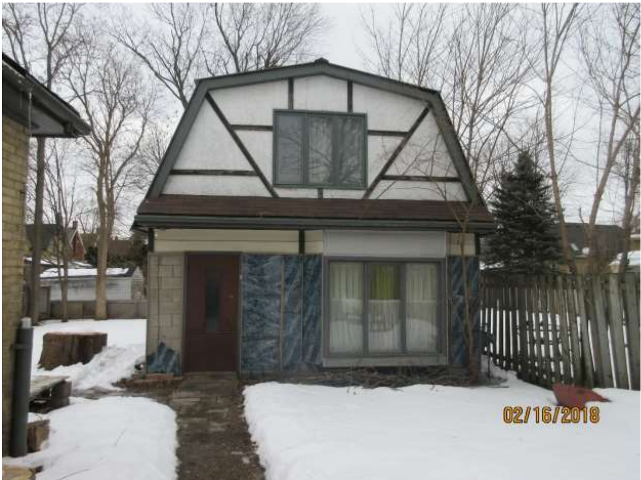
Image 6: Main (west) façade of the detached outbuilding located at 504 English Street.
