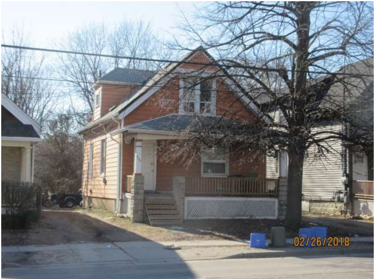
Image 4: View of the property located at 200 Wharncliffe Road North (February 26, 2018).
