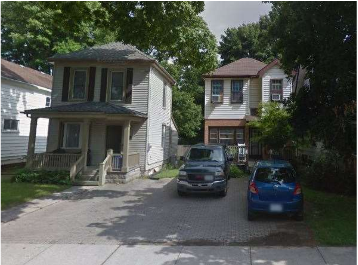
Image 5: View of (north) façades of the buildings located at 64 and 66 Euclid Avenue
