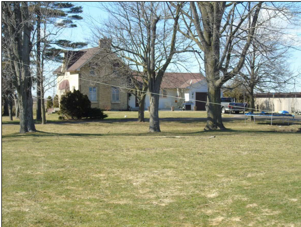
Image 5: View showing east side of the farmhouse. The historic portion of the dwelling is located on the left and the rear wing is a much newer addition (2018)
