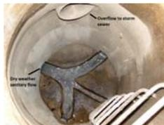
Sanitary sewer manhole with overflow to storm sewer
