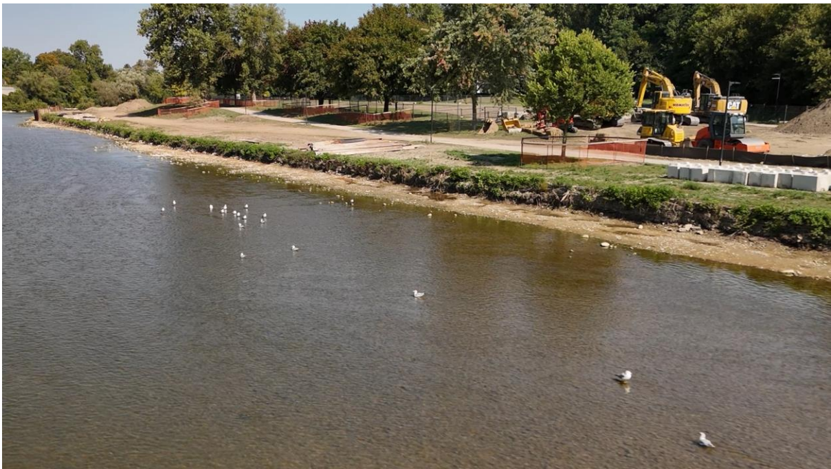
Above: Aerial view of Harris Park during construction in September 2024.
