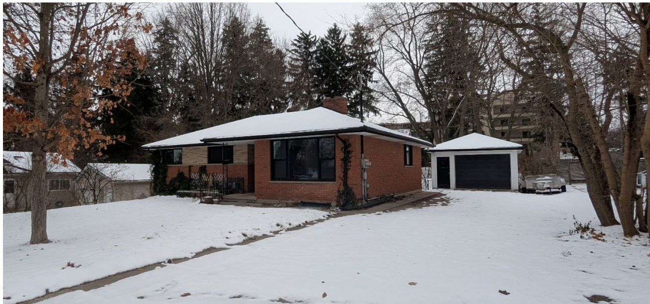
Figure 11: View of 402 North Street. (MHBC, 2025)
