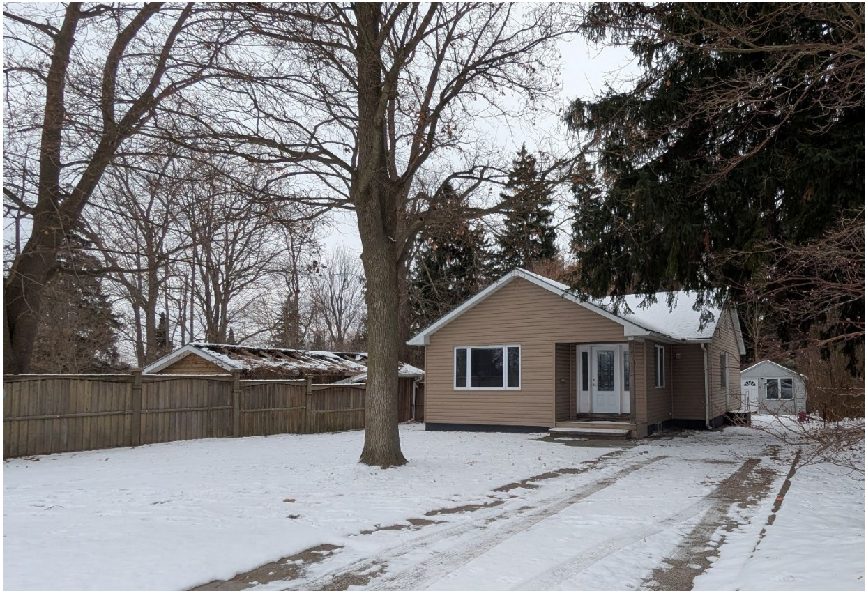
Figure 9: View of 396 North Street. (MHBC, 2025)
