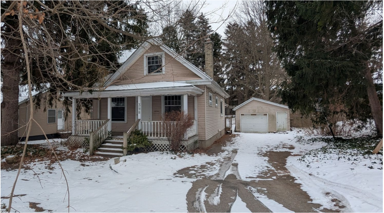
Figure 10: View of 398 North Street. (MHBC, 2025)
