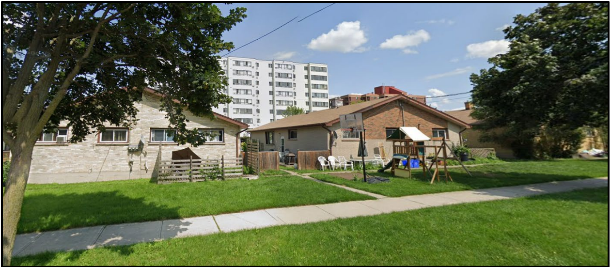
Figure 5 – Streetview of the subject lands.
