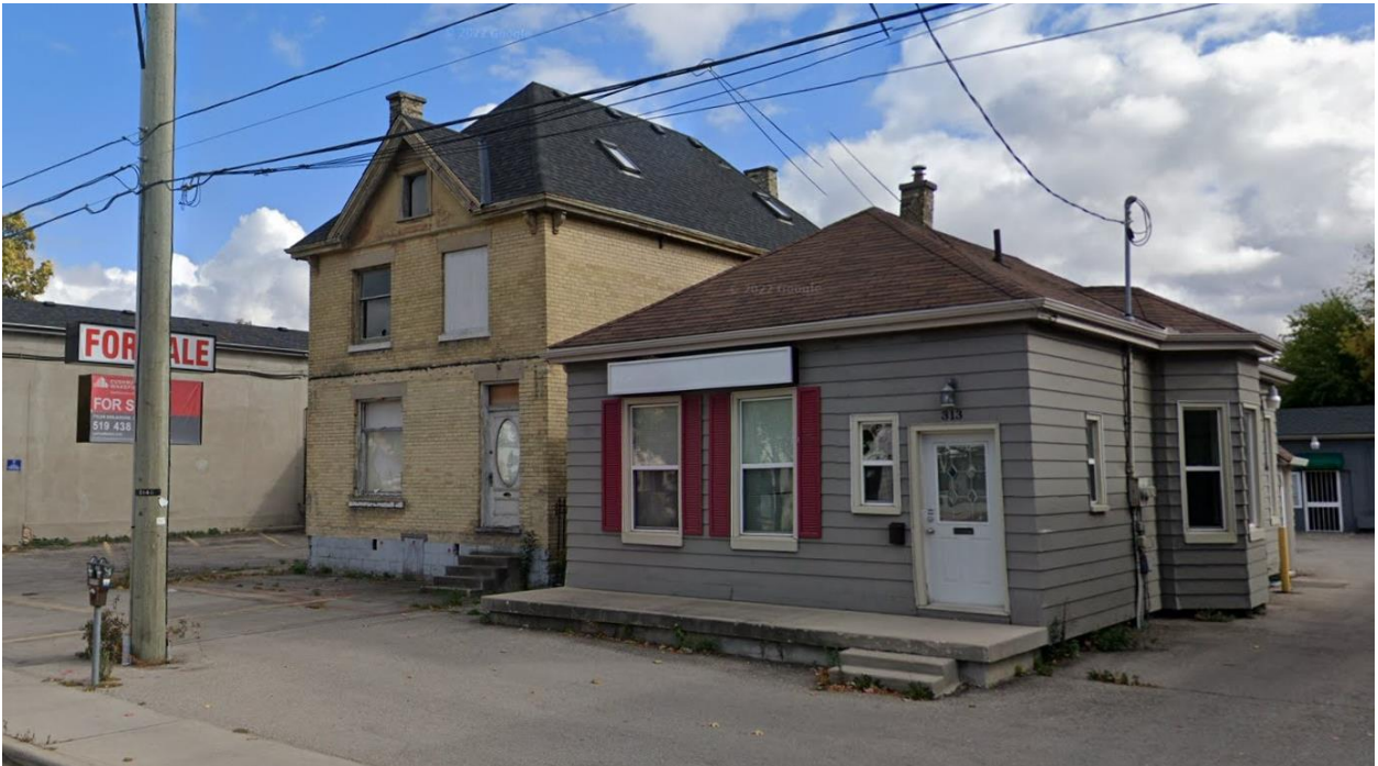
Figure 3 - Streetview of the 2 Vacant Commercial Buildings at 313 and 317 Horton Street East
