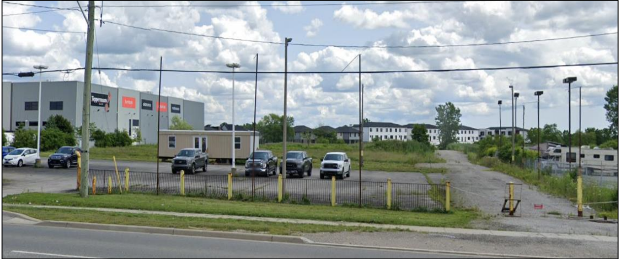
Figure 3 - Streetview of 1210 Wharncliffe Road South (view looking southeast)
