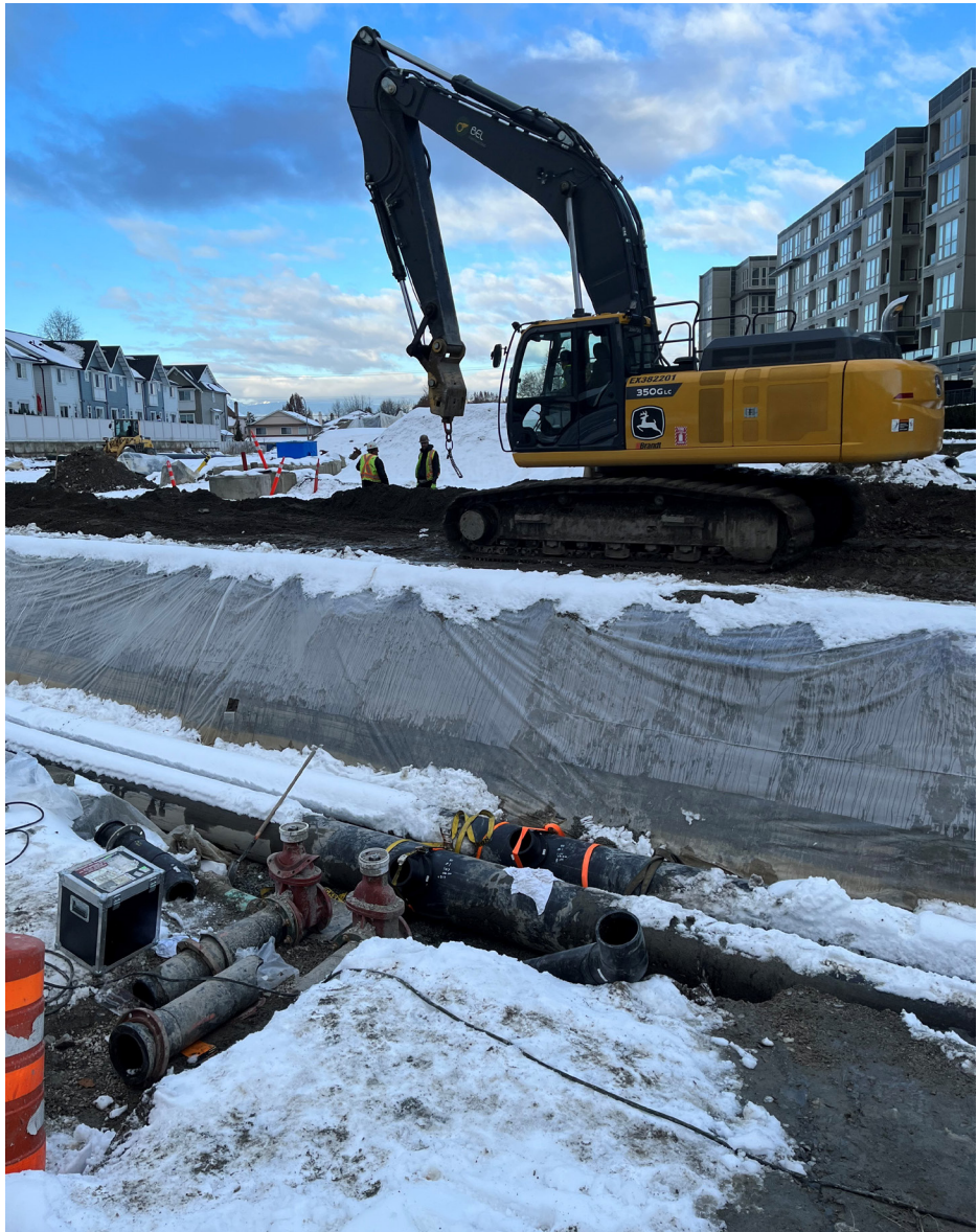
Implementing distribution piping in the ADEU.
