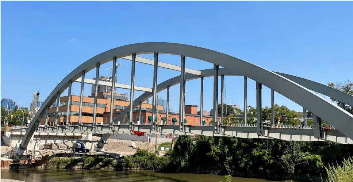
Above: A view of the new steel arches, which were lifted in place in the summer of 2023.
