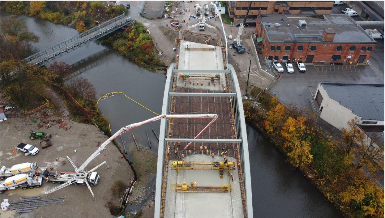
Above: An aerial view of the concrete pouring for the new bridge deck.
