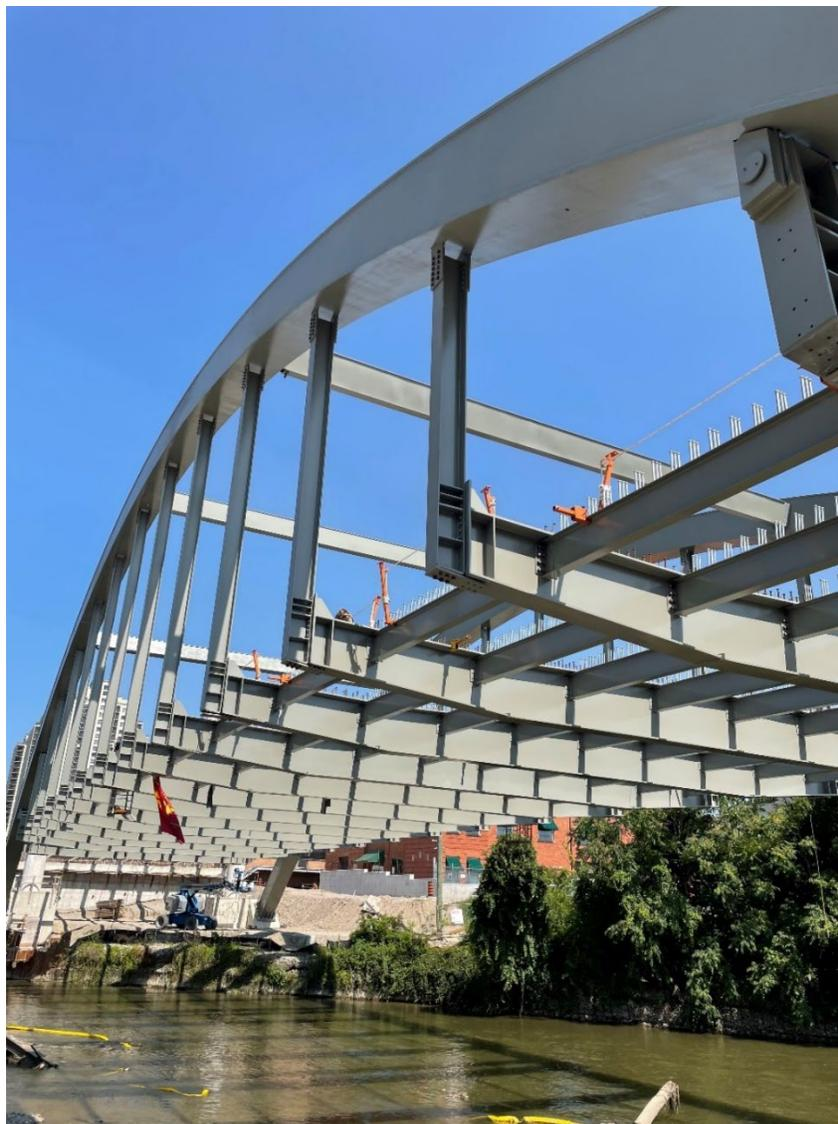
Above: A photo of the new bridge floor joist, hangers, stringers, and arch cross beams work on the concrete deck formwork, including an elaborate grid of steel rebar was completed in the fall of 2023. In addition to replacing the bridge structure, the Victoria Bridge reconstruction project includes intersection improvements at the Horton and Ridout Street intersection to add new traffic signals, bike lanes and asphalt.
