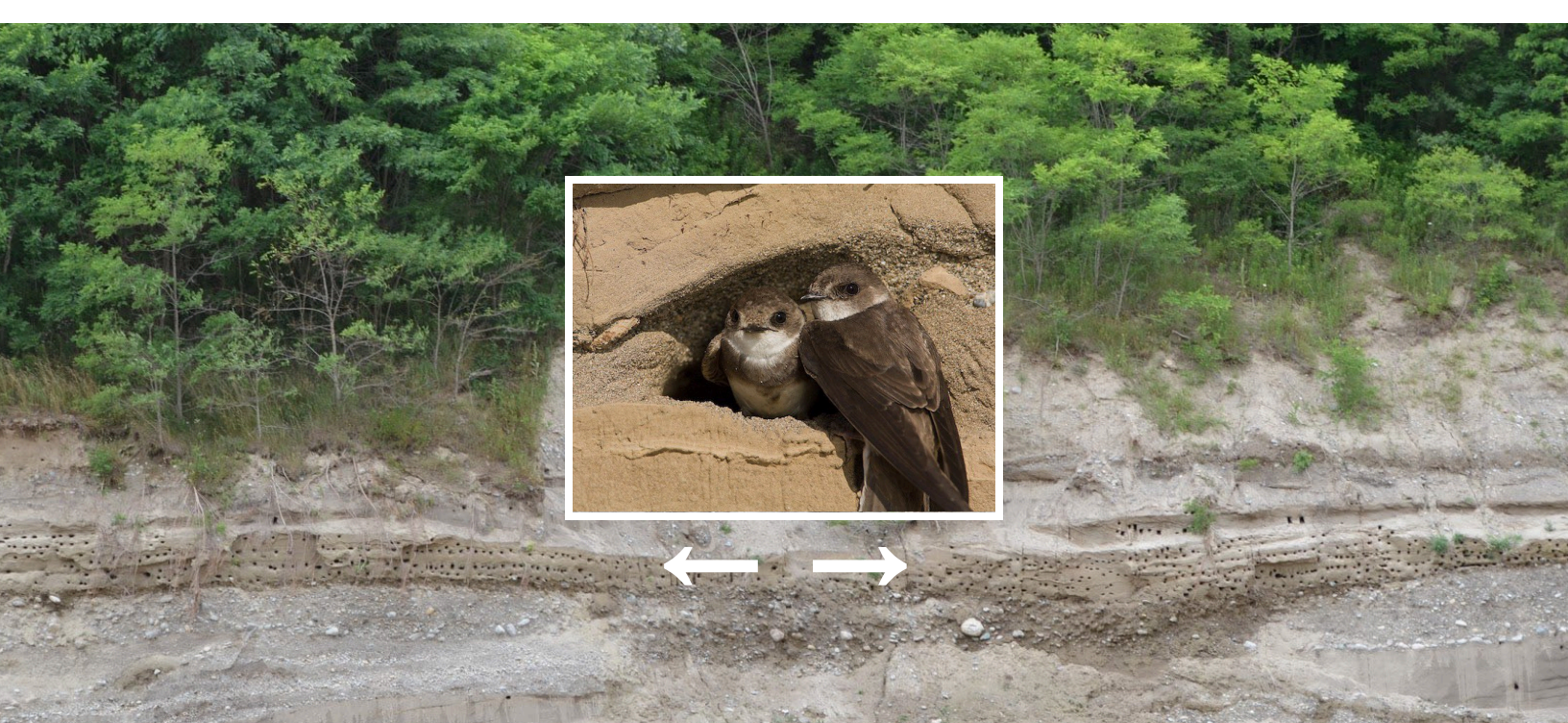
A portion of the Byron gravel pit Bank Swallow colony on the west bank.
