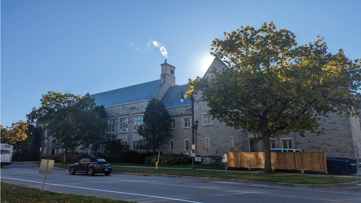
Photos 31 & 32: (above) View of Medway Hall north (front) elevation looking south-west; (below) View of north (front) elevation of Medway Hall looking south-east (MHBC, 2023).
