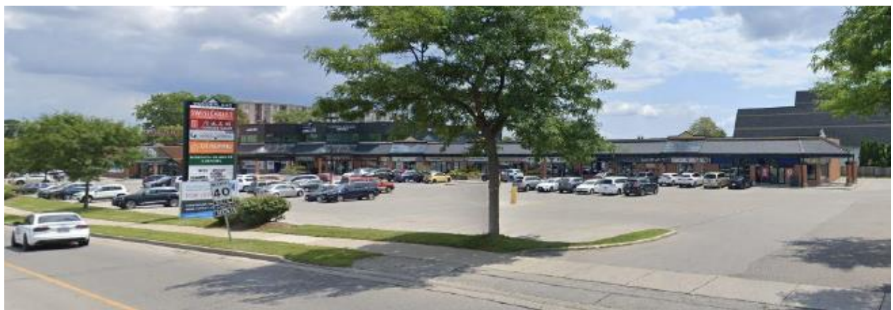
Figure 2 - Streetview of 735 Wonderland Rd N (view looking northwest from Beaverbrook Ave)
