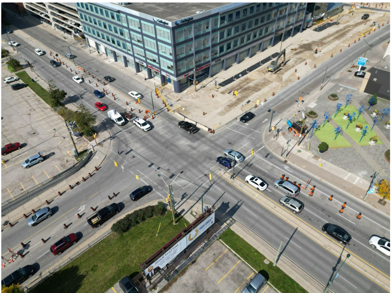
Above: Aerial view of the construction site at Wellington Street and York Street.
