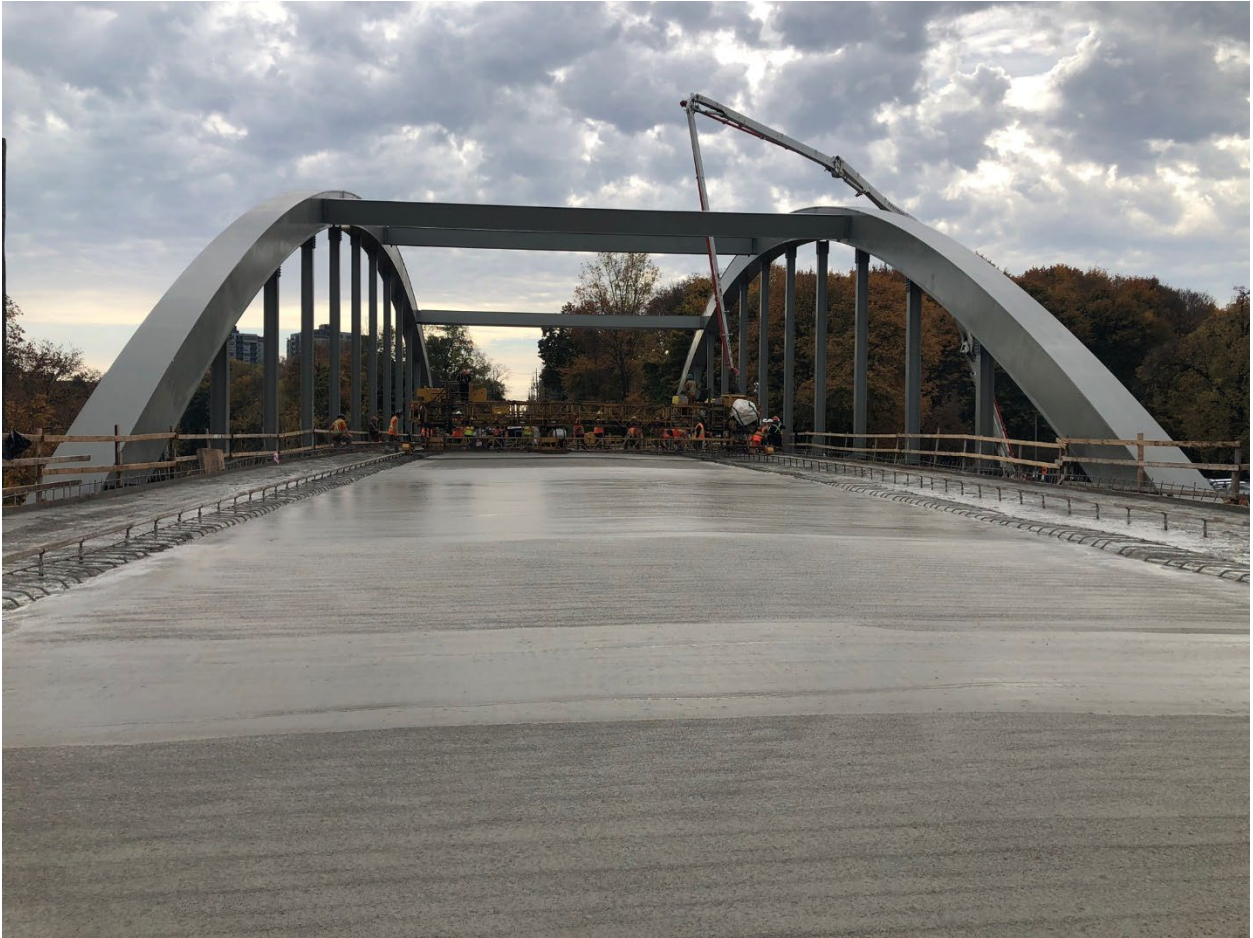
Above: Crews pouring concrete for the new bridge deck.
