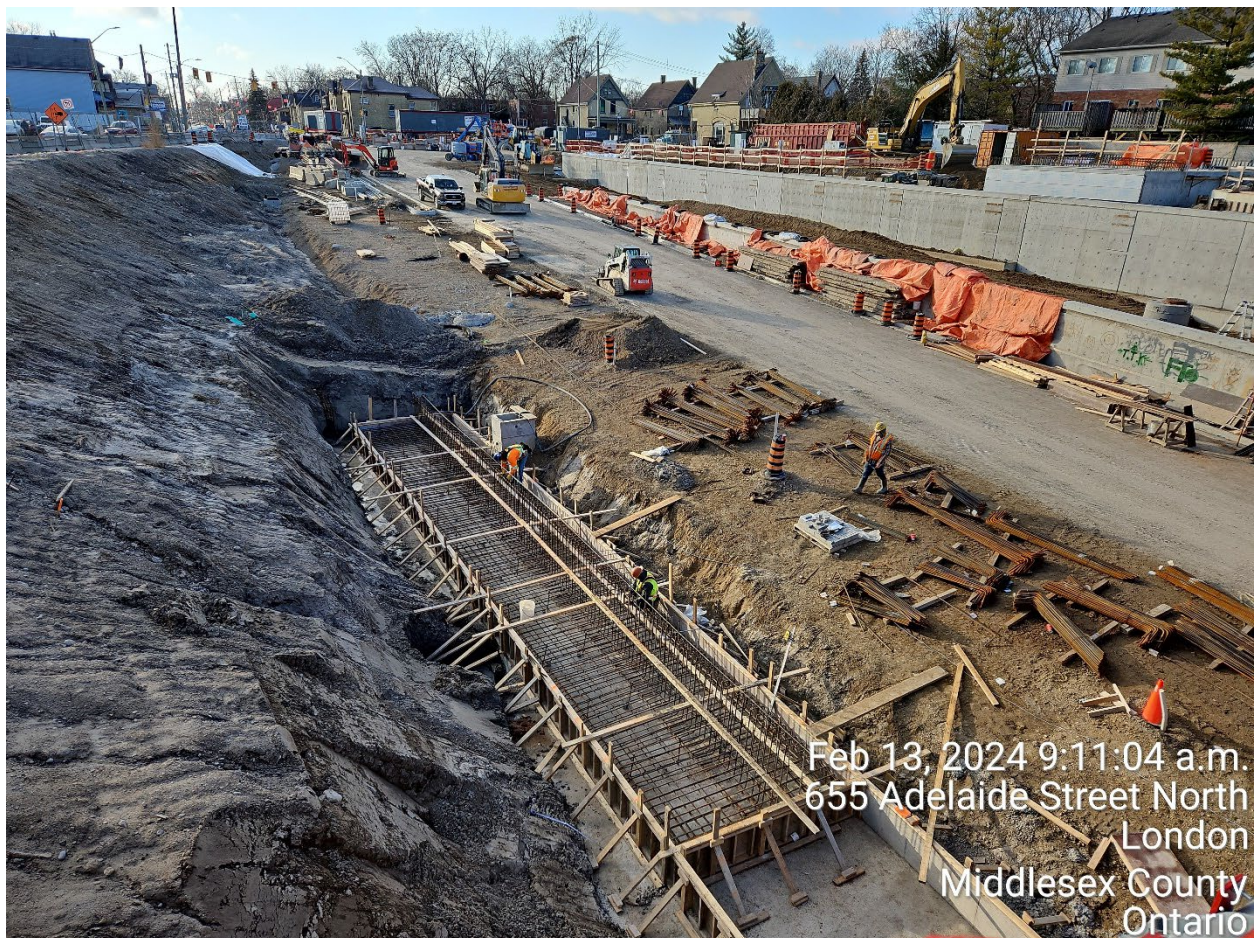
Above: Aerial view of the Adelaide Underpass construction site.
