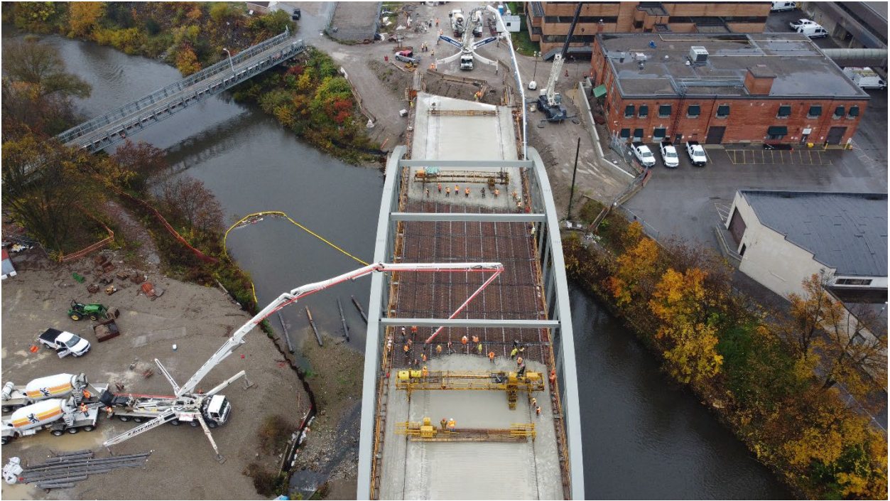
Above: An aerial view of the concrete pouring for the new bridge deck.
