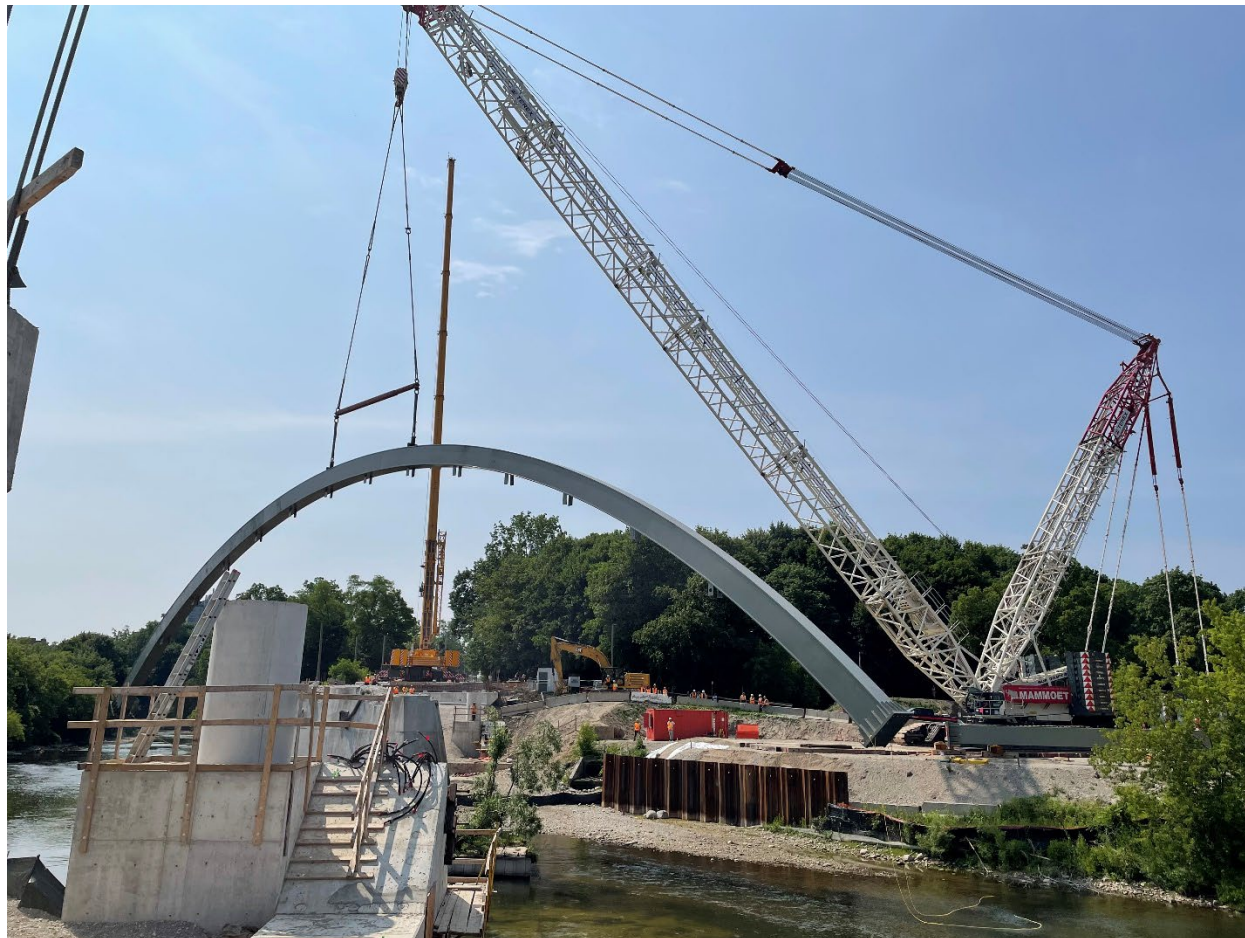
Above: Lifting operation of the new steel arches.
