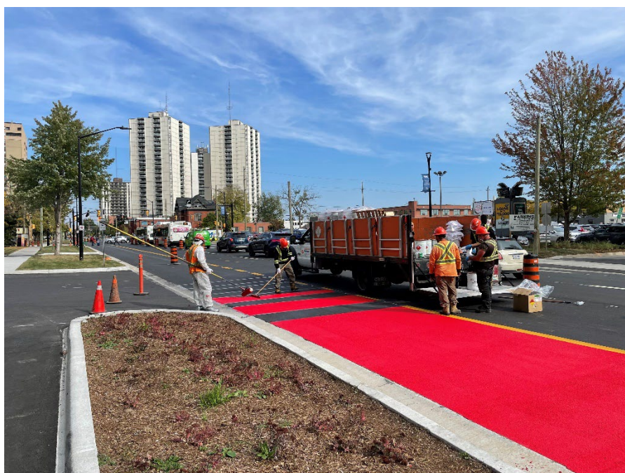
Above: Red paint operations at King Street.
