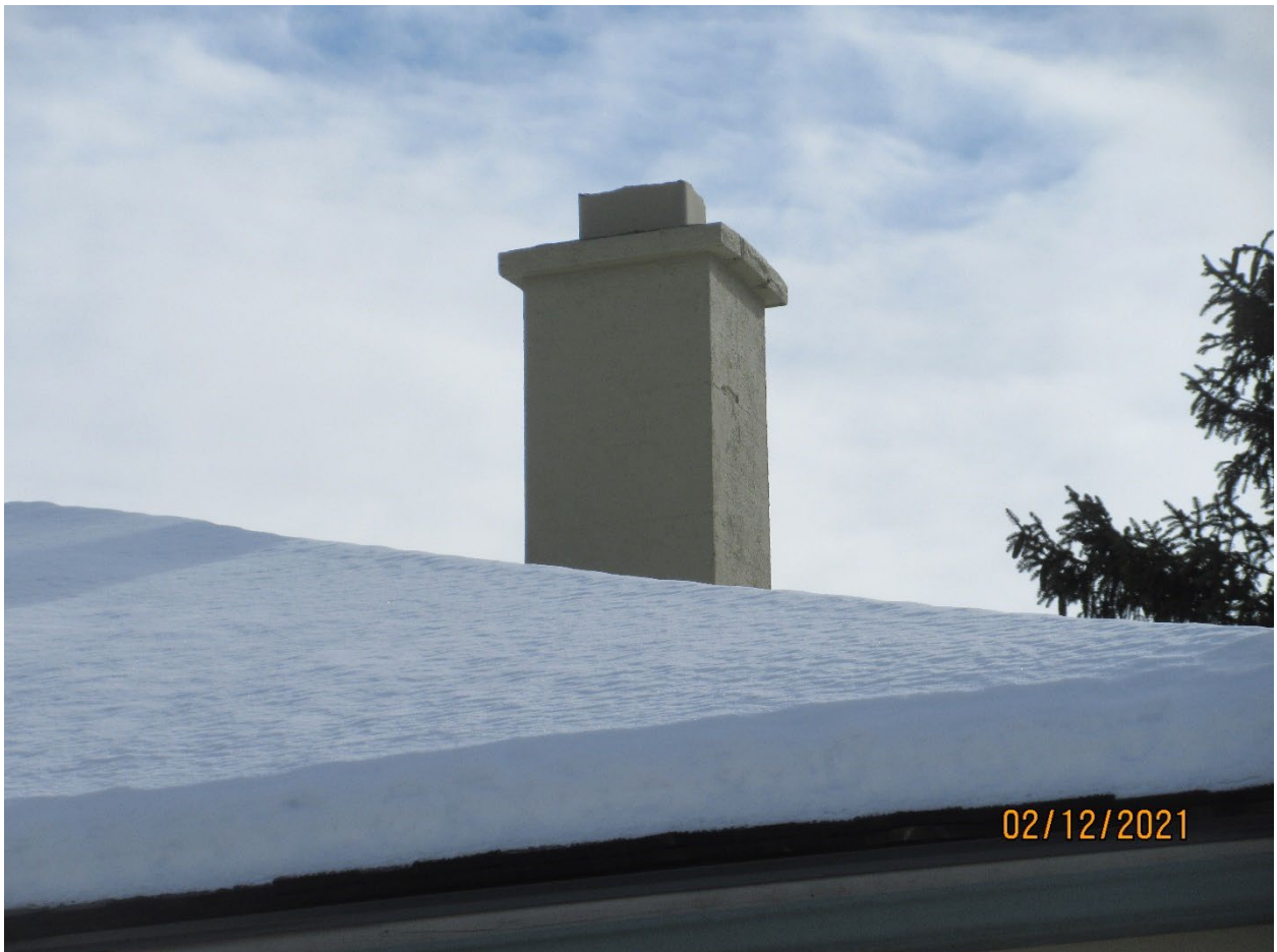
Image 10: Photograph of the west chimney, as seen from Carfrae Street (2021).
