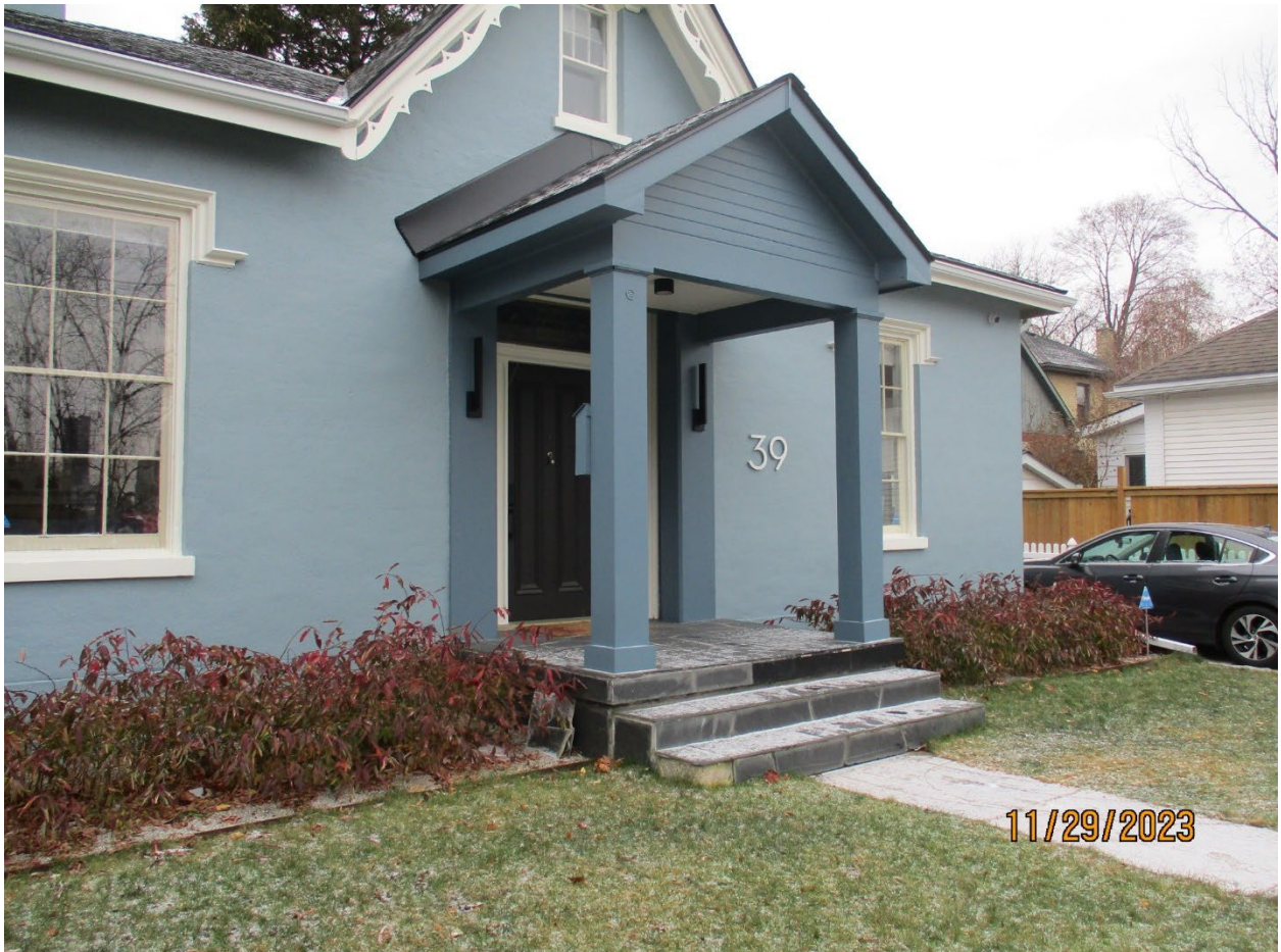
Image 20: Photograph showing the simple form of the painted wood porch over the front doorway with a shingle gable roof, supported by a plain frieze and boxed piers with simple capital and base details (2023).
