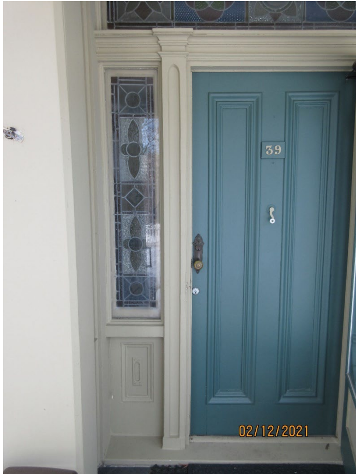
Image 15: Photograph showing the front doorway with single leaf, painted wood door with two long panels, set in a rectangular opening with rectangular sidelights to both sides, a panelled dado below, and a rectangular transom. The sidelights and transom feature reconstructed leaded and stained glass in repetitive geometric patterns with coloured and textured glass. The doorway is recessed in the façade with a plain reveal. The door opening is framed by pilasters, with entablature supporting the architectural framework of the doorway (2021).
