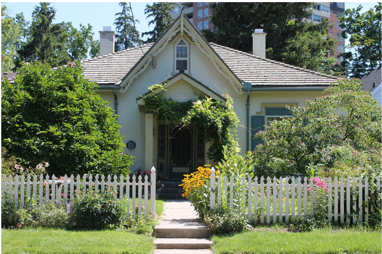
Image 2: Photograph of Carfrae Cottage on July 21, 2015.
