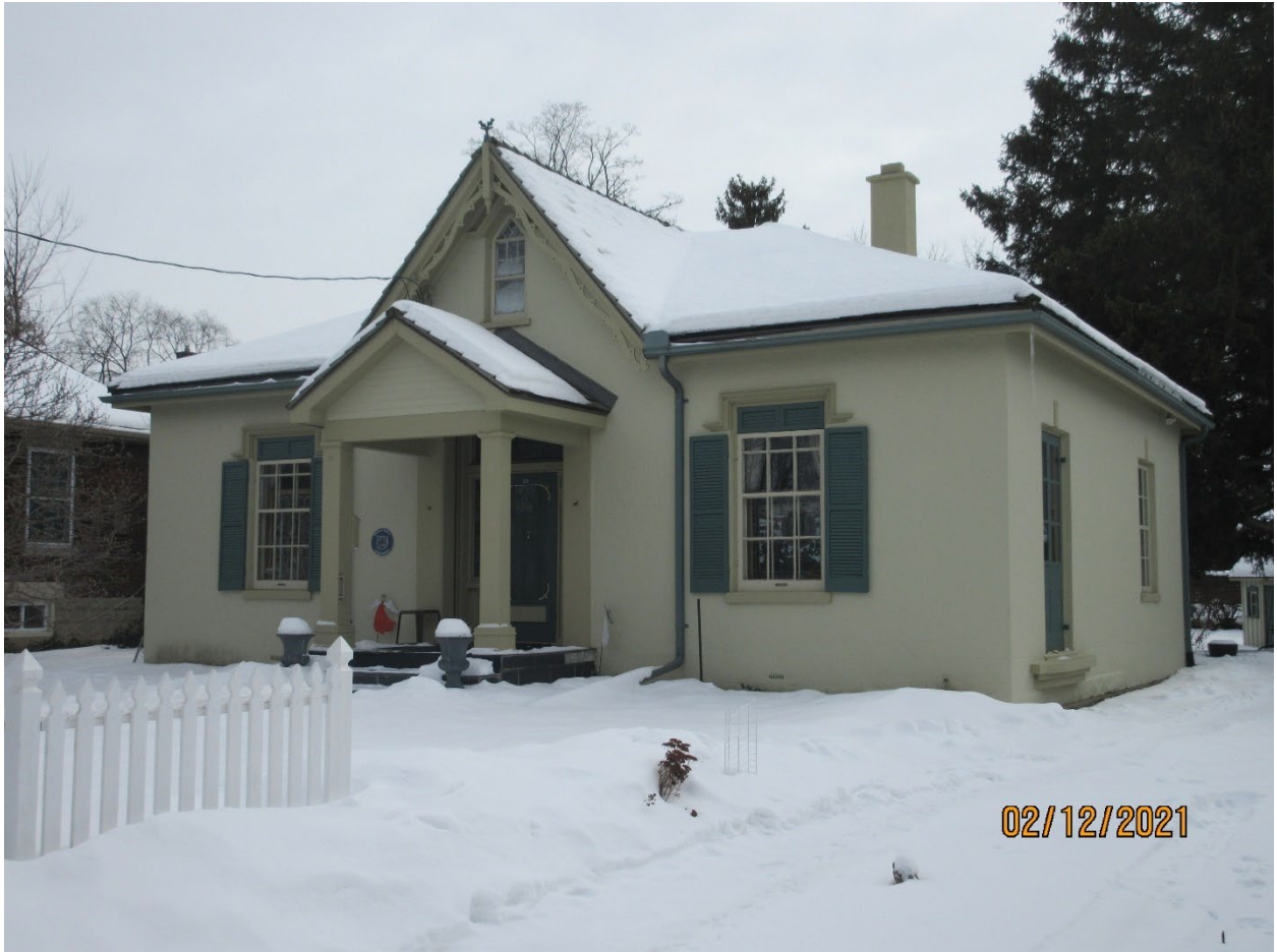
Image 5: View of Carfrae Cottage, looking southeast from the northwest corner of the property at 39 Carfrae Street (2021).
