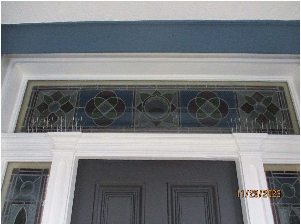
Image 18: Detail photograph showing the entablature of the doorway with pilaster, as well as a detail of the stained glass transom (2023).
