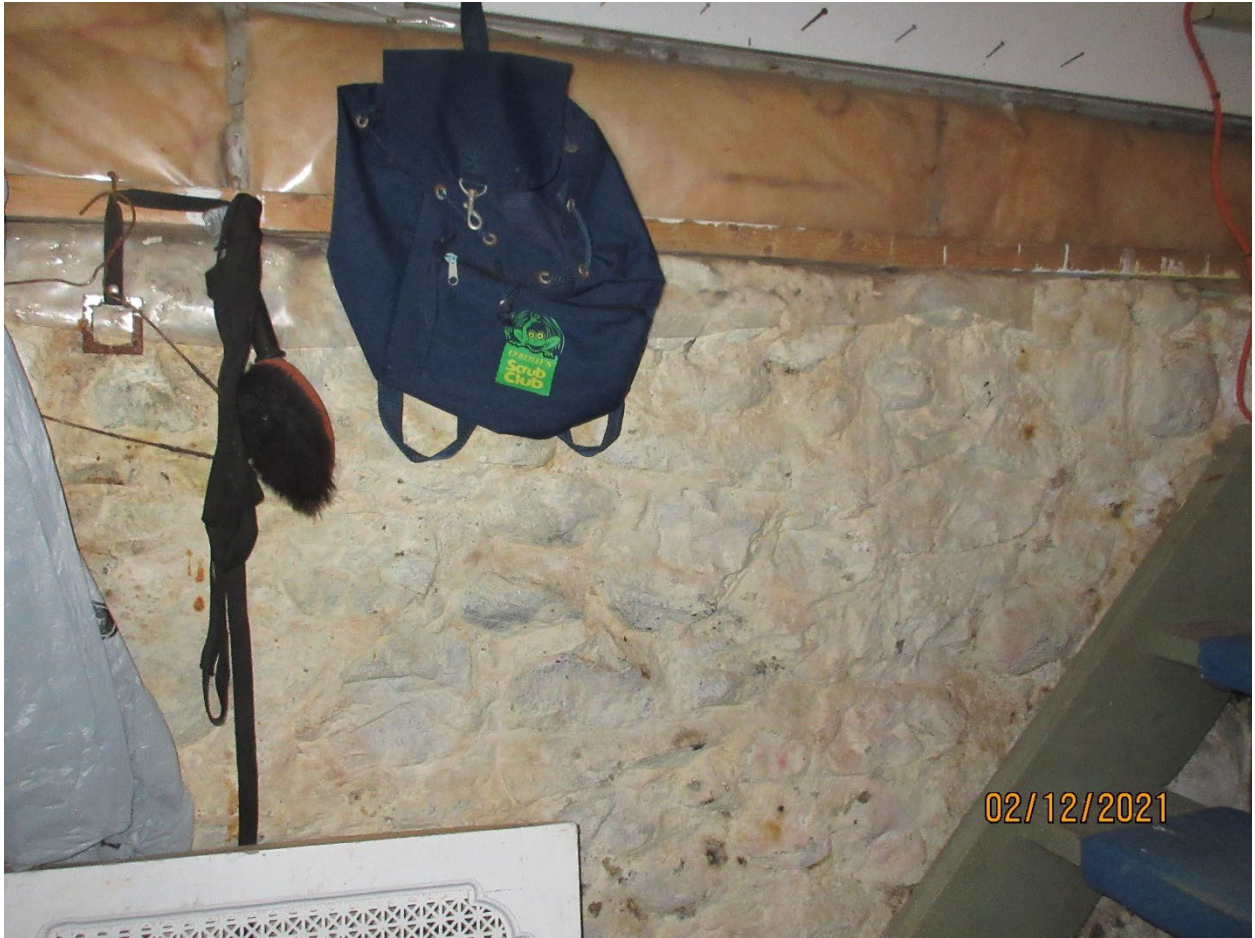
Image 9: Photograph showing an example of the rubble stone foundation construction of Carfrae Cottage, as seen in the basement (2021).
