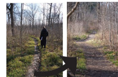
Existing Trail Water travels on the fall line down the hill Level 1 transitioning to level 2
