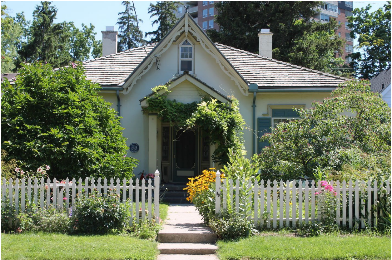
Image 2: Photograph of Carfrae Cottage on July 21, 2015.
