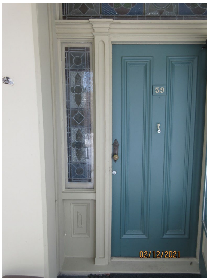
Image 15: Photograph showing the front doorway with single leaf, painted wood door with two long panels, set in a rectangular opening with rectangular sidelights to both sides, a panelled dado below, and a rectangular transom. The sidelights and transom feature reconstructed leaded and stained glass in repetitive geometric patterns with coloured and textured glass. The doorway is recessed in the façade with a plain reveal. The door opening is framed by pilasters, with entablature supporting the architectural framework of the doorway (2021).
