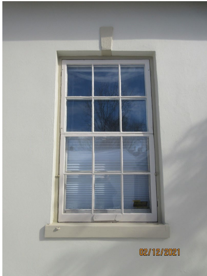
Image 30: Photograph of the painted wood six-over-six shingle hung wood window on west façade (2021).
