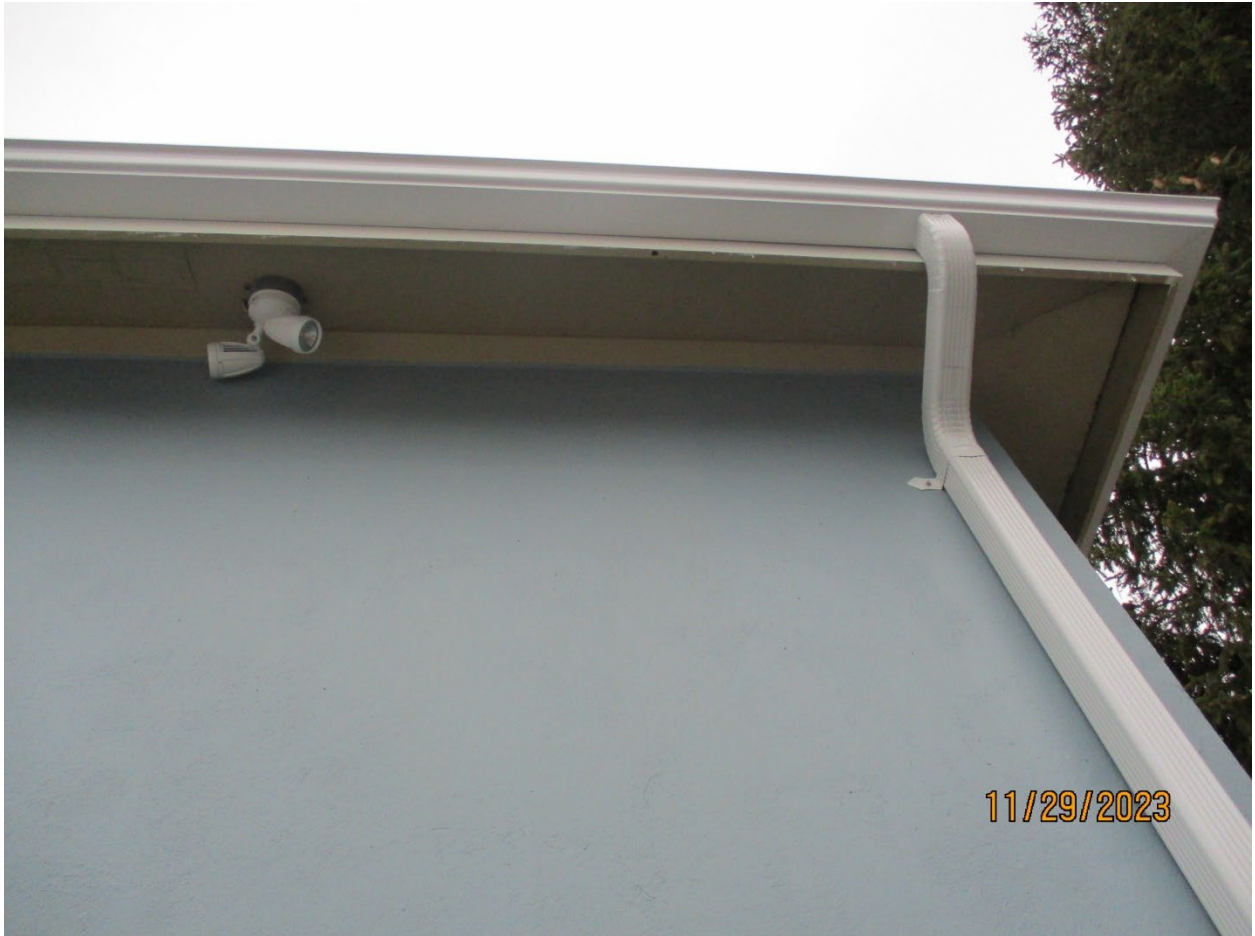
Image 13: Photograph showing the sloped soffit of the roofline (2023).
