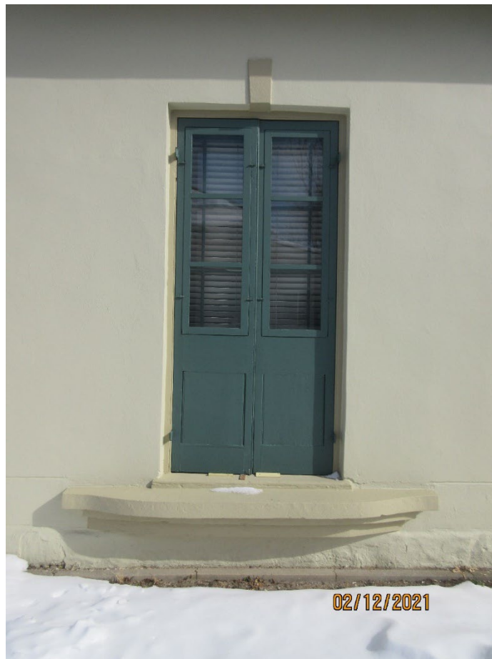
Image 28: Photograph of the painted wood French doors and painted wood storm doors in the opening of the west façade, sill as an indication of the former verandah of Carfrae Cottage (2021).
