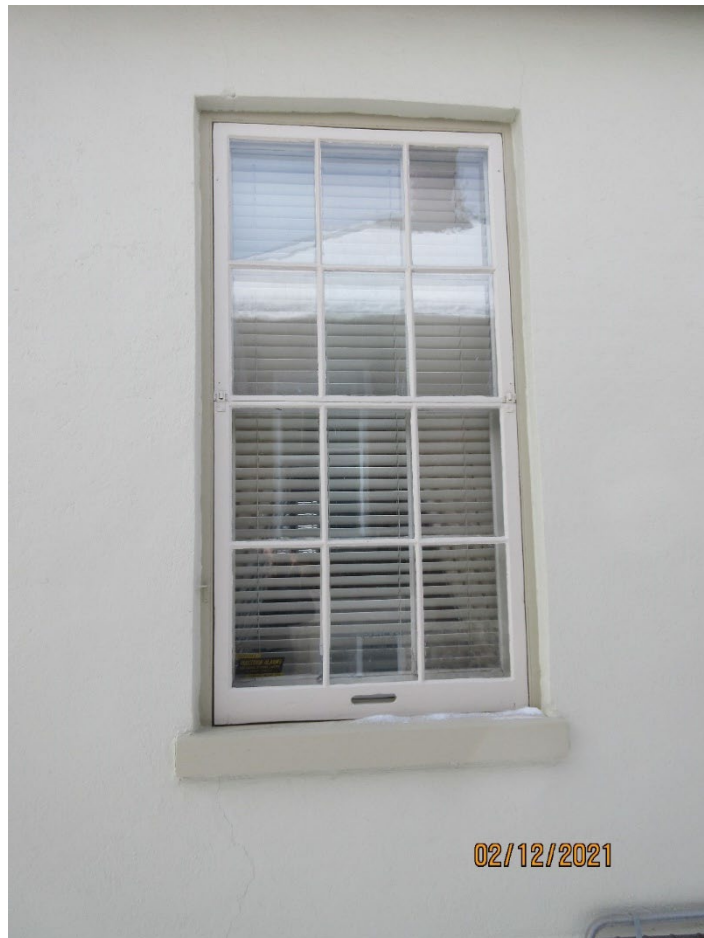
Image 34: Photograph of the six-over-six double hung painted window on east façade and wood sill on the east façade (2021).
