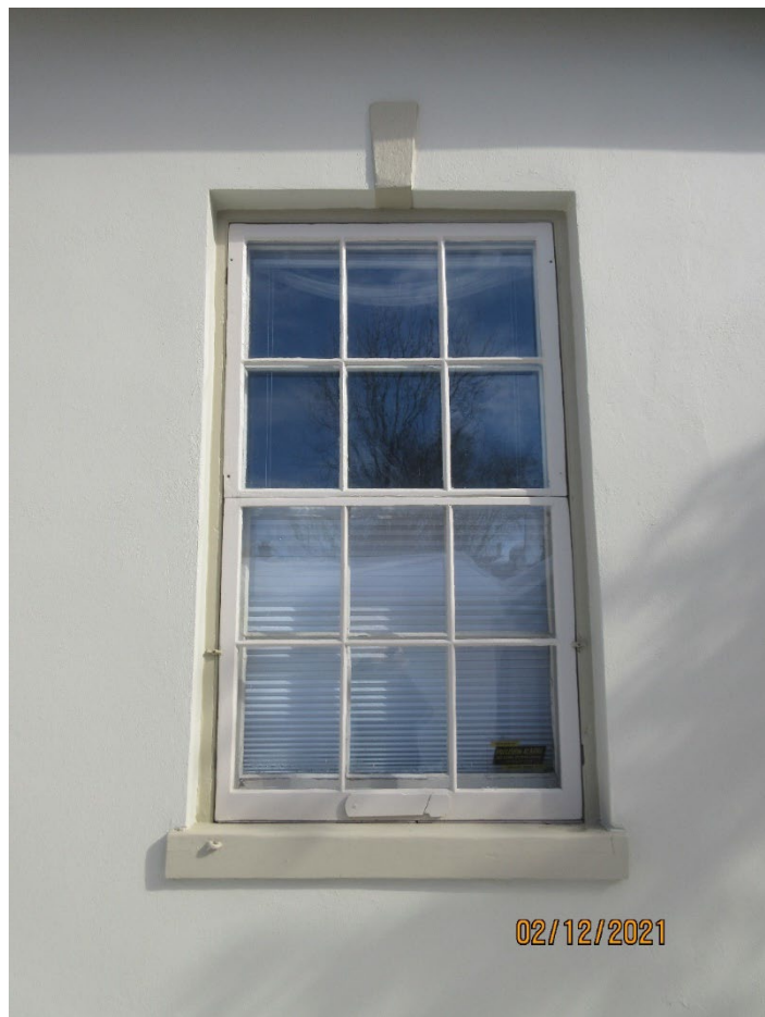
Image 30: Photograph of the painted wood six-over-six shingle hung wood window on west façade (2021).
