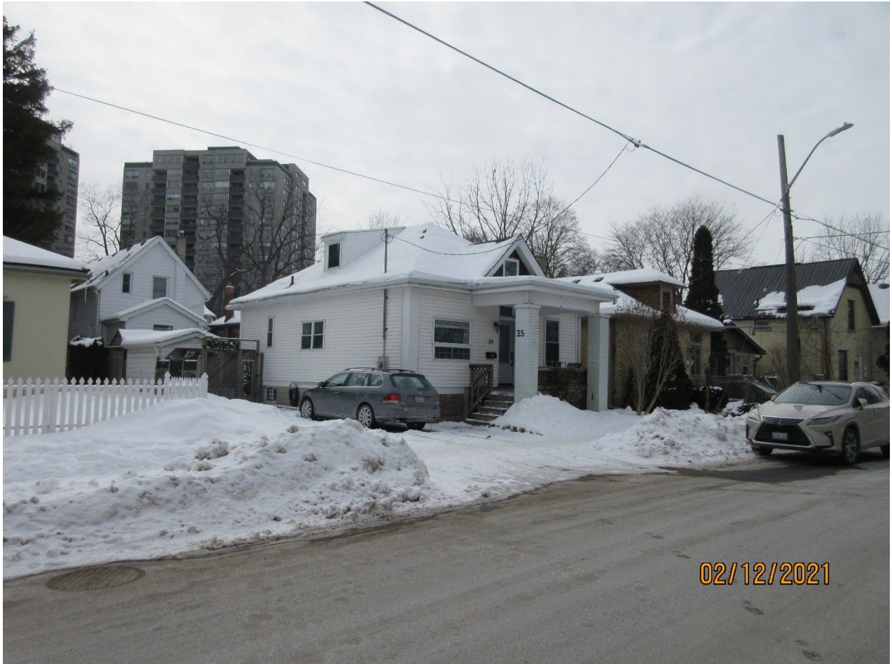
Image 8: View to the west of the property at 39 Carfrae Street, showing the property at 35 Carfrae Street (2021).
