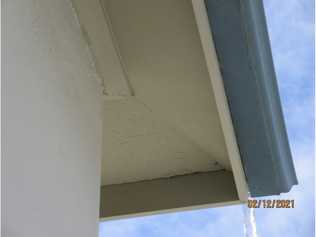
Image 12: Photograph showing the sloped soffit of the roofline (2021).
