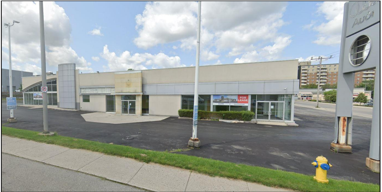
Figure 2 - Streetview of 475 Wharncliffe Road South (view looking NW)
