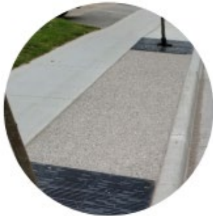
Decorative Paving Treatment
