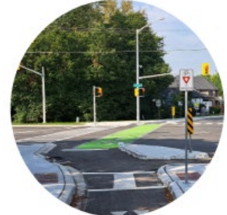
Safe Bike Lane Intersection
